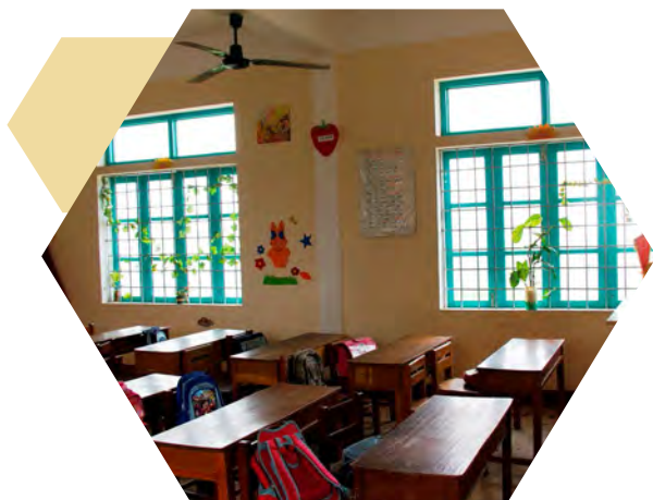
The Parents Association of the school supported the repairs to broken classroom windows represented a danger for students.
