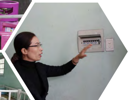
Electrical systems were renewed, according to standards.
