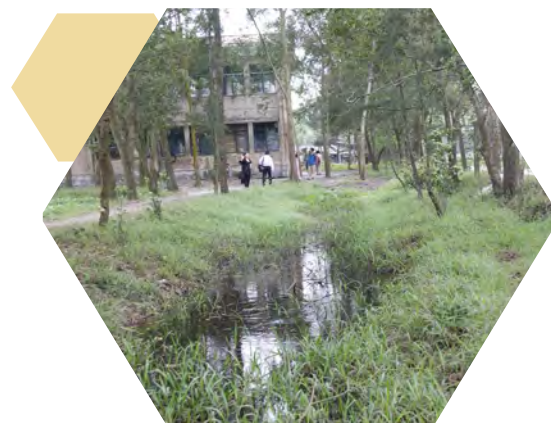
These dangerously deep holes on school grounds were identified during the application of the assessment tool as a major risk for students and school staff.
