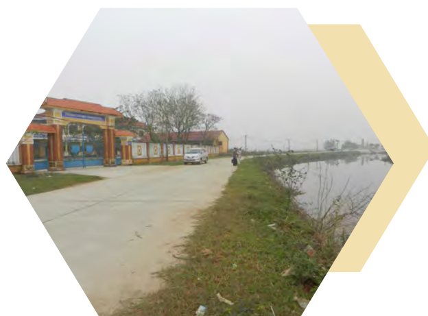
The lack of demarcation between the road and the river created a dangerous situation for students and community members during the flooding season.
