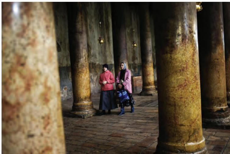
Fig. 2.15 The south aisle looking west; thirty of the nave's 44 columns carry Crusader paintings of saints and the Virgin and Child, although age and lighting conditions make them hard to see. The columns are of red, polished limestone; most have been re-used from the original 4th century Constantinian basilica
