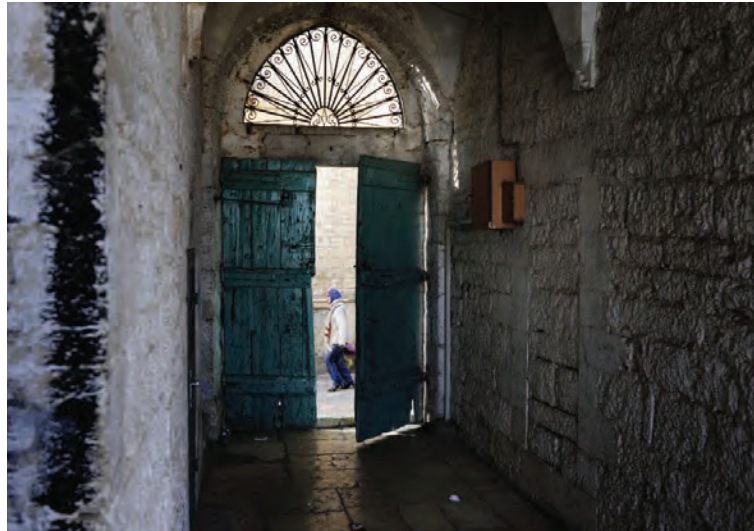
Fig. 2.27 a gate of a traditional Hosh, traditional house
