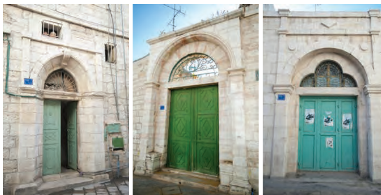
Fig 2.50 Examples of three main entrances along Star Street that, in reflecting contemporary taste c. 1900, utilise decoratively local skills in masonry and ironwork
