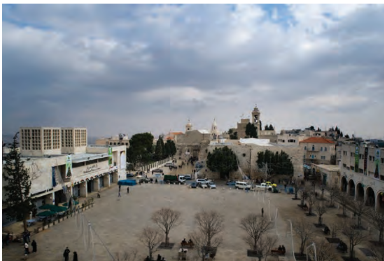
Fig. 2.1 The western elevation of the architectural ensemble of and around the Church of the Nativity, Bethlehem, viewed across Manger Square from the roof of Bethlehem Municipality
