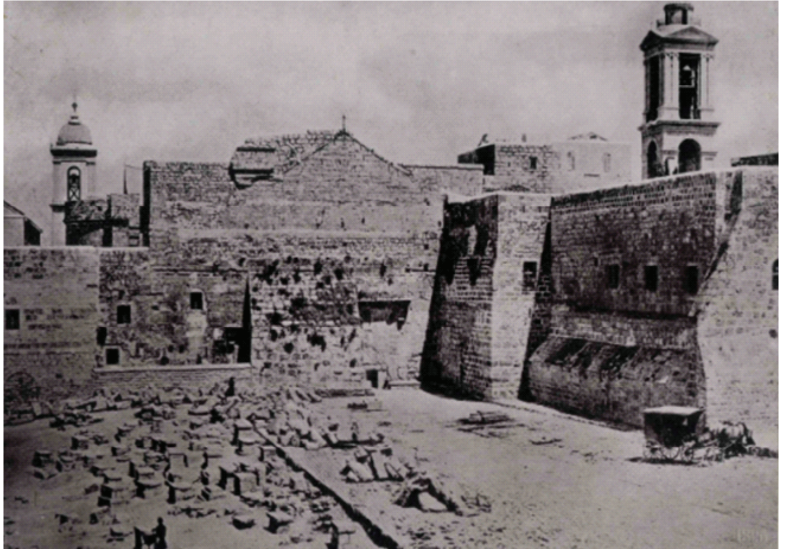
Fig. 7.10 The western elevation of the Church of the Nativity in Bethlehem in 1894, after the construction of the bell tower of the Greek Orthodox convent and the Church of St. Catherine, Photograph by Ch. Scolik, George Al Ama Collection
