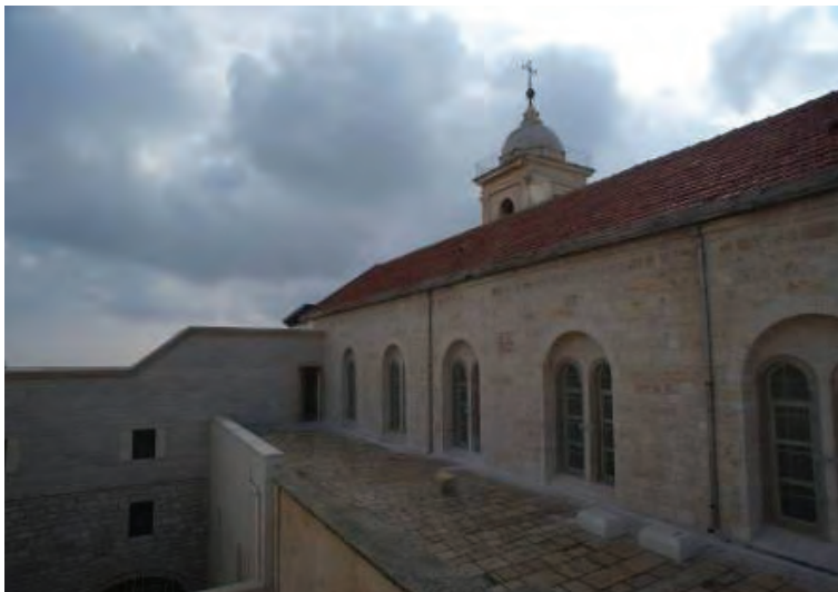
Fig. 7.46 the roof of the Basilica
