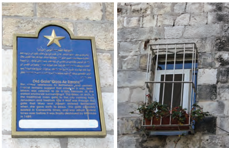
Fig. 2.49 Mamluk engraving on the window lintel on the first floor of the western elevation of Damascus Gate. The inscription on the plaque next to the Gate reads: ‘Old Gate ‘Qoos Zarara’: the oldest references to Bethlehem and archeological remains suggest that small as it was, Bethlehem was referred to as a city because of the walled enclosure surrounding it. This Qoos, or arch, is the traditional main gate to the city coming from Jerusalem and tradition has it that was through this gate that Mary and Joseph entered Bethlehem when she gave birth to Jesus. The wall probably existed in Canaanite times, and was rebuilt several times over before it was finally destroyed by Mamluks in 1489.’
