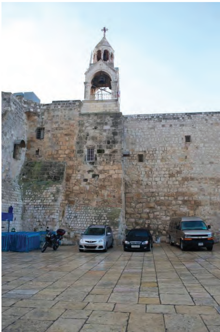
Fig 7.38 the forecourt in front of the Church looking at the Armenian Convent walls and bell-tower
