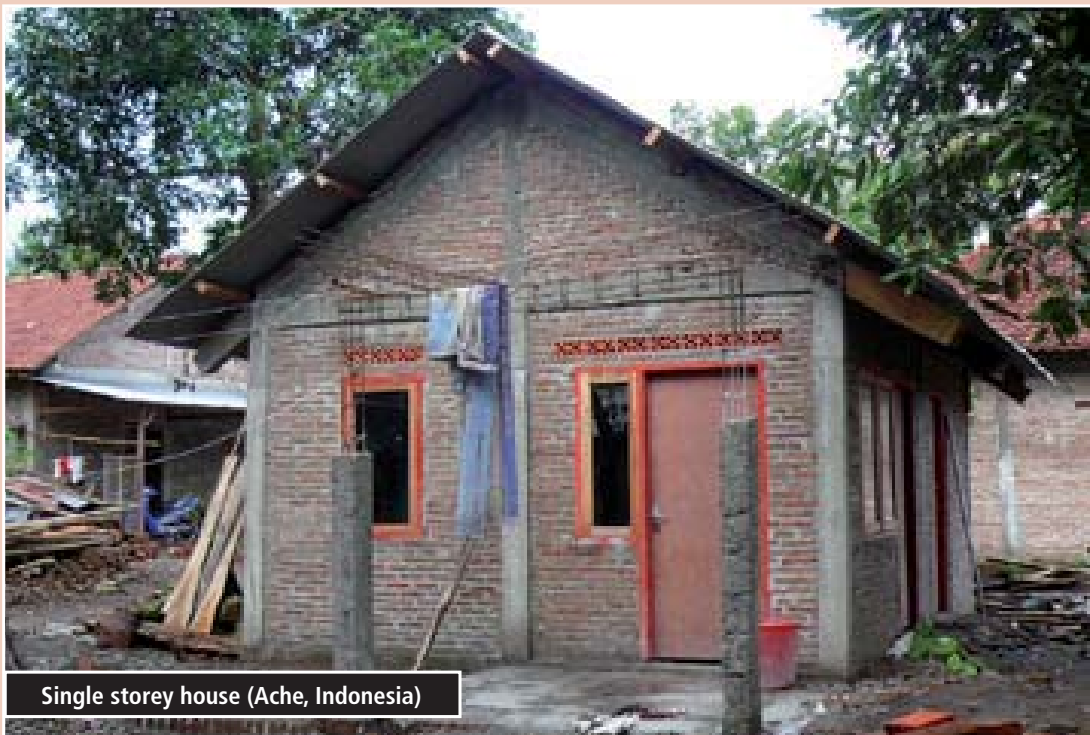
Figure 4.18: Confined brick masonry
