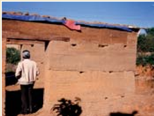
a) Tapial house under construction house
