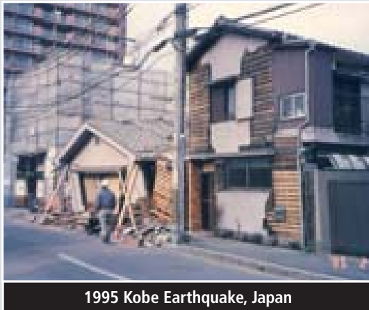
Figure 6.5: Damage to wooden houses
