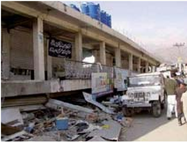
Figure 8.2: Collapsed RC building (2005 Northern Pakistan Earthquake)
