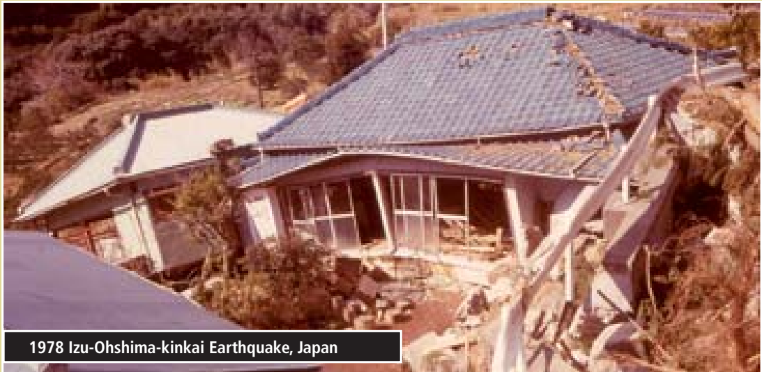
Figure 2.2: Damage caused by ground failure
