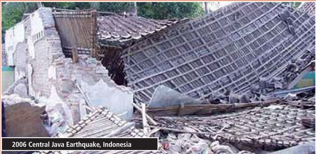
Figure 4.4: Damage brick masonry
