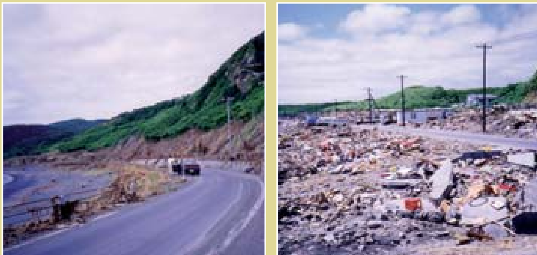
1993 Hokkaido-nansei-oki Earthquake, Japan (Tsunami run-up height reached 15 m average and 31 m max. and all houses were swept away.)
