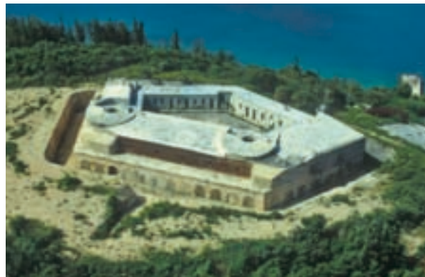
Fort Cunningham was rebuilt in the 1870s with two wrought iron gun facades; the larger for five guns appears in the foreground.
