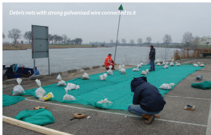
Usually we have to tailor our methodologies to protect sites underwater. We can, however, base our solutions on methods tried somewhere else. Here, a Roman quay in the River Meuse in the Netherlands is being protected with a layer of geotextile (above, left) followed by a layer of clay (above), debris nets with strong galvanised wire connected to it (left) and sandbags. © RCE
