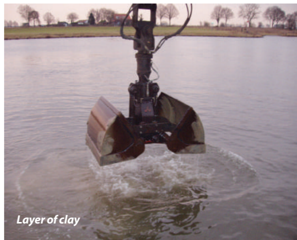
Usually we have to tailor our methodologies to protect sites underwater. We can, however, base our solutions on methods tried somewhere else. Here, a Roman quay in the River Meuse in the Netherlands is being protected with a layer of geotextile (above, left) followed by a layer of clay (above), debris nets with strong galvanised wire connected to it (left) and sandbags. © RCE
