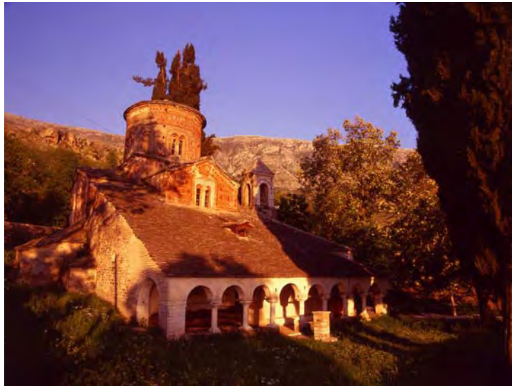
Fig. 5 – The church at Labove
