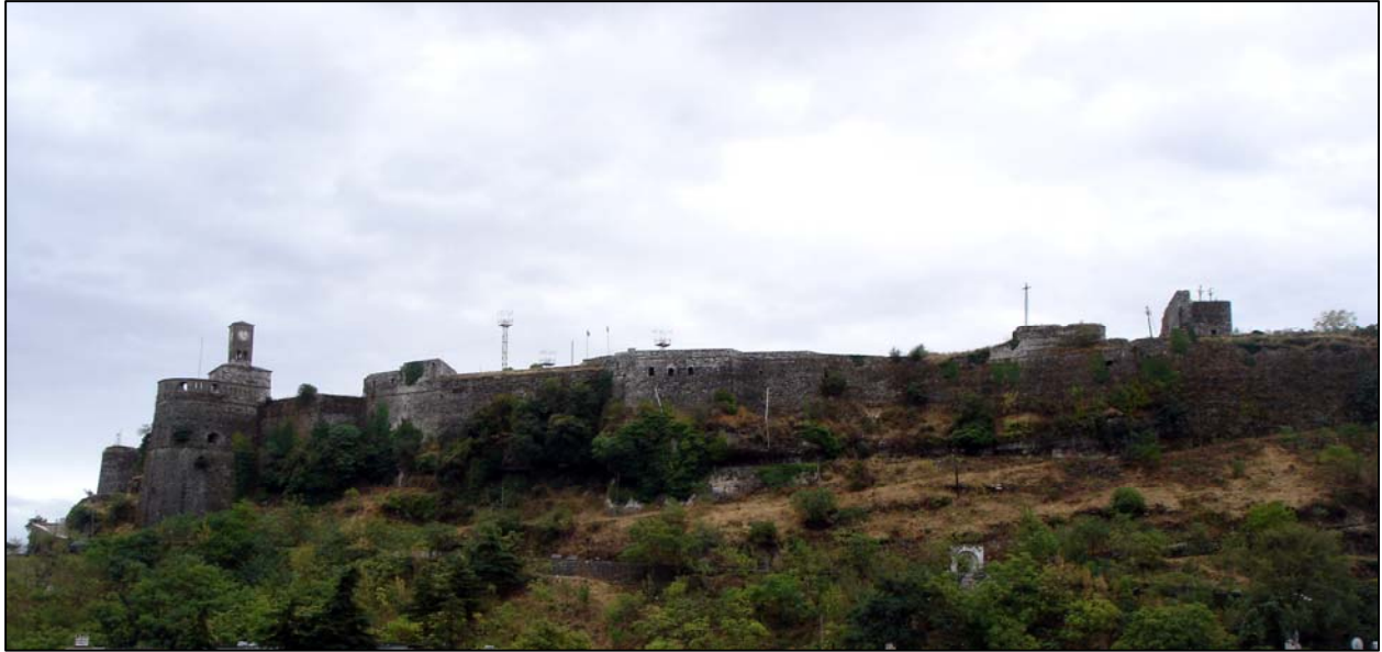
GENERAL VIEW OF THE WESTERN SIDE OF THE CASTLE
