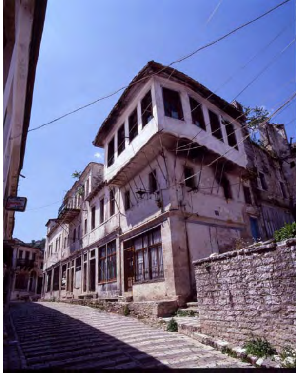
Fig. 11 – An almost deserted street in the bazaar
