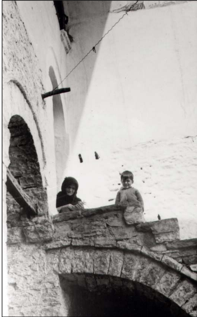
VIEW OF LOOP-HOLES IN THE WALL THE HOUSE OF SKENDULI
