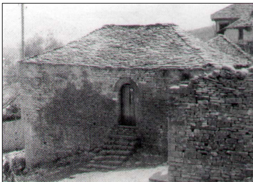
VIEW OF THE WATER BUTT
