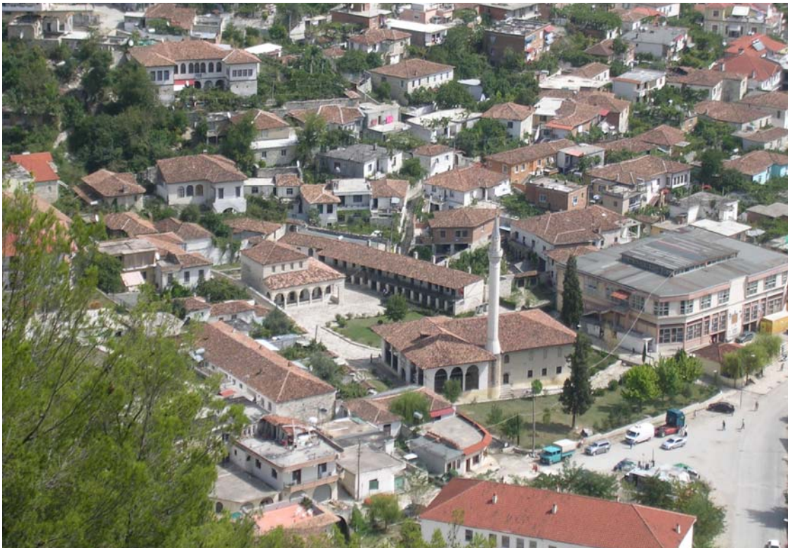
The Medieval Centre and the buildings of the Buffer Zone.
