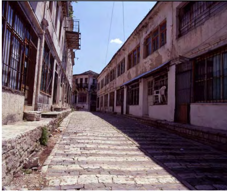
Fig. 32 – Bazaar street, much of which is abandoned and derelict
