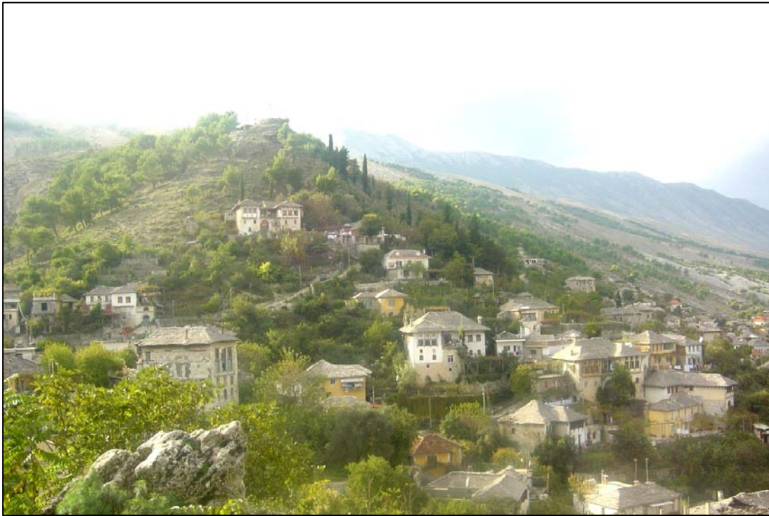
GENERAL VIEW OF "TEQE" QUARTER
