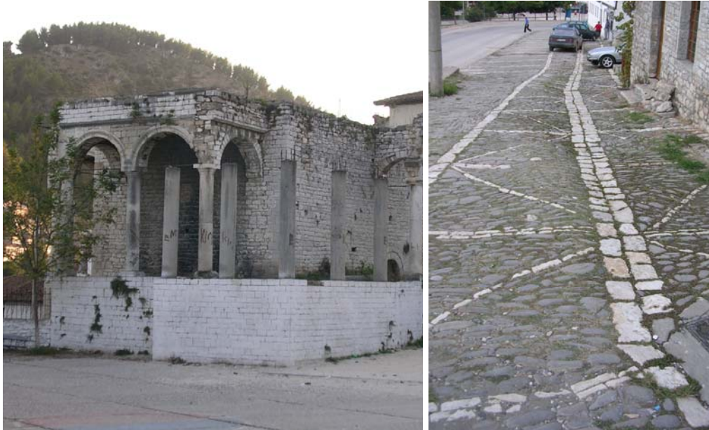
Turkish Villa in Area 1, that has to be subject of Detailed Recovery Plan (left) and Historical paving of ancient streets to be restored (right).
