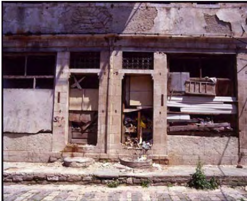
Fig. 12 – A rubbish-filled building in the bazaar
