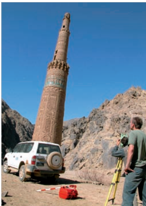
Fig. 7 a and b | Comparative monitoring on the inclination of the Minaret (2006 and 2002). TOP: © UNESCO/T. STEVENS NEXT: © UNESCO/M. SANTANA
