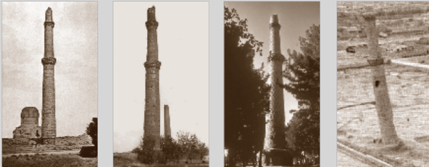
Fig.1 | The Fifth Minaret in Herat (from left to right; 1915, 1933, 1975 and 1993). The position of the photographer is different in each shot, but the general trend of inclination is clear.
