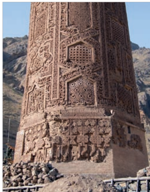
Fig. 19 | The Minaret of Jam during strengthening work (2006).
