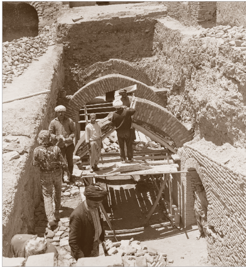
Fig. 9 | Afghan workers rebuilding the collapsed vaults of a building in the Herat Citadel (1978-79).
