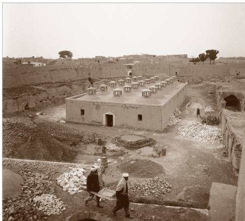
Fig. 7 | Military Museum before restoration work, Herat Citadel (1975). PHOTO: © A. BRUNO
