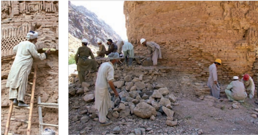
Fig. 17 and 18 | Afghan workers during strengthening work on the Minaret of Jam (2006).
