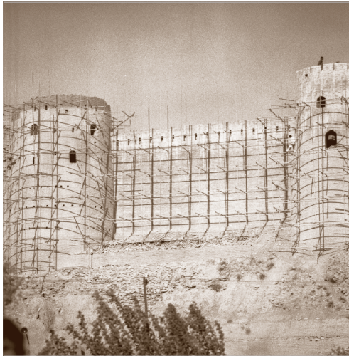
Fig.11 | Citadel ramparts during restoration work (1978-79). PHOTO: ©A. BRUNO
