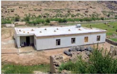
Fig. 3 | Project house in the Jam site (2003). PHOTO: © UNESCO/F. LANGLOIS
