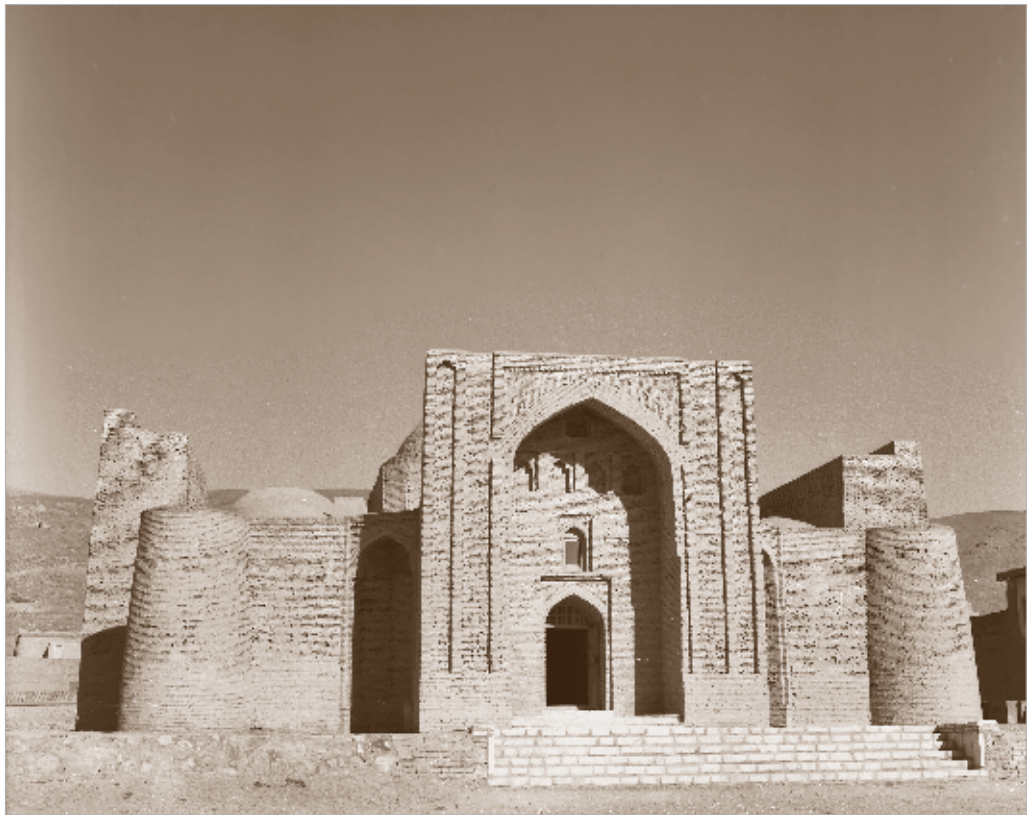
Fig. 6 | Rawza (1966): the 'Abd al-Razzaq Mausoleum after restoration. PHOTO: © ISIAO
