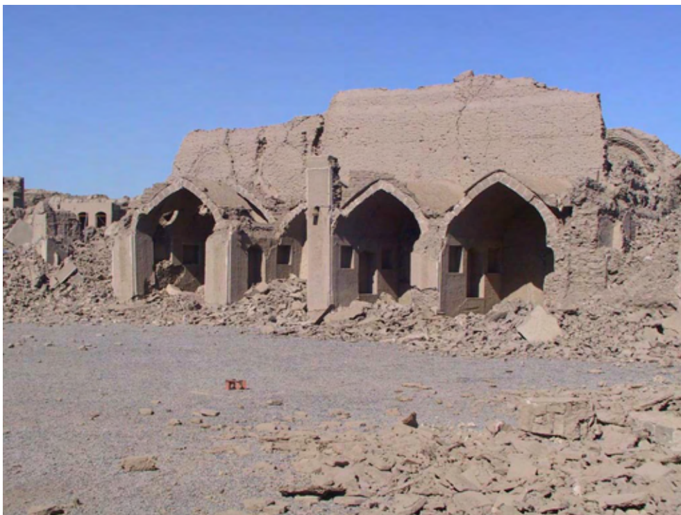
Fig. 29. Tekiyeh before and after earthquake
