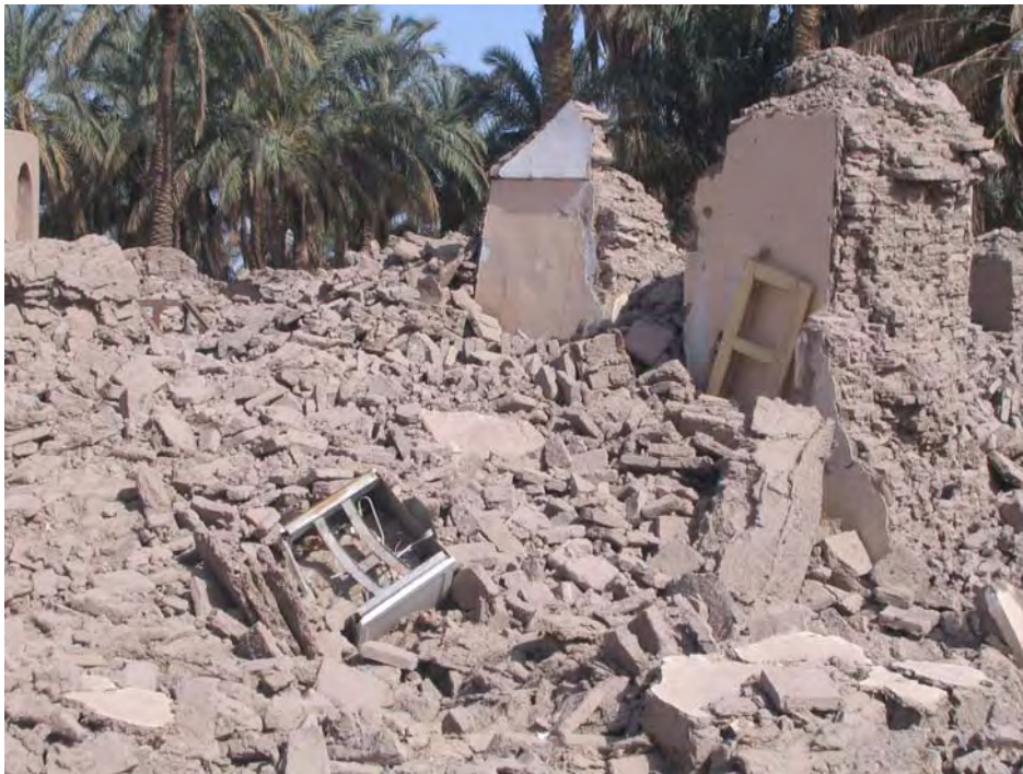
Fig.50. Ahmadiyah School before and after the earthquake
