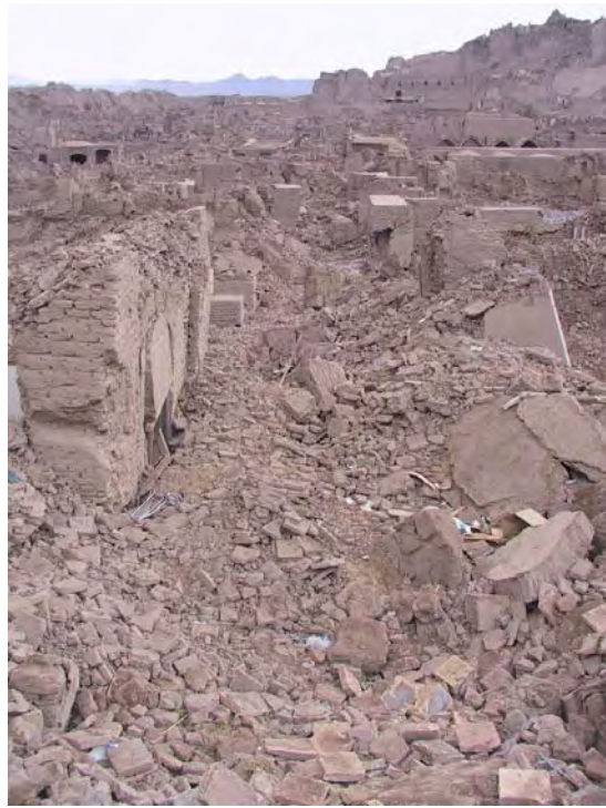
Fig. 31. Bazaar before and after the earthquake
