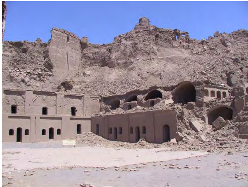
Fig. 19. Garrison before and after earthquake
