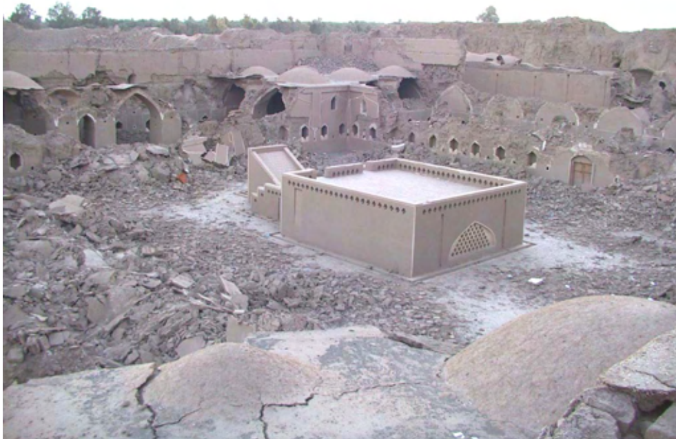
Fig. 20. The Stables before and after earthquake.
