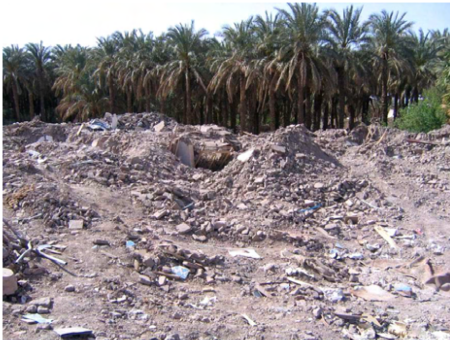
Fig.60. Mehdizadeh House before and after the earthquake
