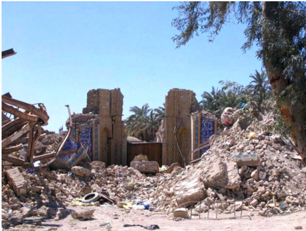
Fig.44. Vakil Mosque before and after the earthquake
