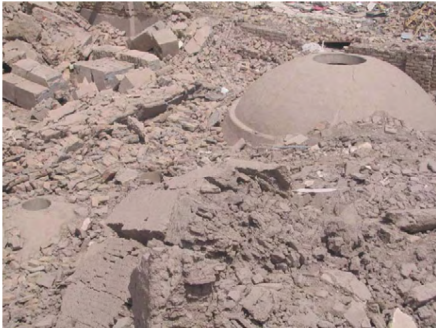
Fig.42. Vakil Bath after and before the earthquake
