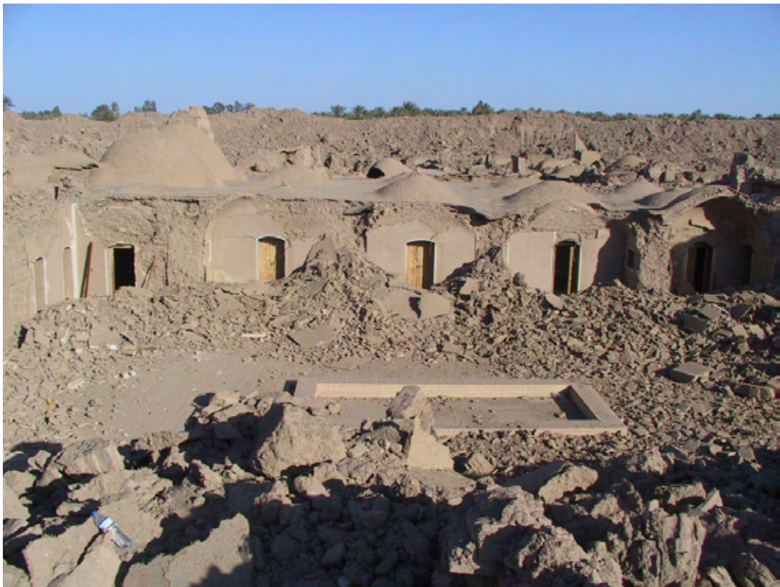
Fig. 22. Mirza Na'im School before and after earthquake.
