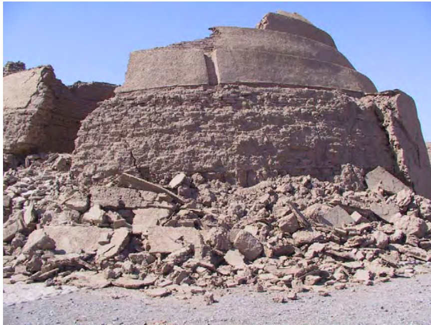
Fig.13. Yakhdan before and after earthquake
