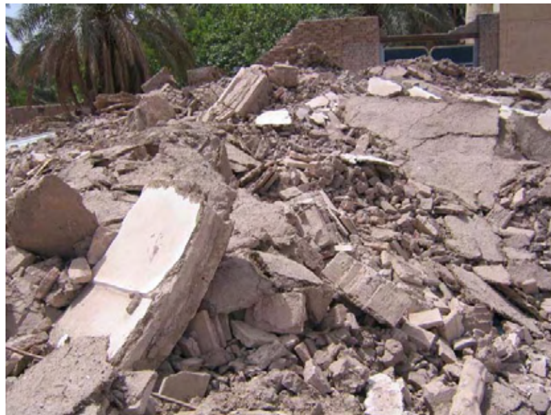
Fig.54. Views from the Emad School before and after the earthquake
