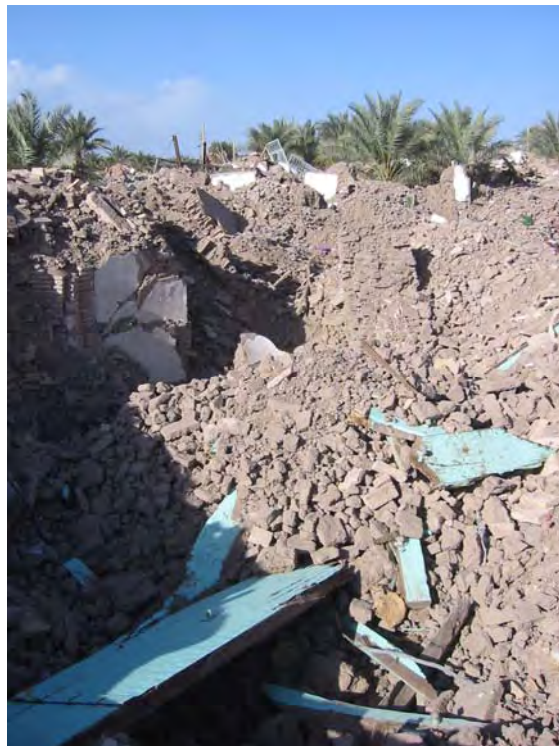
Fig.48. Ansari House after the earthquake
