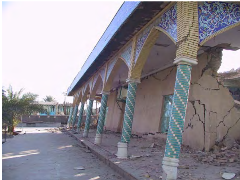
Fig.58. Emāmzādeh Asiri Mausoleum after the earthquake
