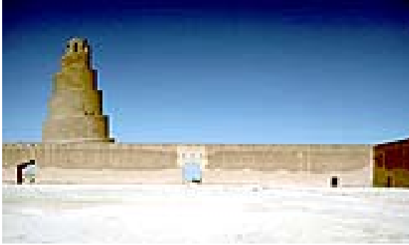
(Figure # 12) The Great Mosque and its Spiral Minaret inside.
