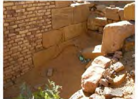
DSCN3838.JPG, Structural Deterioration of Pyramids, Water Damage, Southern Cemetery
