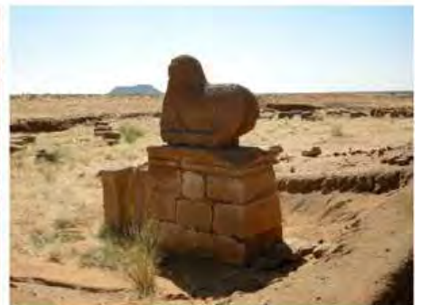
DSCN4124.JPG, Naqaa, Amun Temple, Exposure and Deterioration of Ancient Plasters, Inappropriate/Inexistent Site Drainage, Deterioration of Ancient Mud Structures
