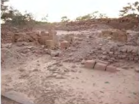
DSCN3968.JPG, Structural Instability of Walls/Collapse of Archaeological Features, Inappropriate Dumping of Excavation Spoils, Inappropriate/Inexistent Site Drainage, Royal City
