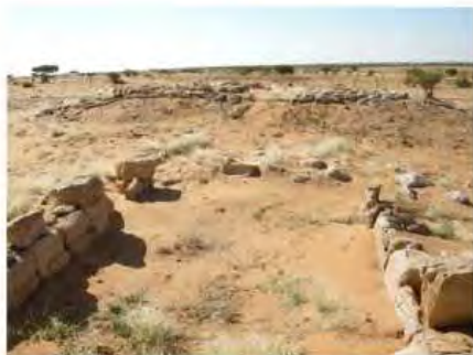
DSCN4061.JPG, Naqaa, Temple B200, Structural Instability of Walls/Collapse of Archaeological Features, Degradation of Stone/Masonry Elements
