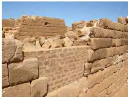
DSCN4180.JPG, Musawwarat - Great Enclosure, Restoration Works
