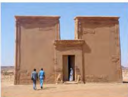
DSC06216.JPG, Musawwarat - Re-erected Lion Temple, Restoration Works
