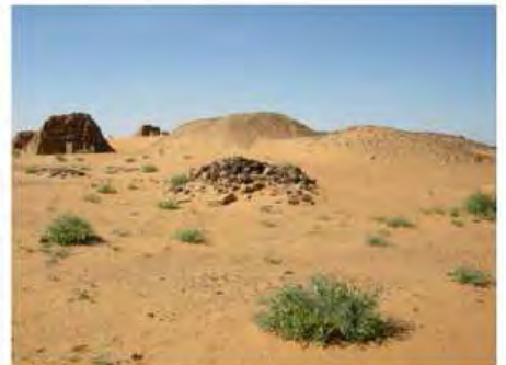
DSCN3826.JPG, Structural Deterioration of Pyramids, Southern Cemetery
