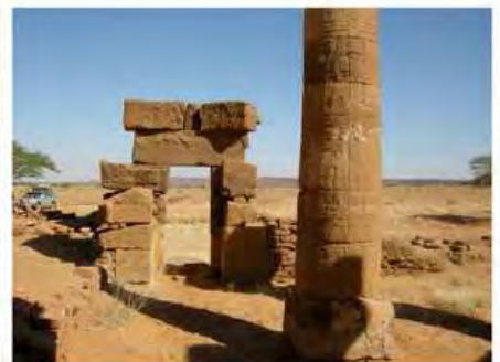
DSCN4099.JPG, Naqaa, Amun Temple, Degradation of Stone/Masonry Elements, Exposure and Deterioration of Ancient Plasters
