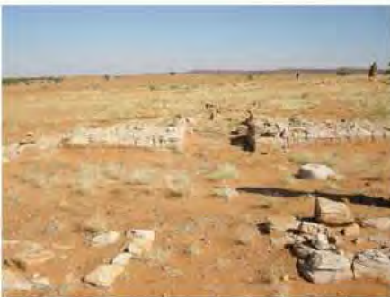
DSCN4066.JPG, Naqaa, Temple B200, Degradation of Stone/ Masonry Elements
