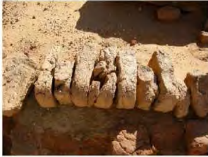
DSCN4090.JPG, Naqaa, Amun Temple, Degradation of Stone/Masonry Elements, Structural Instability of Walls/Collapse of Archaeological Features
