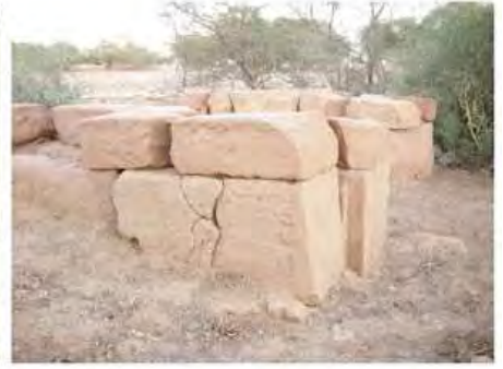
DSCN3931.JPG, Structural Instability of Walls/Collapse of Archaeological Features, Degradation of Stone/Masonry Elements, Inappropriate/Inexistent Site Drainage, Vegetation Damage, Royal City
