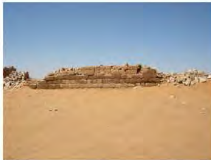
DSCN4168.JPG, Musawwarat - Great Enclosure, Degradation of Stone/Masonry Elements, Structural Instability of Walls/Collapse of Archaeological Features, Salt Crystallization
