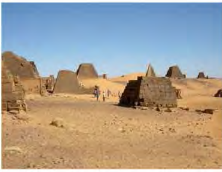
DSCN3756.JPG, Structural Deterioration of Pyramids, Northern Cemetery
