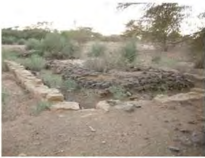
DSCN3941.JPG, Vegetation Damage, Structural Instability of Walls/Collapse of Archaeological Features, Royal City
