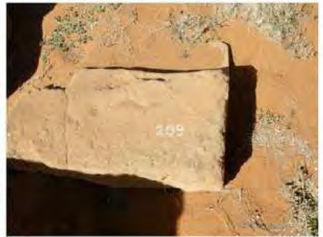
DSCN4116.JPG, Naqaa, Amun Temple, Inappropriate/Inexistent Site Drainage
