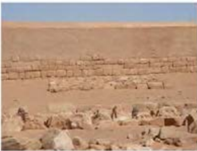
DSC06179.JPG, Musawwarat - Great Enclosure, Restoration Works
