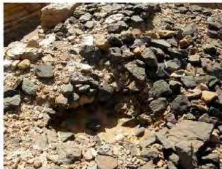
DSCN3730.JPG, Structural Deterioration of Pyramids, Northern Cemetery
