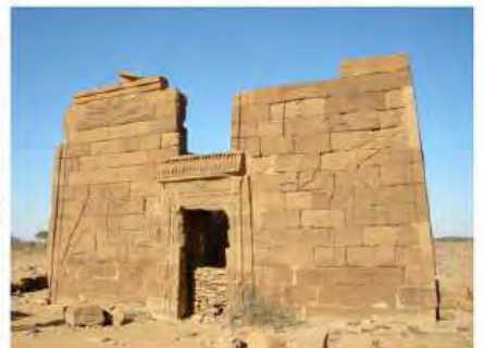
DSCN4019.JPG, Lion Temple B300 - Naqaa, Naqaa, Inappropriate/ Inexistent Site Drainage
