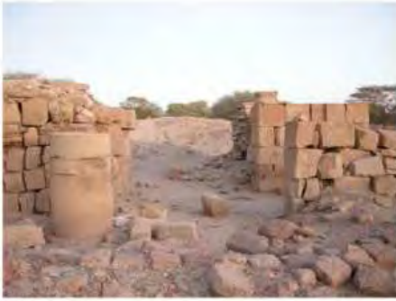
DSCN3989.JPG, Structural Instability of Walls/Collapse of Archaeological Features, Royal City
