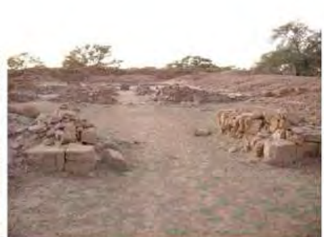
DSCN3964.JPG, Structural Instability of Walls/Collapse of Archaeological Features, Degradation of Stone/Masonry Elements, Inappropriate/Inexistent Site Drainage, Inappropriate Dumping of Excavation Spoils, Royal City
