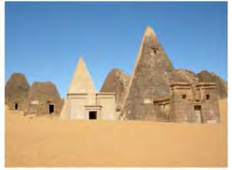
DSCN3782.JPG, Site Wide View, Salt Crystallization, Northern Cemetery
