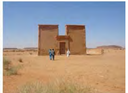
DSC06215.JPG, Musawwarat - Re-erected Lion Temple, Restoration Works
