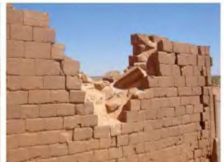
DSC06209.JPG, Musawwarat - Great Enclosure, Restoration Works
