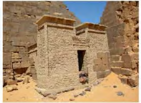
DSCN3800.JPG, Henkel Restoration, Southern Cemetery
