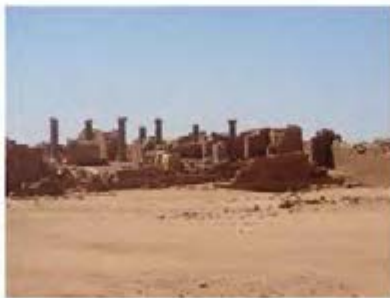
DSC06183.JPG, Musawwarat - Great Enclosure, Structural Instability of Walls/Collapse of Archaeological Features, Structural Instability of Walls/Collapse of Archaeological Features
