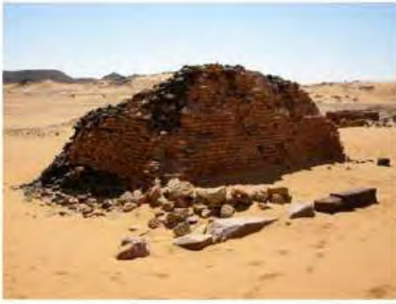
DSCN3780.JPG, Structural Deterioration of Pyramids, Northern Cemetery
