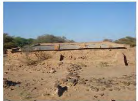
DSC06264.JPG, Redundant/Inappropriate Visitor Infrastructure, Royal City
