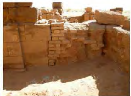
DSCN4107.JPG, Naqaa, Amun Temple, Deterioration of Ancient Mud Structures
