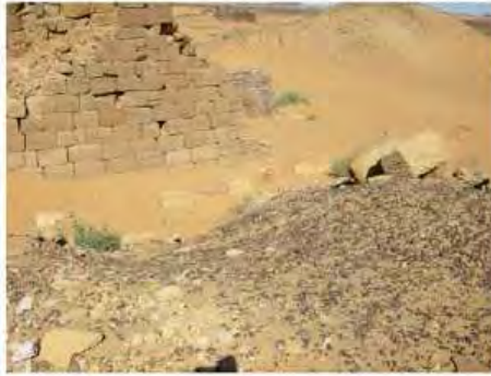
DSCN3846.JPG, Structural Deterioration of Pyramids, Southern Cemetery
