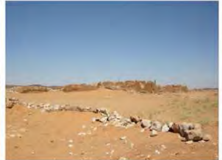
DSCN4166.JPG, Musawwarat - Great Enclosure, Structural Instability of Walls/Collapse of Archaeological Features
