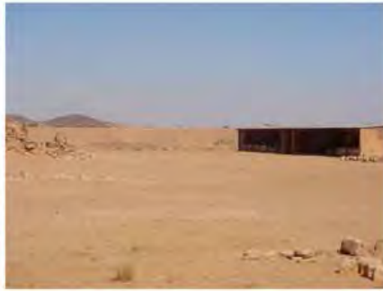
DSC06196.JPG, Musawwarat - Great Enclosure, Restoration Works
