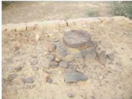
DSCN3936.JPG, Degradation of Stone/Masonry Elements, Structural Instability of Walls/Collapse of Archaeological Features, Royal City
