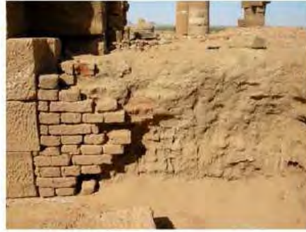
DSCN4110.JPG, Naqaa, Amun Temple, Deterioration of Ancient Mud Structures
