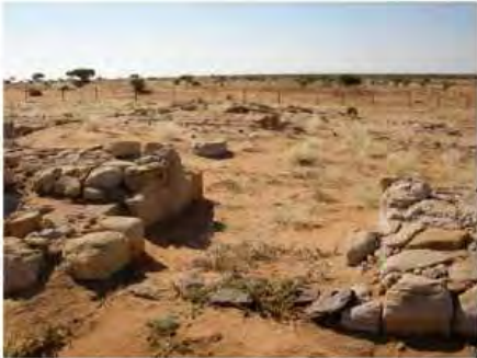
DSCN4062.JPG, Naqaa, Temple B200, Degradation of Stone/Masonry Elements, Structural Instability of Walls/Collapse of Archaeological Features, Vegetation Damage
