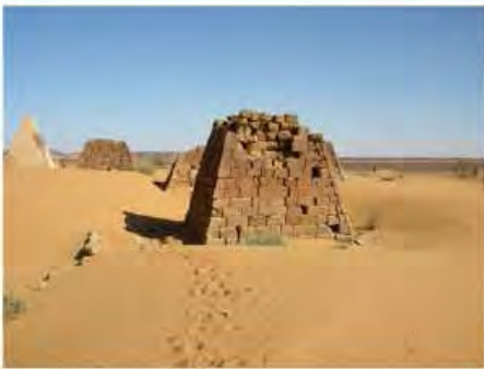
DSCN3864.JPG, Structural Deterioration of Pyramids, Southern Cemetery
