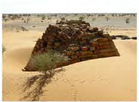
DSCN3853.JPG, Structural Deterioration of Pyramid, Southern Cemetery
