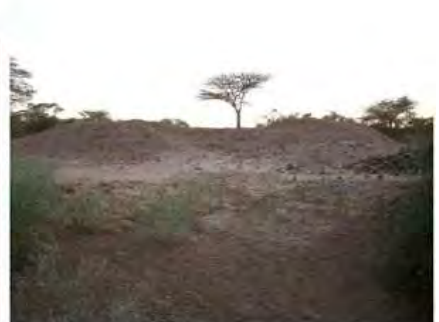
DSCN3952.JPG, Inappropriate/Inexistent Site Drainage, Inappropriate Dumping of Excavation Spoils, Vegetation Damage, Royal City
