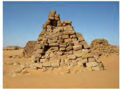
DSCN3859.JPG, Structural Deterioration of Pyramids, Southern Cemetery
