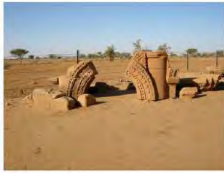
DSCN3997.JPG, The Kiosk - Naqaa, Naqaa, Degradation of Stone/ Masonry Elements, Inappropriate/Inexistent Site Drainage
