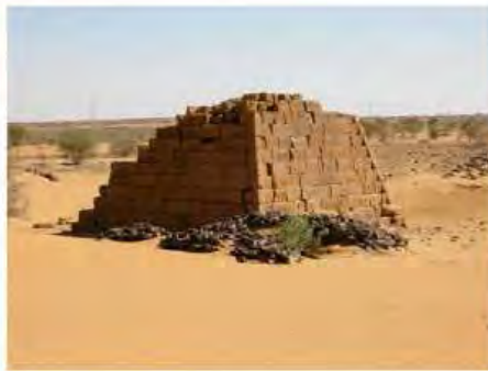
DSCN3865.JPG, Structural Deterioration of Pyramids, Southern Cemetery
