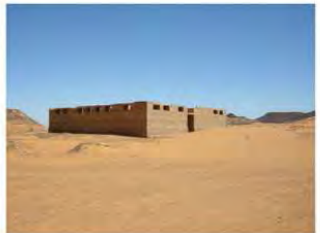
DSCN3815.JPG, Redundant/Inappropriate Visitor Infrastructure
