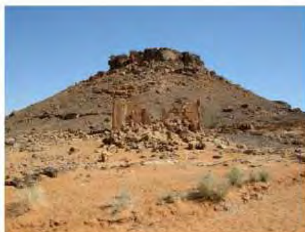
DSCN4138.JPG, Naqaa, Temple F, Structural Instability of Walls/ Collapse of Archaeological Features
