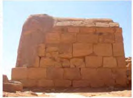
DSC06191.JPG, Musawwarat - Great Enclosure, Restoration Works
