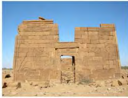
DSCN4047.JPG, Lion Temple B300 - Naqaa, Naqaa, Inaproprate/ Inexistent Site Drainage
