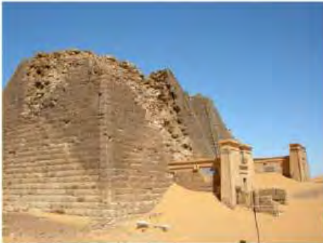
DSCN3774.JPG, Structural Deterioration of Pyramids, Public Safety Hazard, Northern Cemetery
