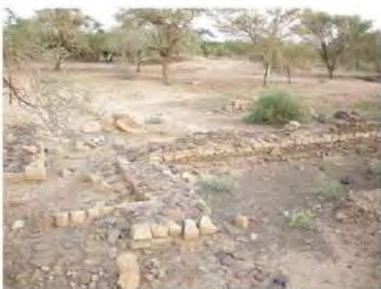
DSCN3950.JPG, Structural Instability of Walls/Collapse of Archaeological Features, Degradation of Stone/Masonry Elements, Vegetation Damage, Royal City
