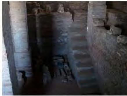
DSC06259.JPG, Inappropriate/Inexistent Site Drainage, Royal City
