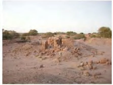
DSCN3993.JPG, Structural Instability of Walls/Collapse of Archaeological Features, Inappropriate/Inexistent Site Drainage, Inappropriate Dumping of Excavation Spoils, Royal City
