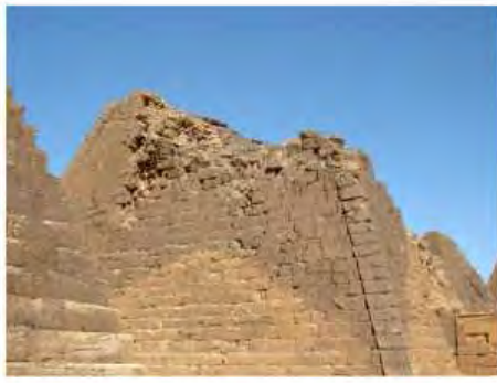
DSCN3757.JPG, Public Safety Hazard, Structural Deterioration of Pyramids, Northern Cemetery
