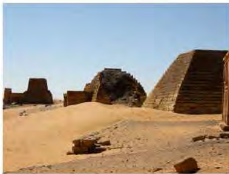
DSCN3760.JPG, Site Wide View, Structural Deterioration of Pyramids, Northern Cemetery
