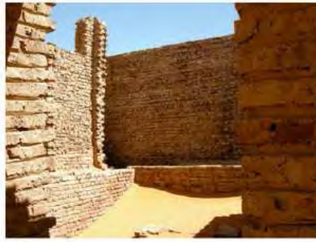
DSCN3817.JPG, Redundant/Inappropriate Visitor Infrastructure
