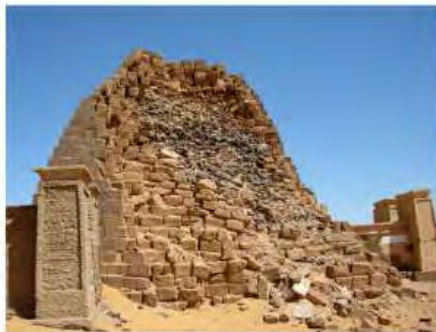
DSCN3802.JPG, Structural Deterioration of Pyramids, Southern Cemetery
