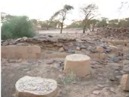
DSCN3947.JPG, Structural Instability of Walls/Collapse of Archaeological Features, Degradation of Stone/Masonry Elements, Royal City
