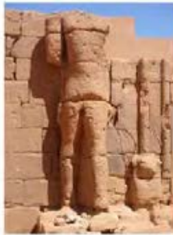
DSC06175.JPG, Musawwarat - Great Enclosure, Restoration Works
