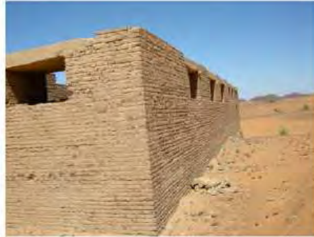
DSCN3820.JPG, Redundant/Inappropriate Visitor Infrastructure
