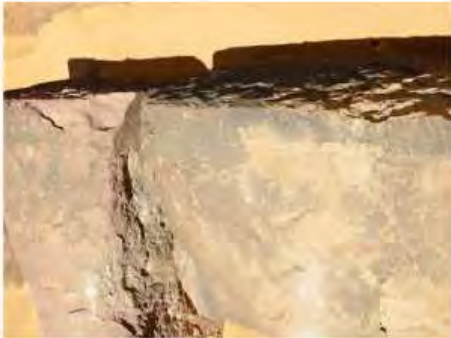
DSCN3807.JPG, Henkel Restoration, Southern Cemetery
