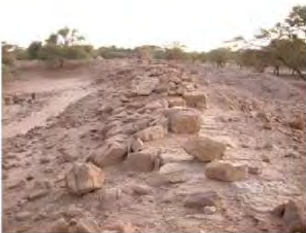
DSCN3974.JPG, Structural Instability of Walls/Collapse of Archaeological Features, Inappropriate Dumping of Excavation Spoils, Degradation of Stone/Masonry Elements, Royal City
