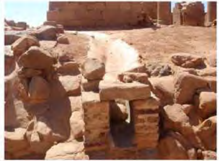
DSC06197.JPG, Musawwarat - Great Enclosure, Restoration Works
