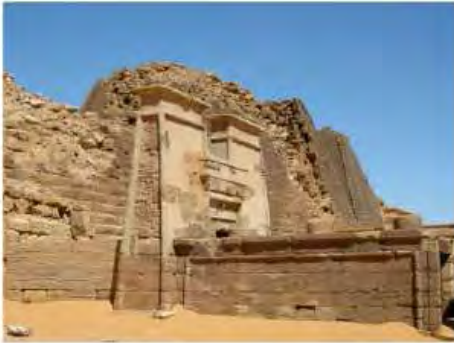
DSCN3771.JPG, Public Safety Hazard, Northern Cemetery
