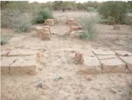
DSCN3935.JPG, Degradation of Stone/Masonry Elements, Structural Instability of Walls/Collapse of Archaeological Features, Inappropriate/Inexistent Site Drainage, Vegetation Damage, Royal City
