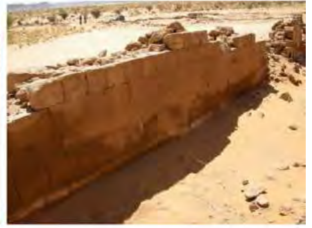
DSCN4175.JPG, Musawwarat - Great Enclosure, Restoration Works, Degradation of Stone/Masonry Elements, Salt Crystallization
