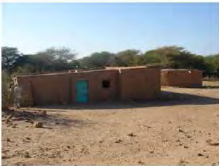
DSC06262.JPG, Redundant/Inappropriate Visitor Infrastructure, Royal City
