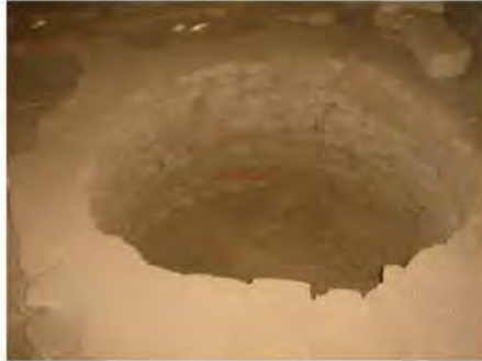
DSC06245.JPG, Inappropriate/Inexistent Site Drainage, Degradation of Stone/Masonry Elements, Royal City
