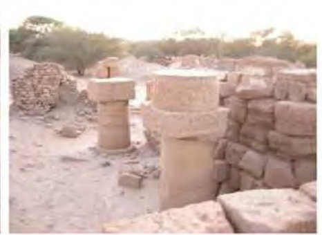
DSCN3982.JPG, Structural Instability of Walls/Collapse of Archaeological Features, Inappropriate Dumping of Excavation Spoils, Inappropriate/Inexistent Site Drainage, Royal City
