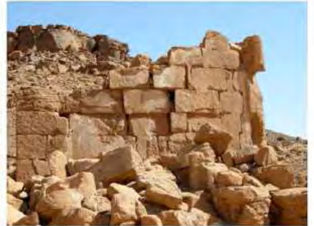
DSCN4143.JPG, Naqaa, Temple F, Exposure and Deterioration of Ancient Plasters, Structural Instability of Walls/Collapse of Archaeological Features, Structural Instability of Walls/Collapse of Archaeological Features
