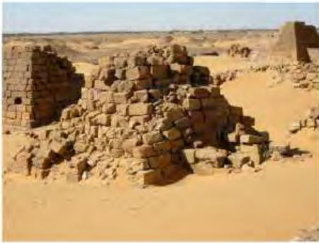
DSCN3851.JPG, Structural Deterioration of Pyramids, Southern Cemetery
