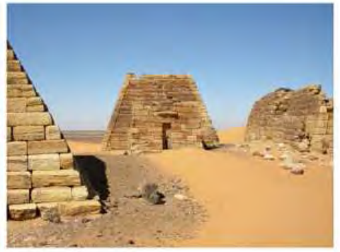
DSCN3746.JPG, Public Safety Hazard, Northern Cemetery
