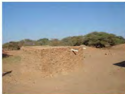
DSC06266.JPG, Redundant/Inappropriate Visitor Infrastructure, Royal City
