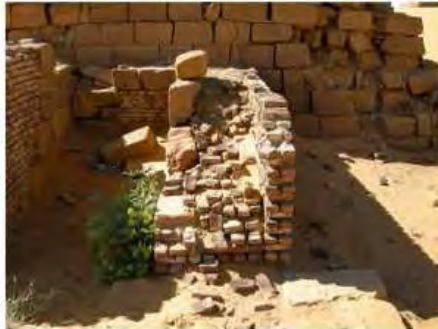
DSCN3837.JPG, Failure of Past Repair Work, Southern Cemetery
