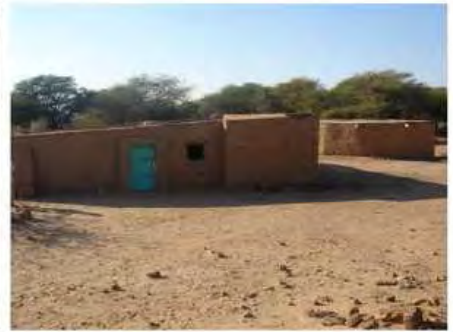
DSC06261.JPG, Redundant/Inappropriate Visitor Infrastructure, Royal City
