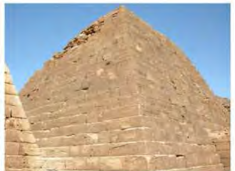
DSCN3755.JPG, Public Safety Hazard, Northern Cemetery
