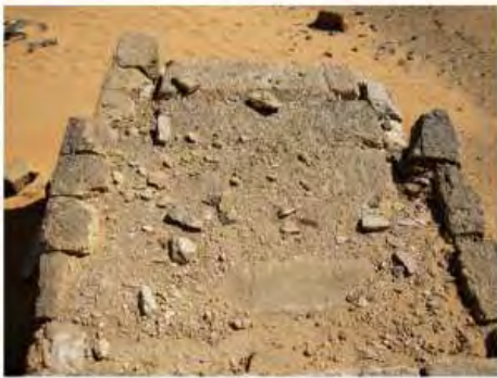
DSCN3732.JPG, Structural Deterioration of Pyramids, Northern Cemetery
