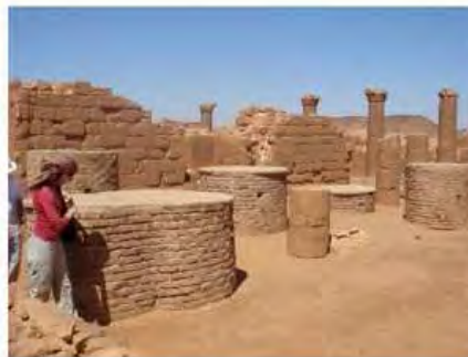
DSC06208.JPG, Musawwarat - Great Enclosure, Restoration Works
