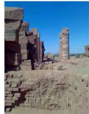
09112008247, Naqaa, Amun Temple, Deterioration of Ancient Mud Structures
