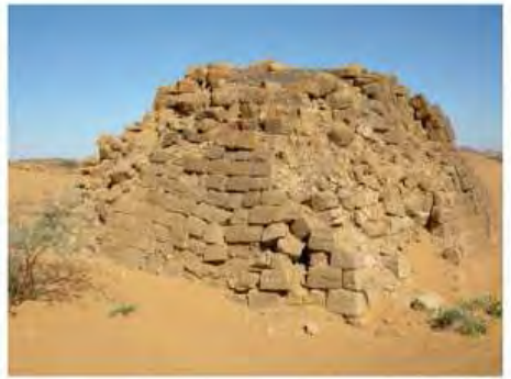
DSCN3844.JPG, Structural Deterioration of Pyramids, Southern Cemetery
