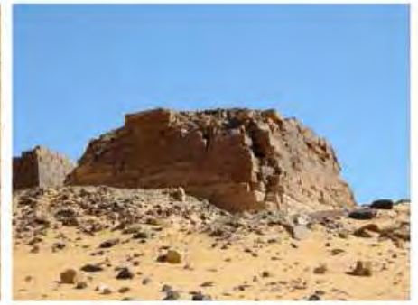
DSCN3710.JPG, Structural Deterioration of Pyramids, Northern Cemetery
