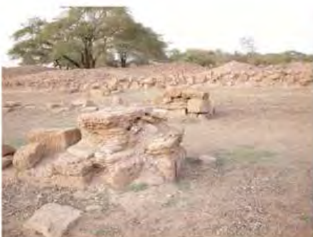
DSCN3962.JPG, Degradation of Stone/Masonry Elements, Structural Instability of Walls/Collapse of Archaeological Features, Inappropriate/Inexistent Site Drainage, Royal City
