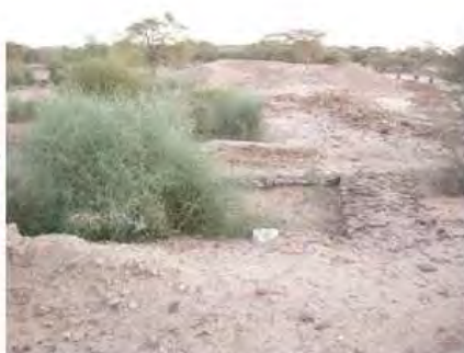
DSCN3951.JPG, Vegetation Damage, Inappropriate/Inexistent Site Drainage, Inappropriate Dumping of Excavation Spoils, Royal City
