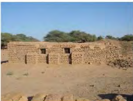
DSC06265.JPG, Redundant/Inappropriate Visitor Infrastructure, Royal City
