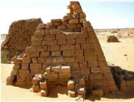
DSCN3857.JPG, Structural Deterioration of Pyramids, Southern Cemetery
