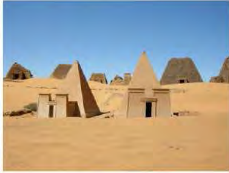
DSCN3784.JPG, Site Wide View, Salt Crystallization, Northern Cemetery
