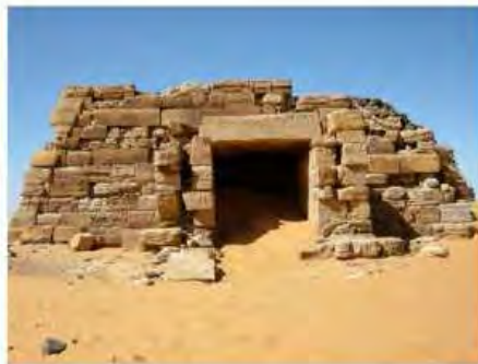
DSCN3727.JPG, Structural Deterioration of Pyramids, Northern Cemetery
