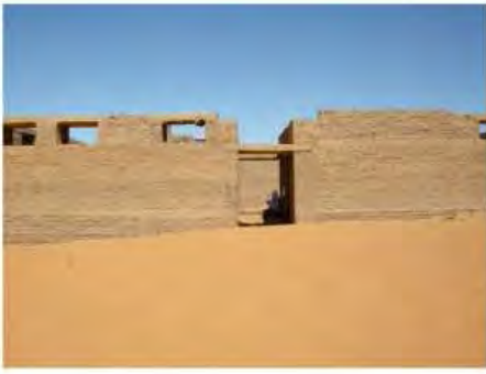
DSCN3816.JPG, Redundant/Inappropriate Visitor Infrastructure
