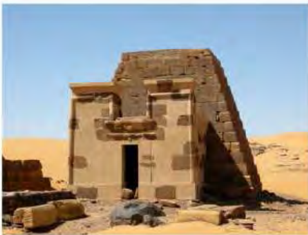
DSCN3801.JPG, Henkel Restoration, Southern Cemetery
