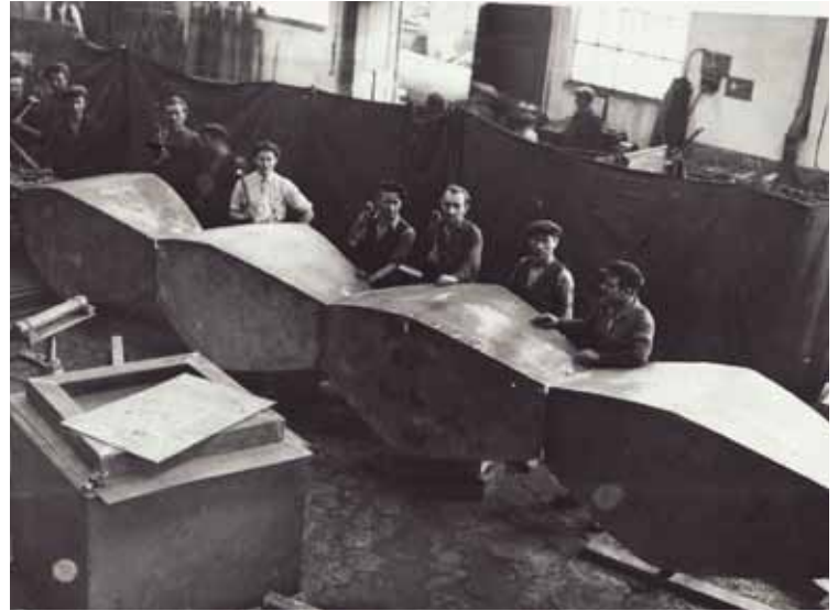
Test fitting of the Endless Column in the Petroșani Central Workshops. 1937 (NIH Archive)
