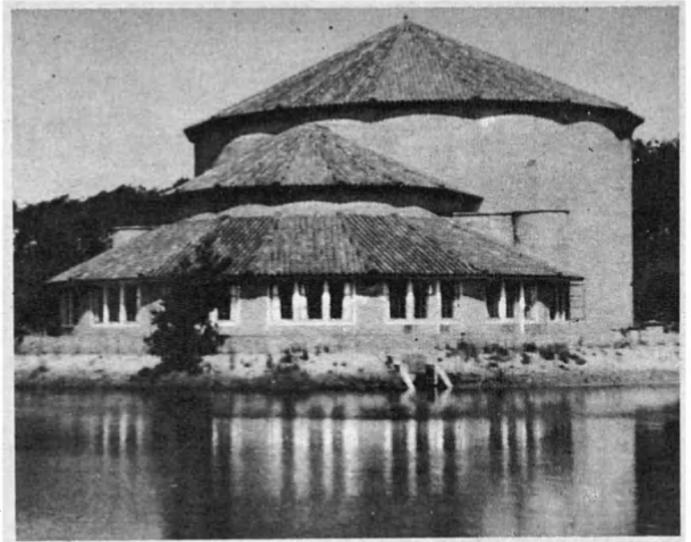
This reinforced concrete shelter in the Netherlands was built before the last war to house works of art in case of hostilities. When World War II came hundreds of paintings, statues and other treasures were placed in its vaults for safekeeping and were thus saved from destruction. Entire framework is made of steel bars one inch in diameter. The walls are 15 feet thick and the roof, at highest point, 30 feet thick. In most structures roof is most vulnerable.
