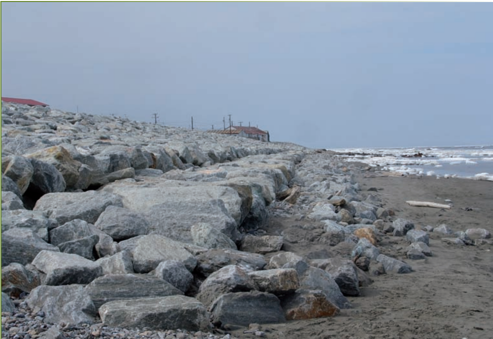
Shishmaref Revetment Project (photo: Sharon McClintock).
