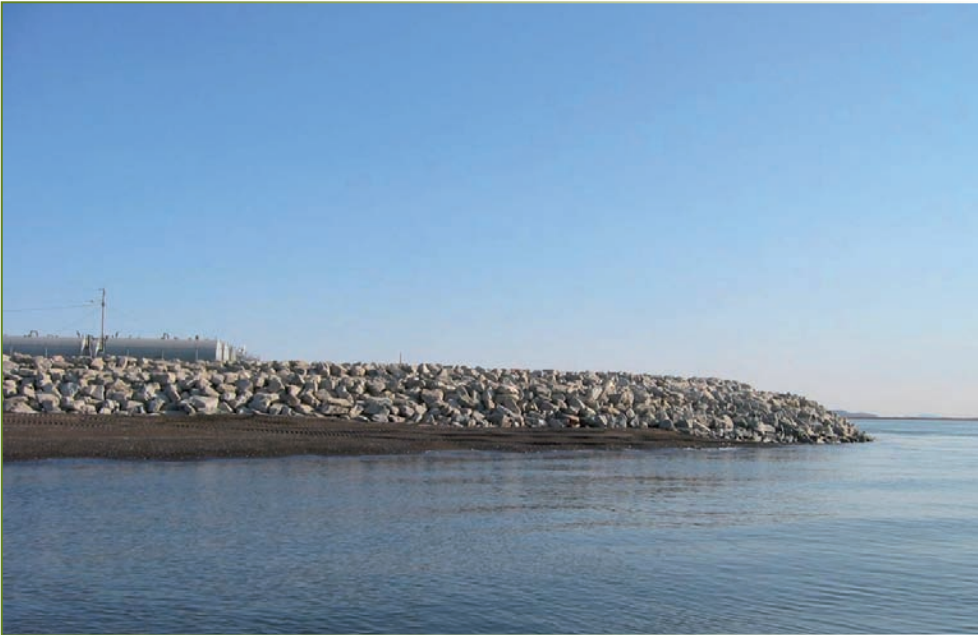
Kivalina Revetment Project 2008-9 (photo: Ron Cothran, MLA).
