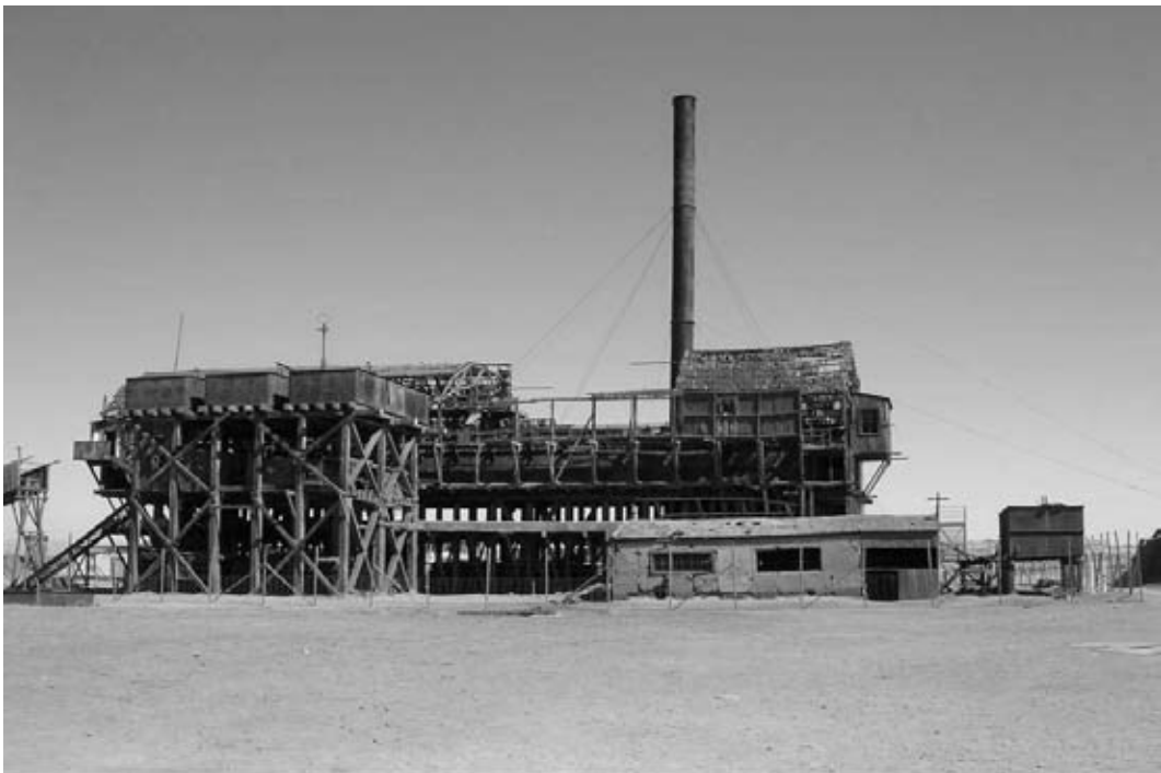
Leaching Shed of the Santa Laura Saltpeter Works
