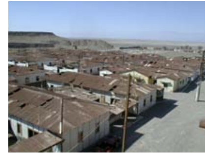
Vista general de los techos del campamento de Humberstone General view of the roofs, Humberstone living quarters Sergio Rowe, 1999
