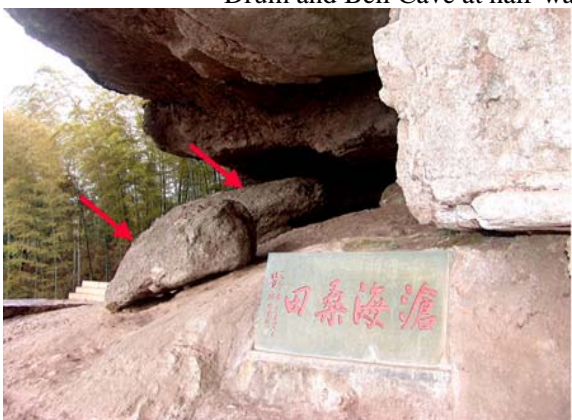
Fairy Meeting Cave at the foot of the Peak Lang and residual falling stones
