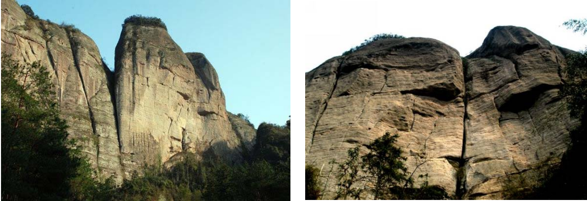
System of cleavages and cracks in the landscape-constituting strata of Danxia landform
