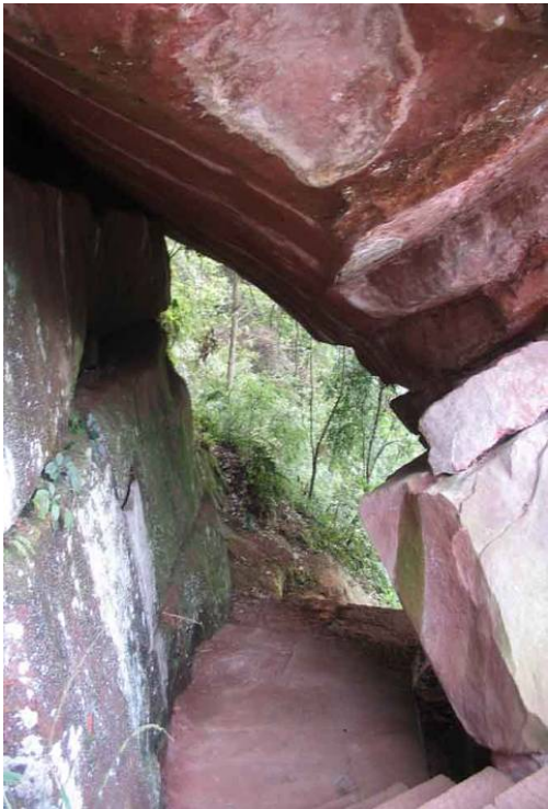
Collapsed rock cave
