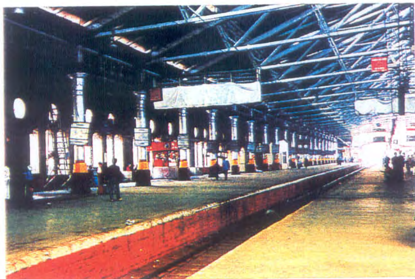
20. View of the original concourse- reflecting high engineering skills in use of steel in late 19 th cent
