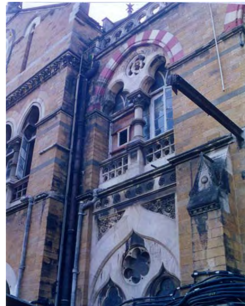
Existing water supply distribution
