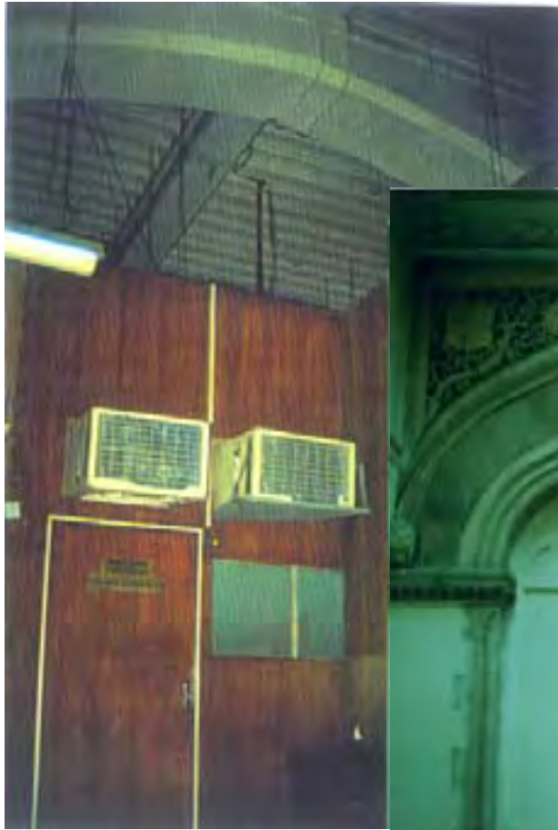
Sensitively Designed Partition for filling up of an arch
