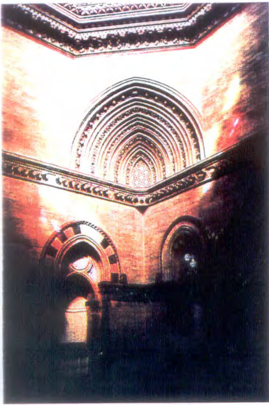
24. Decorative squinches/pendentives in the staircase area to make the square plan an octagon.
