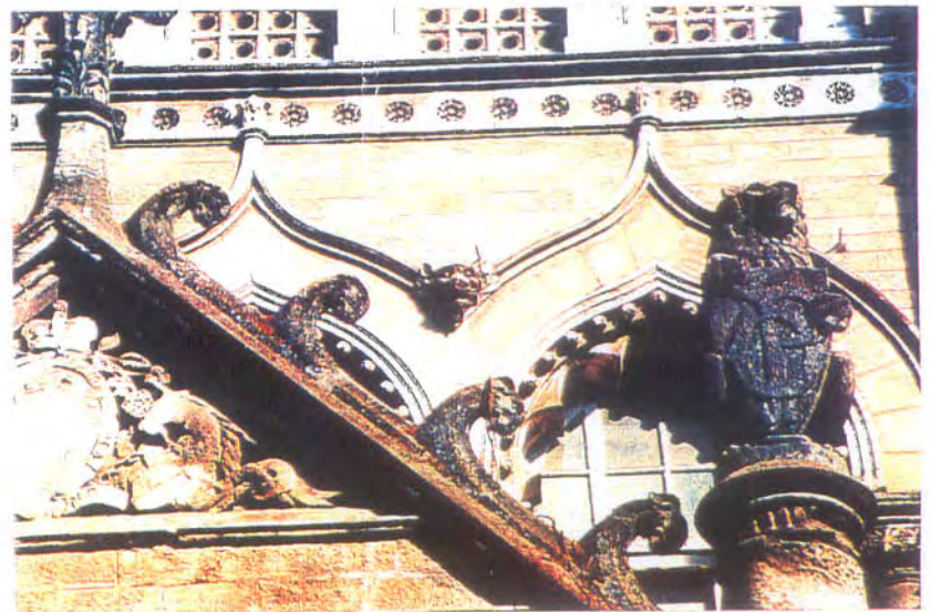
15. Many of the openings have unfortunately been sealed, the proposed restoration project aims in opening these up in future.
