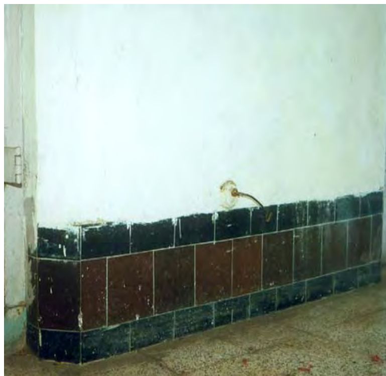
Mosaic Tiles laid later on
