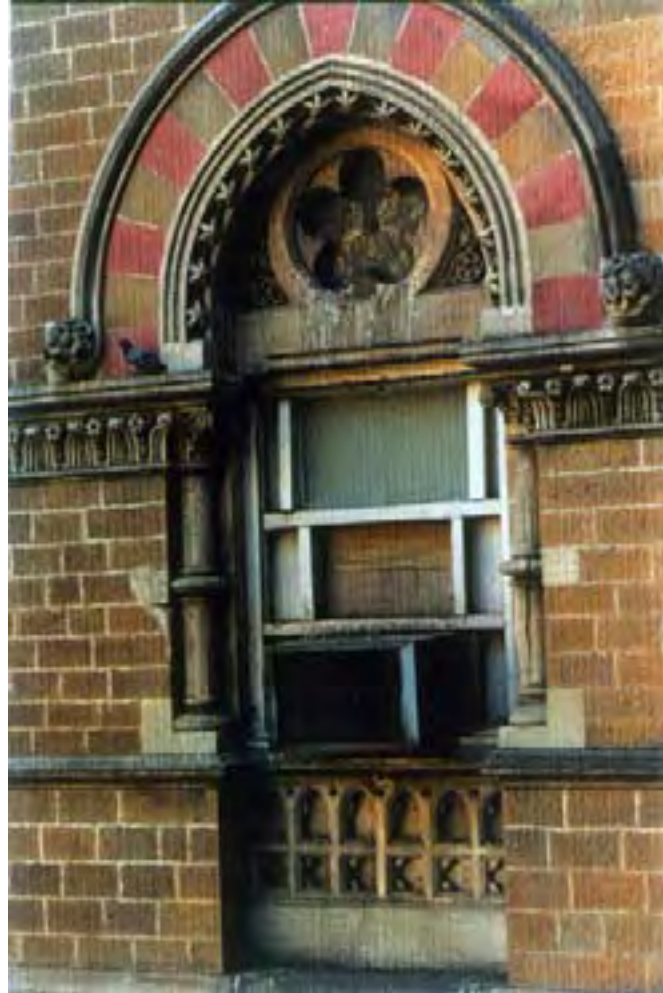
ARCH OPENINGS FILLED UP IN DIFFERENT MANNERS EVERWHERE
