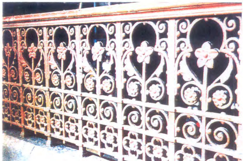
34. highly decorated and originally richly coloured and gilded WI railing was one of the highlights of 2007
