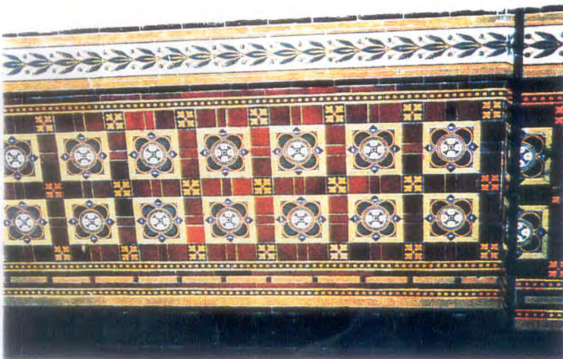
33 Encaustic tile dado in banqueting hall
