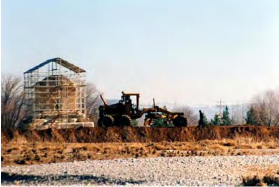
Constructing dikes against the floods
