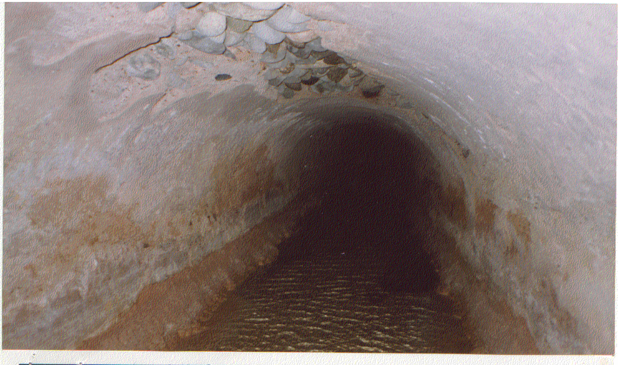
Interior of large daoudi falaj lined with clay and stones
