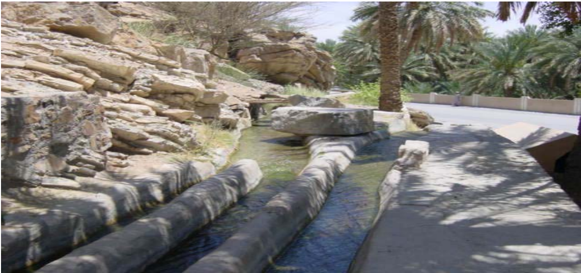
4 Falaj Al-Khatmeen: Distribution point, showing division into three equal flows
