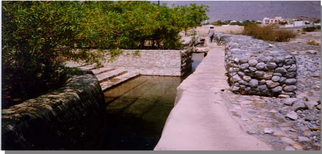
Falaj Daris: View of shari'a , showing access platform for drawing water for domestic purposes
