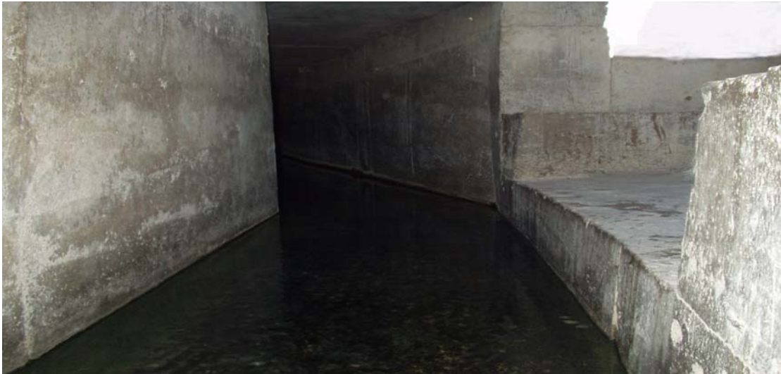
Falaj Al-Malki: Detail of shari'a , showing state of conservation
