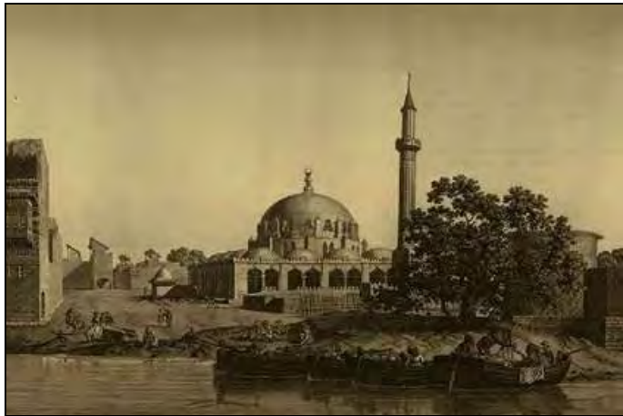
Image 31: Sinan Pasha Mosque, Cairo (Source: Turkey Pious Foundation General Directorate)
