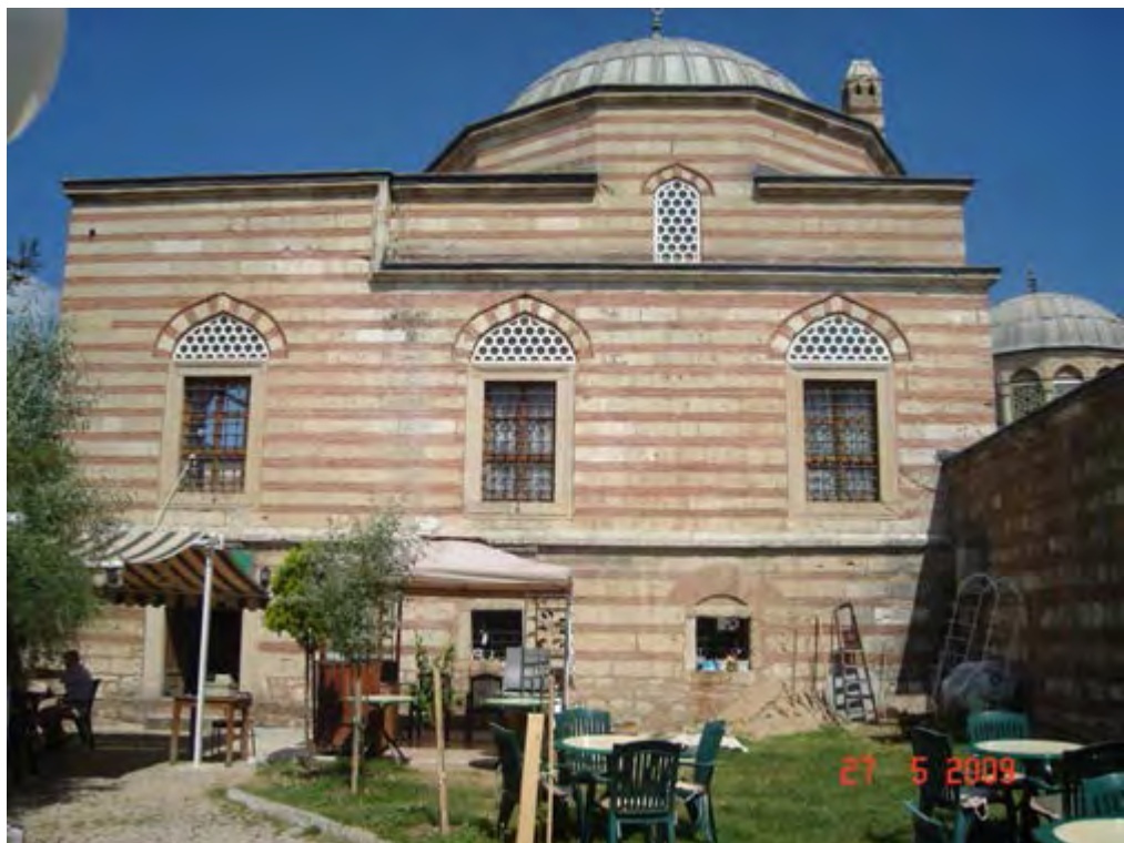
Photo 14- Side Facade of Primary School
