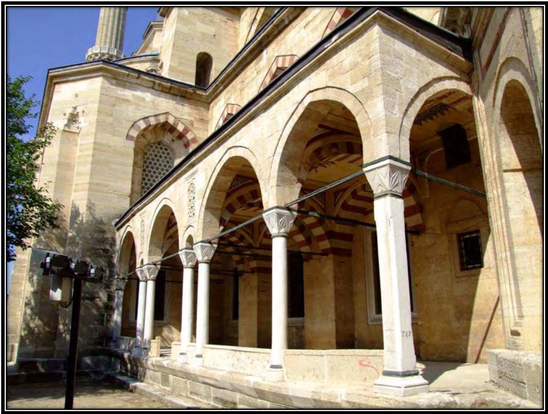
99- GALLERIES AT MİHRAB FACADE
