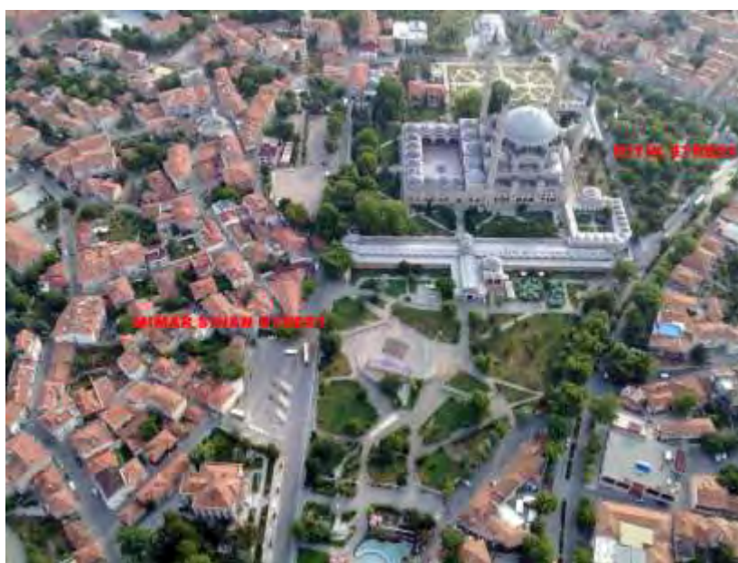
Selimiye Complex (aerial view)
