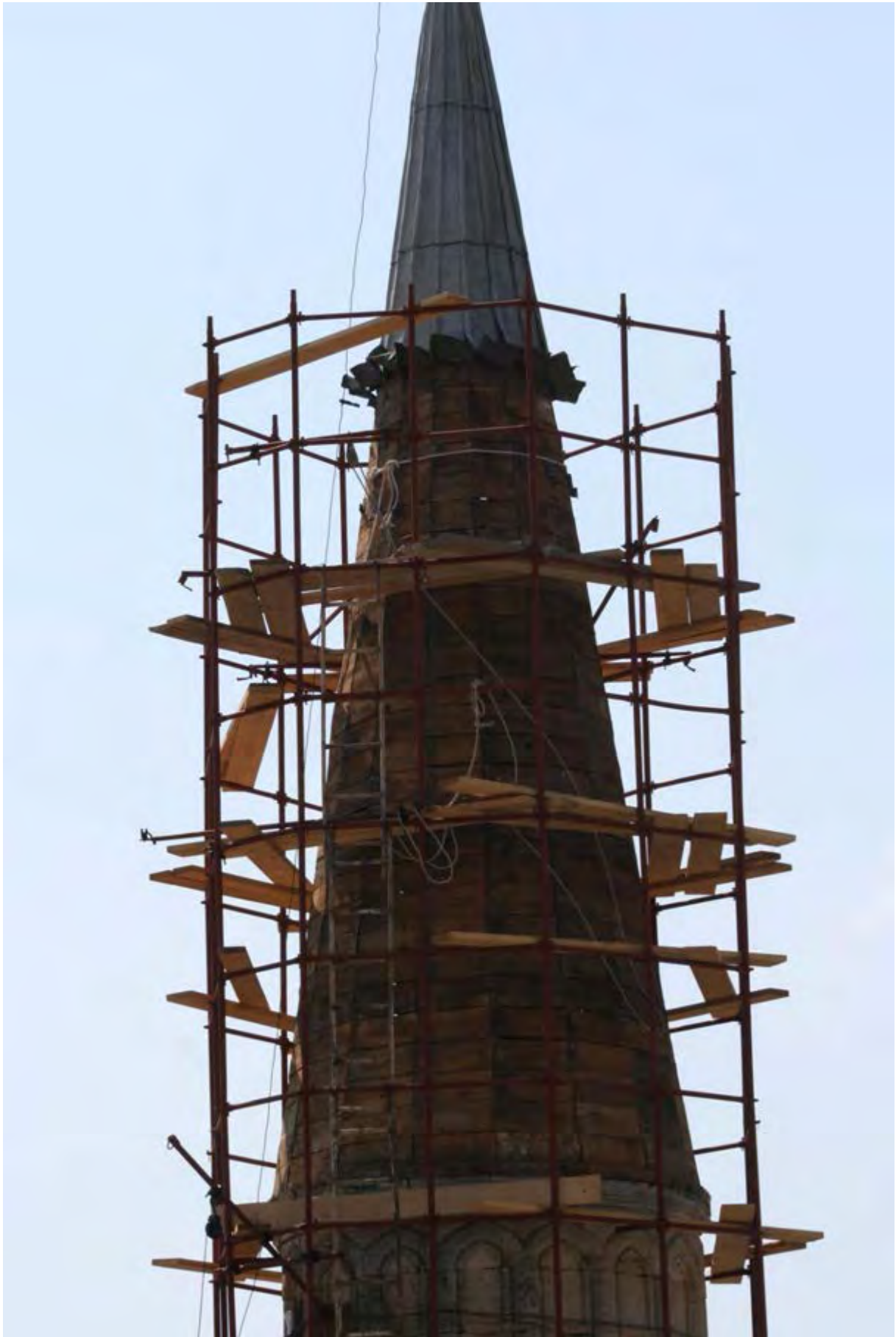
PHOTO 6- REMOVING THE LEADS OF SPIRE
