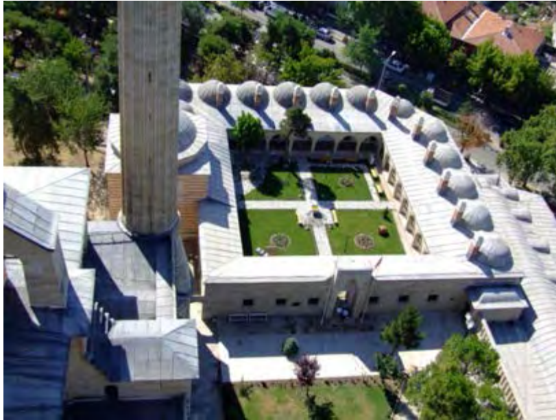
Photo 7- Aerial View of with the Inner Garden
