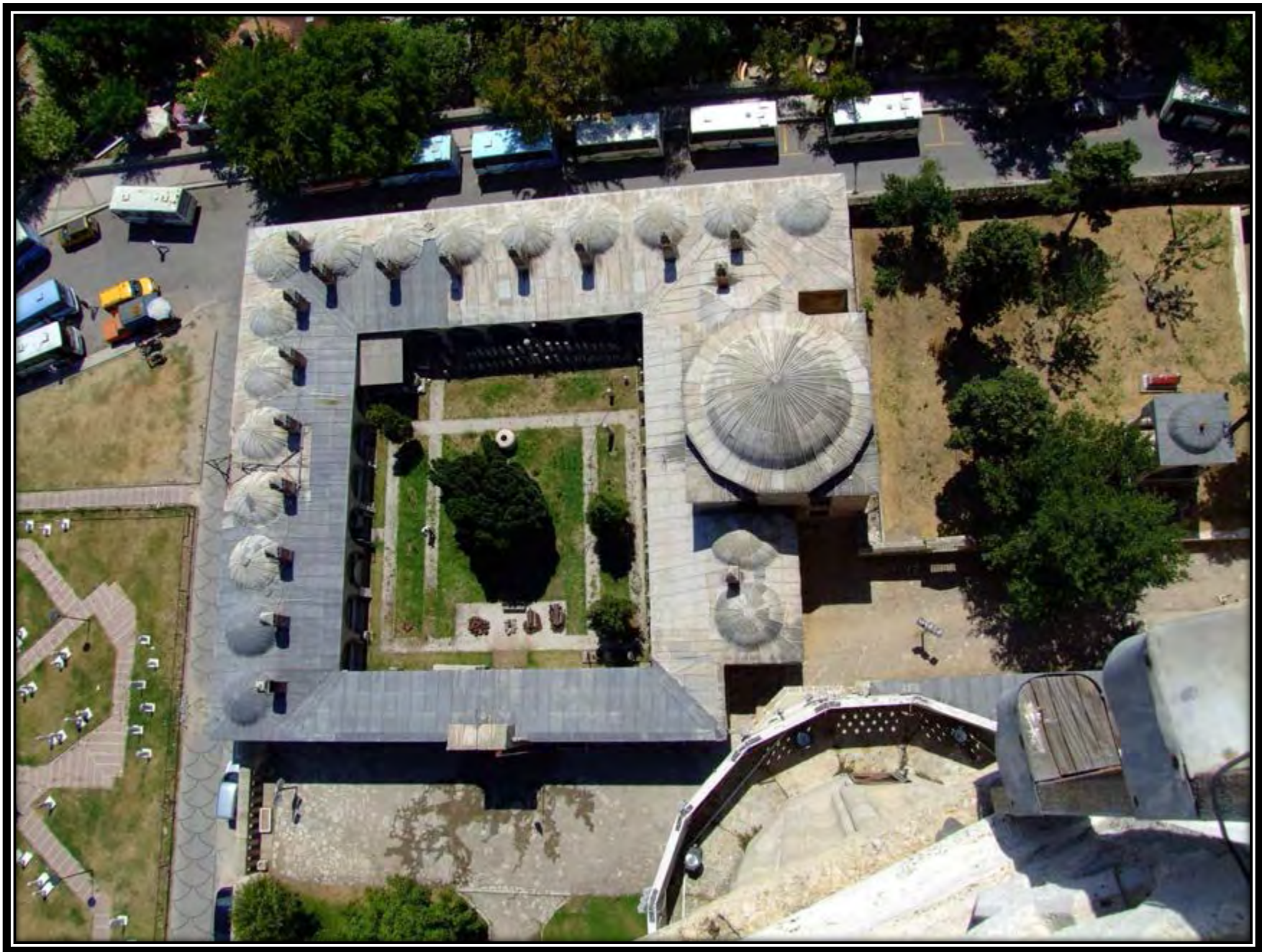
14- DAR'UL HADIS MADRASA'S DOMES AND VAULTS
