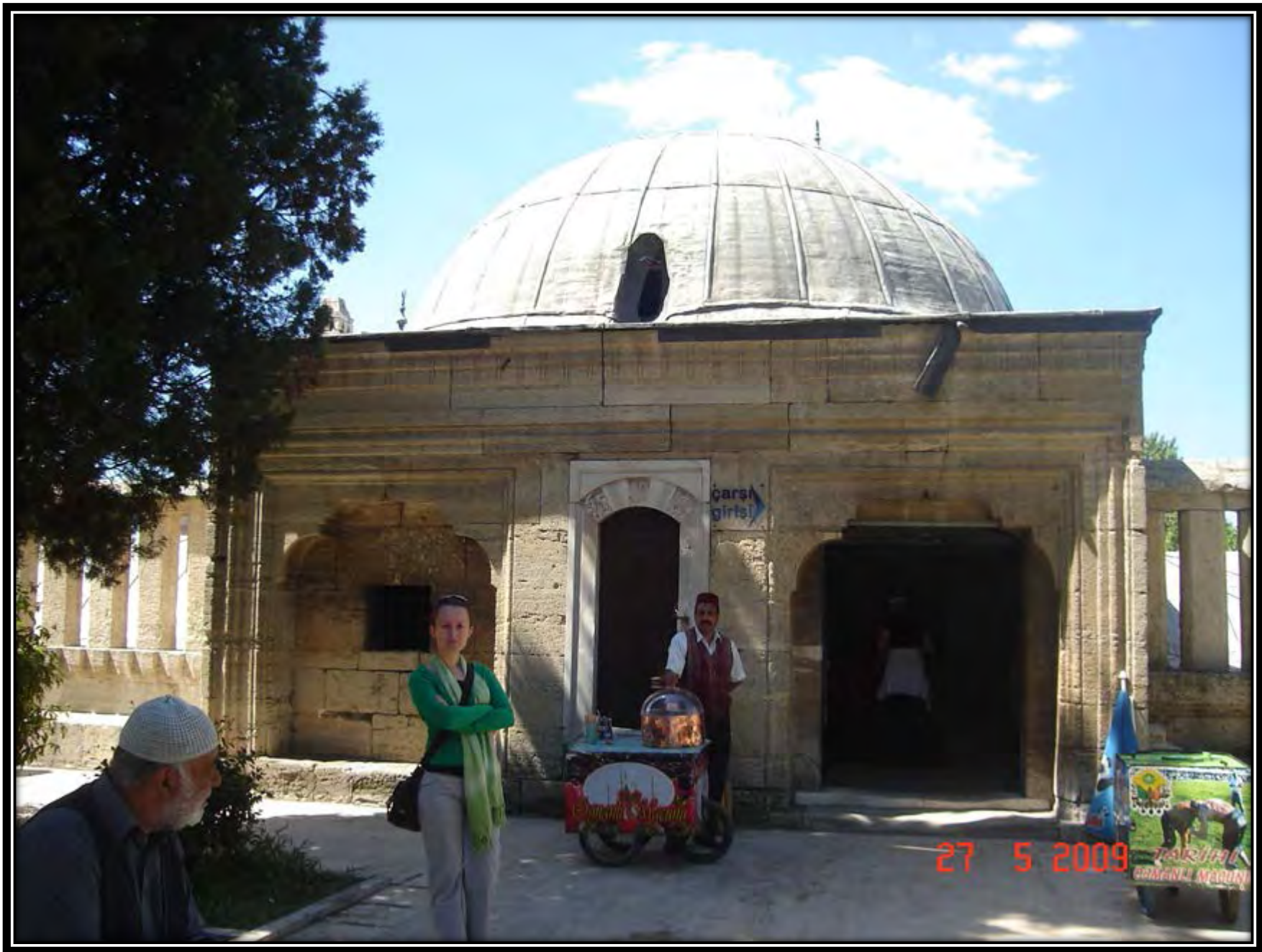
27- CONNECTION DOOR OF ARASTA BAZAAR TO OUTER COURTYARD
