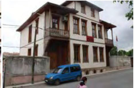
EDİRNE MUFTU's OFFICE (Traditional House)
