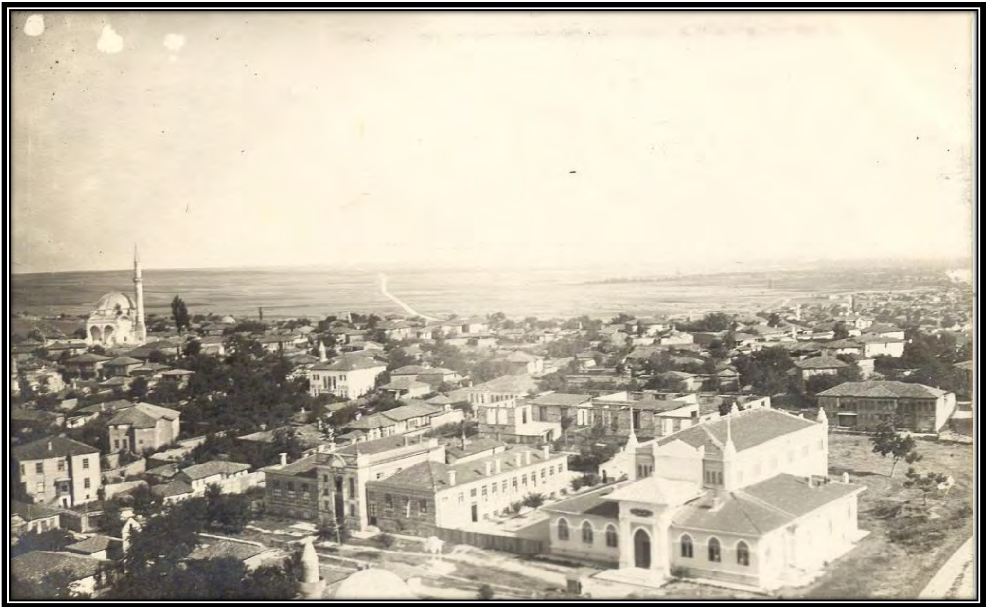
145- ITTIHAT AND TERAKKI CLUB'S BUILDING AND TICARET SCHOOL (1916)
