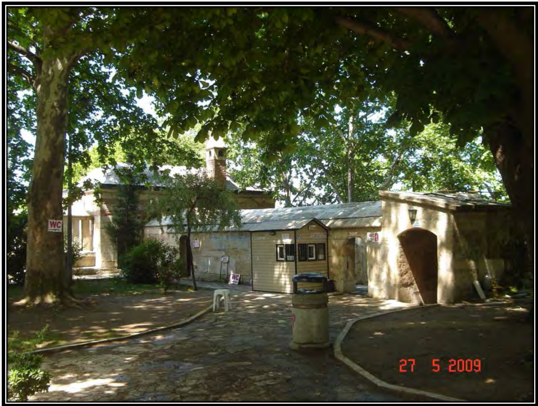
36- MUVAKKITHANE NEAR WC'S FROM OUTER COURTYARD
