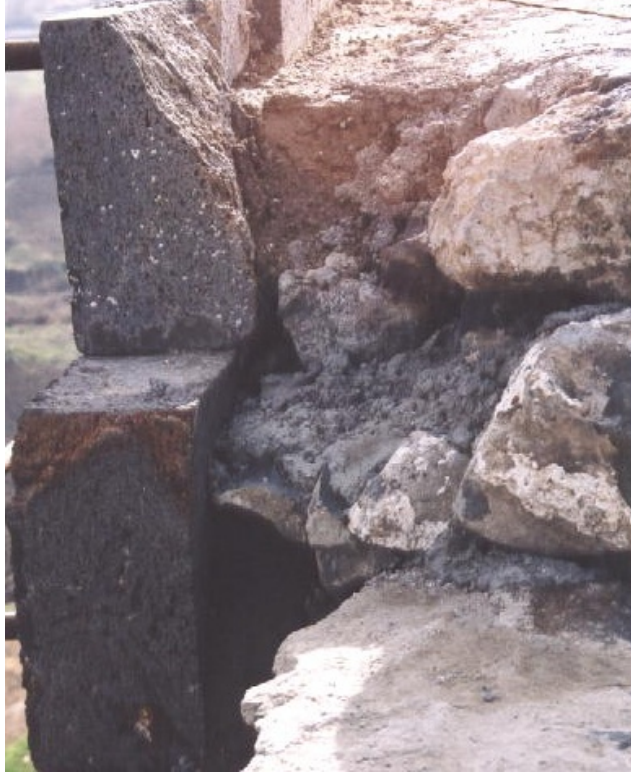
Picture 13. Usage of cement added mortar materials
