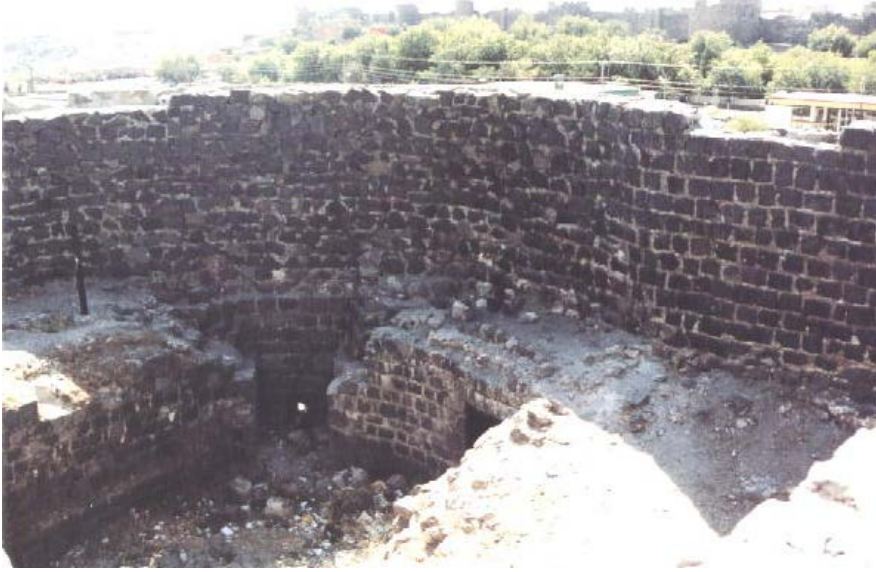
Picture 8. Tower's last section's status prior to the restoration.
