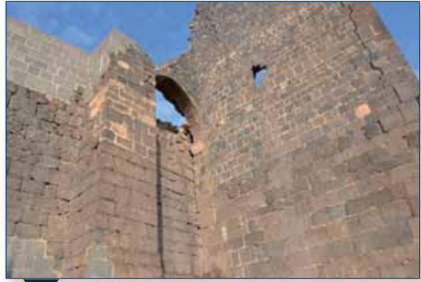
image 2a- 56: Lelebikıran Tower, the connection point with the city walls
