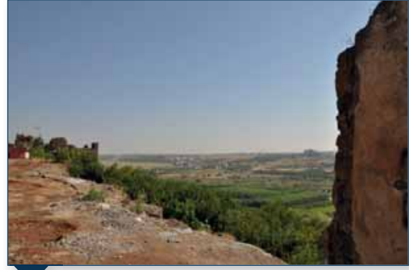
Image 4- 20: The demolished part between the Tower numbers 66 and 67.
