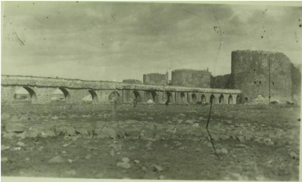
Photo 2: The Kantara (aqueduct) that provided water delivery to the city via Gözeli water sources 1928
