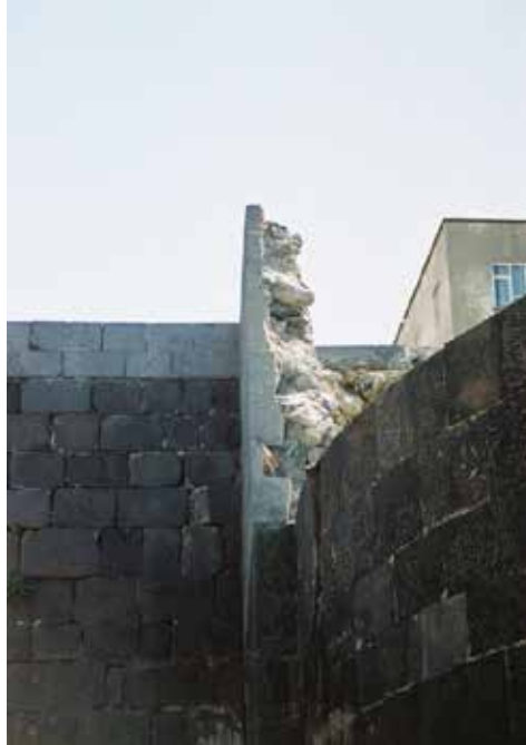
Picture 17. Using cement heavy mortar material
