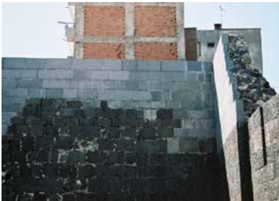
Picture 14. Wall façade that is covered with stone material that is not in harmony with the fabric.
