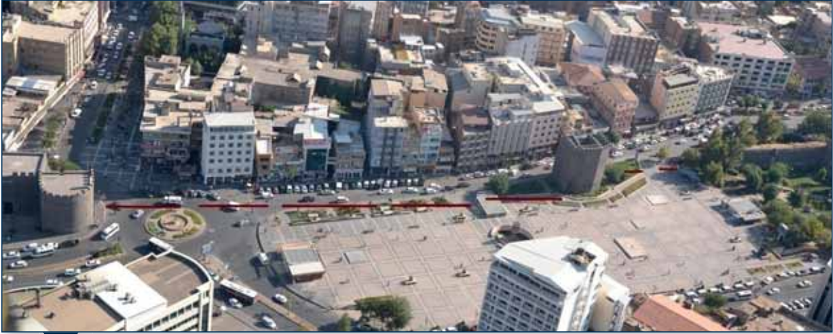
image 2b- 26: The Current State of the Demolitions in the Northern Part of the Fortress
