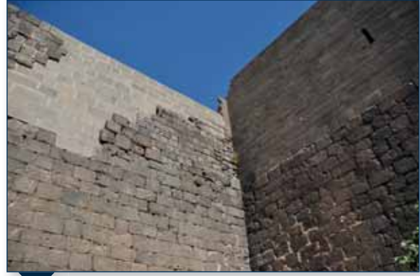
Image 4-49: The stones of different thickness and sizes used in the restorations
