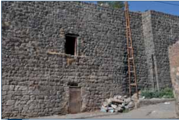
Image 4- 2: A tower from İçkale (the Castle) used as a barn
