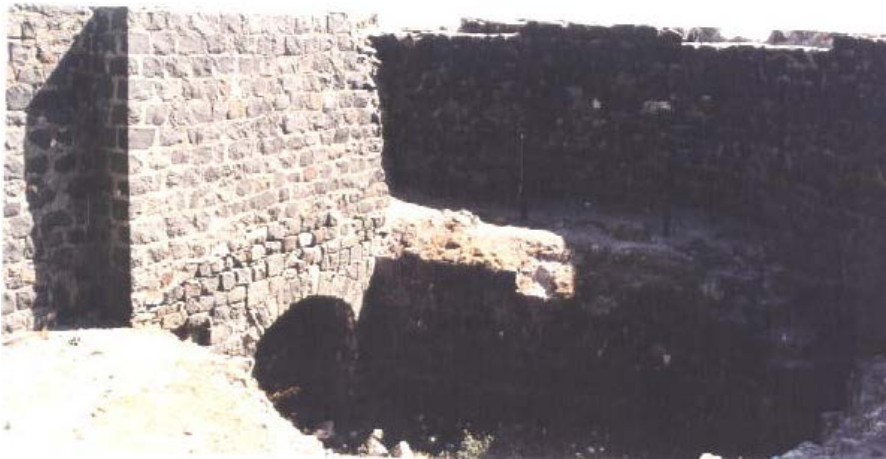
Picture 7. Tower's last section's status prior to the restoration.
