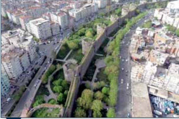
Image 4- 44: The high rise buildings near the City Walls
