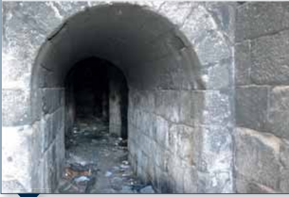
Image 4- 27: Inside of the tower of the Urfa Gate towers(Tower number 21)
