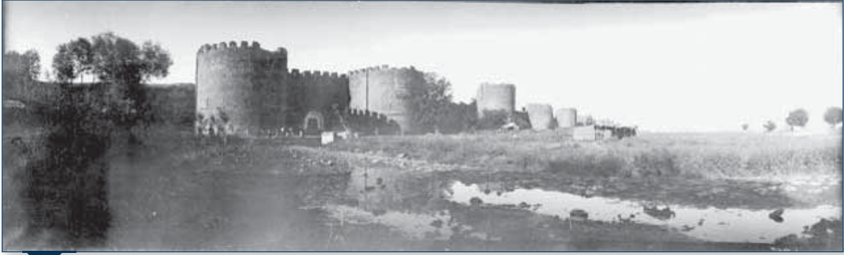
image 2b- 23: The Photos before the Demolition in the Northern Part of the Fortress, 1909
