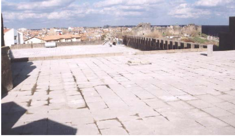
Picture 6. Completely renewed top cover.
