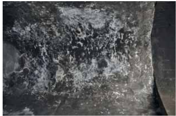
Image 4- 26: Ceiling of Urfa Gate
