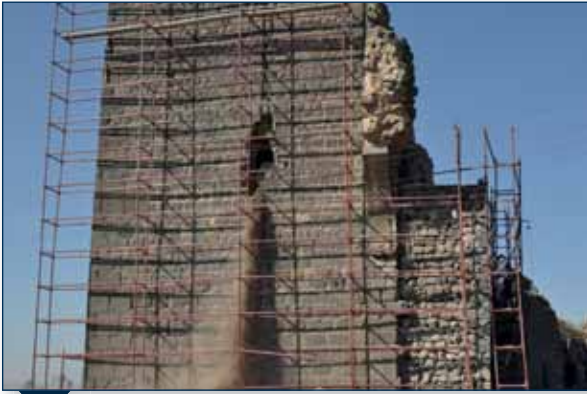
Image 4-48: Repair of Leblebi Kıran Tower (2013)
