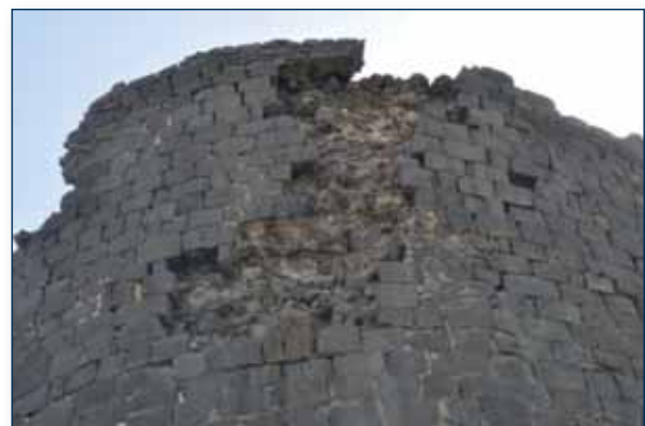
image 2a- 83: Wall masonry, towers number 18-20
