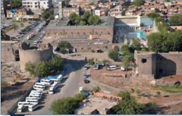
image 2b- 29: Mardin Gate after Demolition
