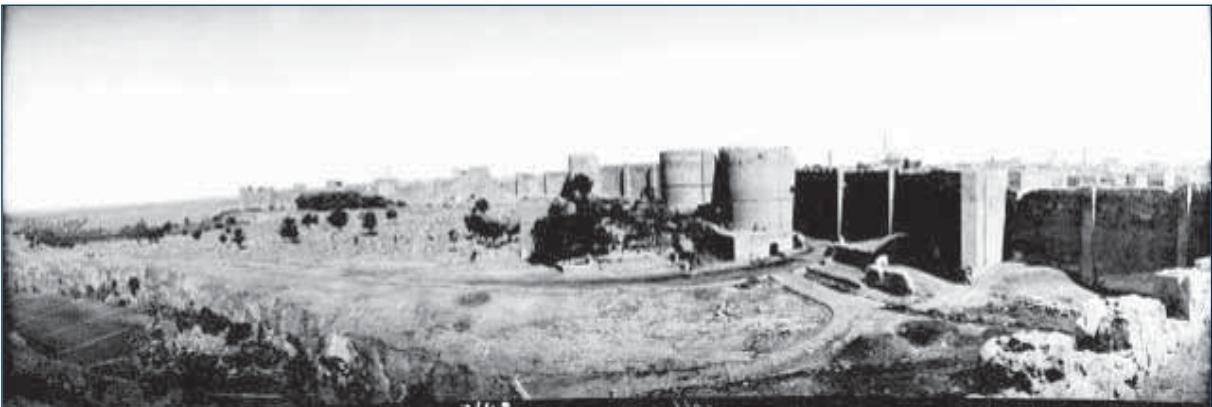
image 2b- 28: The Photos before the Demolition in Mardin Gate, 1909
