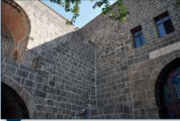
Image 4-47: Repair of Dağ Gate Towers
