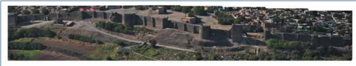
Image 4- 19: The view of the 3rd part of the City Walls and the demolished part between Leblebi Kıran(62) and Fındık (63) Towers
