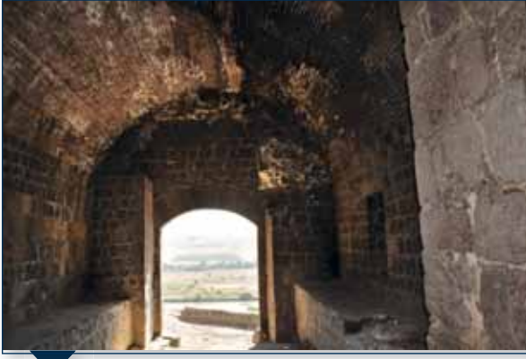
Image 4- 31: Inside of Yeni Gate
