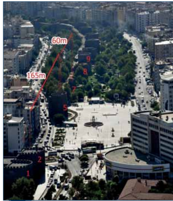
Image 4- 12: The missing parts in the 1st section of the City Walls
