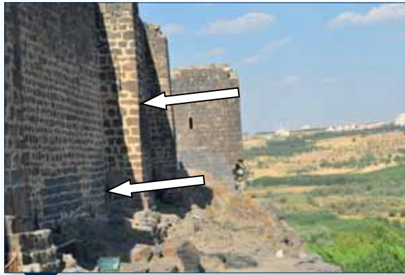
image 2a- 61: The buttresses between the towers
