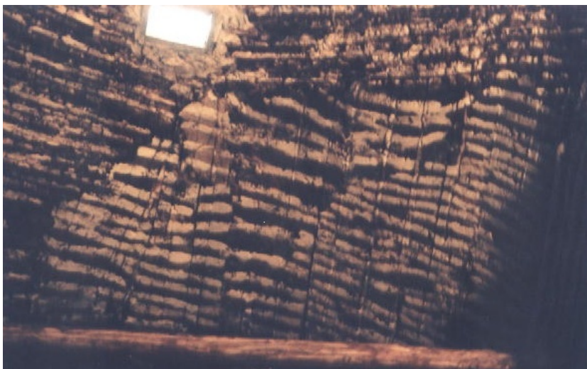
Picture 3. Surface attempted to be given the visual perception of jointings via painting.
