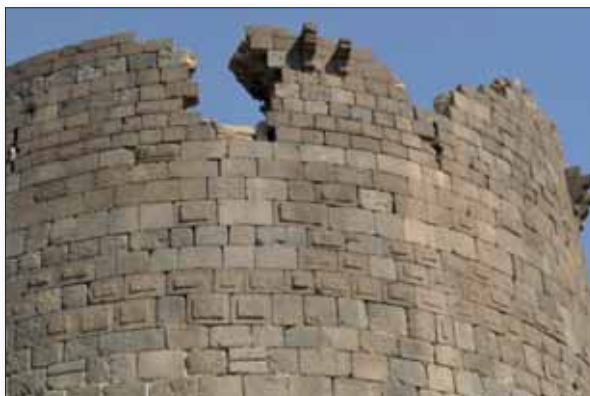
image 2a- 77: Usage of cylindrical and pumped stone in towers (towers 11)
