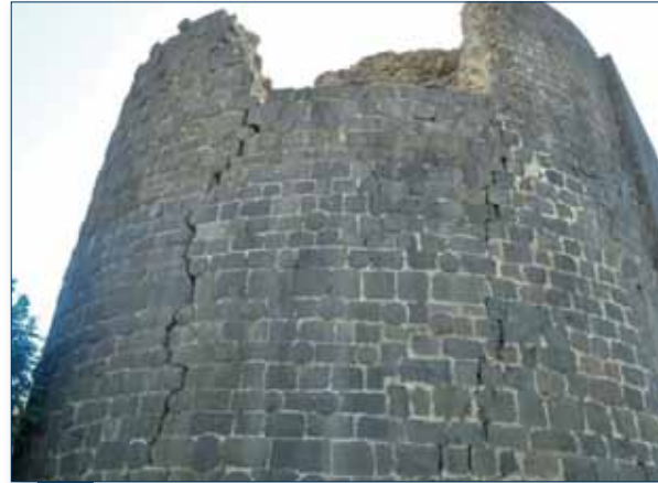
image 2a- 78: Usage of cylindrical and pumped stone in towers (towers 26)
