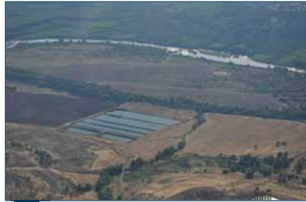
Image 4- 53: Waste Water Treatment Plant of Dicle University
