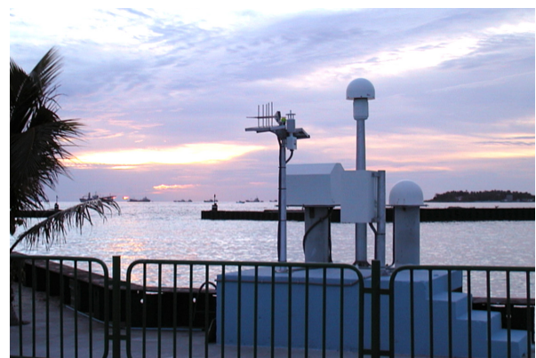
Figure 4. GLOSS Core Network tide gauge station No. 28 at Male, Maldives equipped with a continuous GPS receiver (highest dome) collocated with water level sensors (photo courtesy of D. Caccamise).
