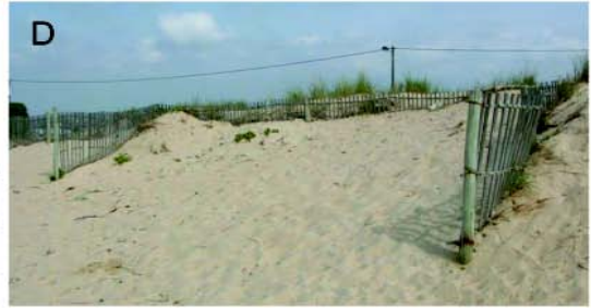
A sand fence system filled with sand and highly ineffective
