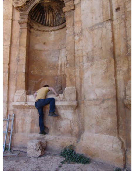
Figure 8.13: Anthropogenic action related to the behaviour of the visitors. The fact that a capital is near the niche helps the visitors climb over. The stone surface is already much damaged with a glossy layer. In some parts, the original stone surface is completely lost.
