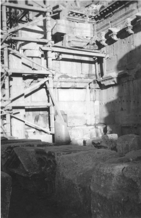
Figure 7.4 & 7.5: The restoration of the south wall of the chamber: dismantling the deformed wall (left), repositioning the carved stone blocs into their original positions (right). Photograph around 1960. (DGA iconographical inventory)
