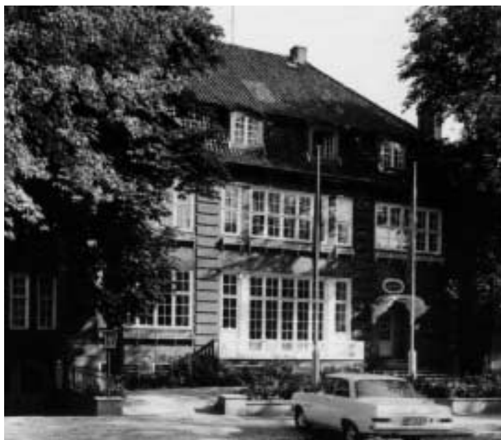
The building at Feldbrunnenstraße 70 where the Institute was housed from 1952 to 1978
