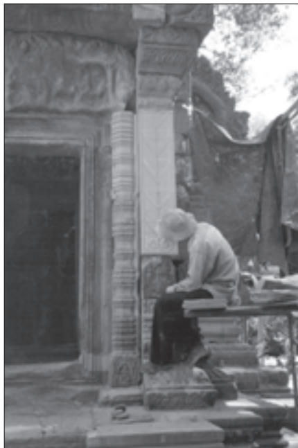
Chau Say Tevoda Temple. Restoration works by Chinese team
