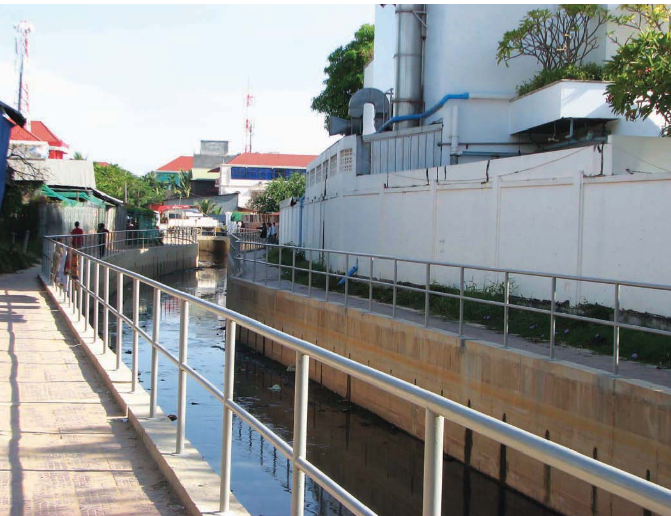
Waste water disposal line - Siem Reap town
