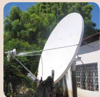
Satellite dish installed at the Institut Halieutique et des Sciences Marines in Tulear, Madagascar, to facilitate VSAT Internet access. The Very Small Aperture Terminal is a ground station used to communicate data via satellite.
