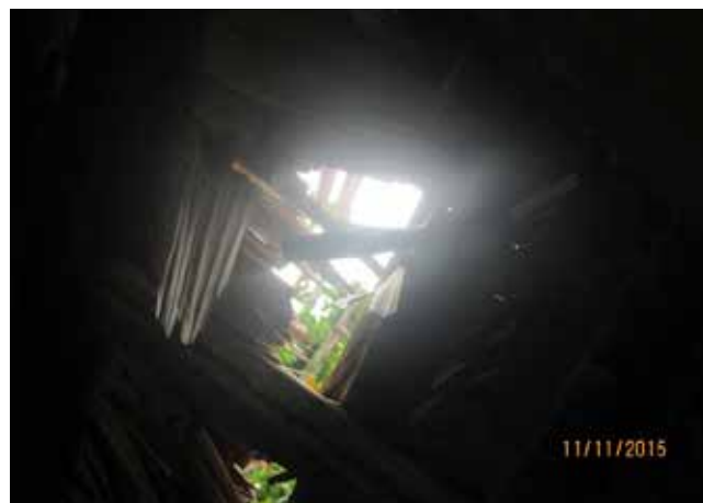
Figure 11: While the Nikaura Nakamal sustained very little damage during Tropical Cyclone Pam, there are now holes in the natangura thatch, which exposes the structural members to the elements.
