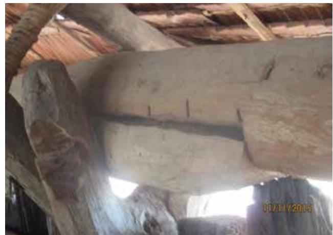
Figure 14: Post/beam connection detail (post- Tropical Cyclone Pam).
