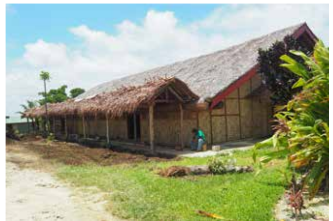
Figure 38: The Chiefs' Nakamal being reconstructed in February 2017
