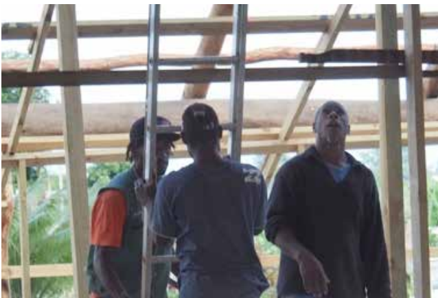
Figure 36: Builders working on the reconstruction of the Chiefs' Nakamal in July 2016.
