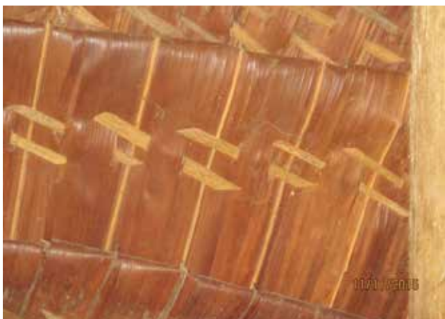
Figure 13: The majority of the natangura roof thatching on the Nikaura Nakamal remains in reasonable condition post- Tropical Cyclone Pam.
