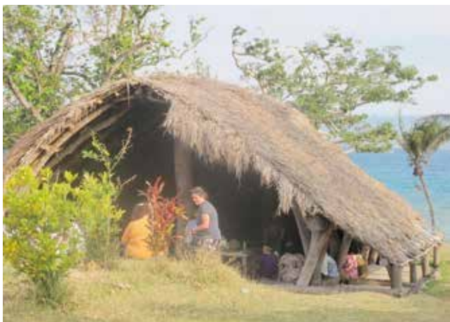
Figure 20: View of the Taloa Farea showing the damage made by Tropical Cyclone Pam to the side entry and front eaves; however, overall the farea fared very well and was still being used as per usual. At this time the village was hosting both a church group workshop and a tour of the farea by architecture students from Australia.
