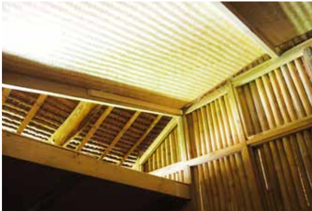
Figure 40: The reconstructed interior utilises woven pandanus ceiling linings and bamboo infill walls.
