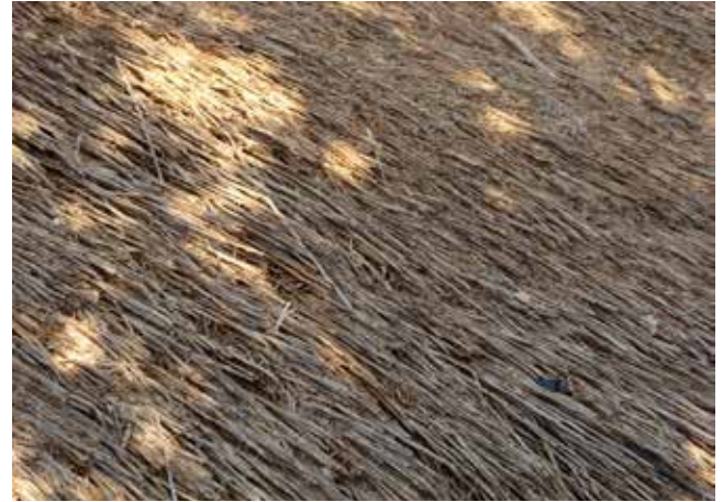
Figure 18: The thick layer of wild cane thatching over the farea (pre- Tropical Cyclone Pam).
