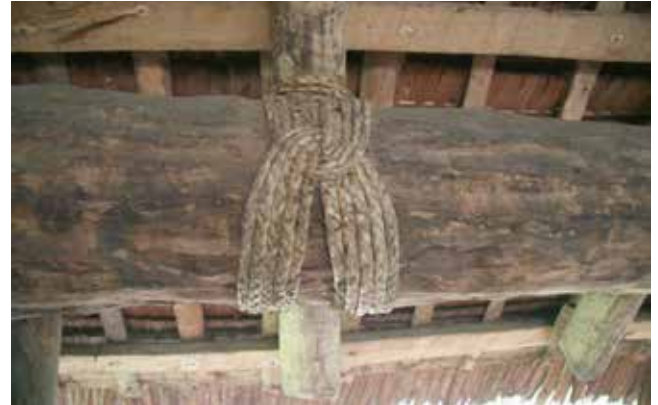
Figure 6: The large edge beam of the Mangarisu Nakamal (pre-Tropical Cyclone Pam).
