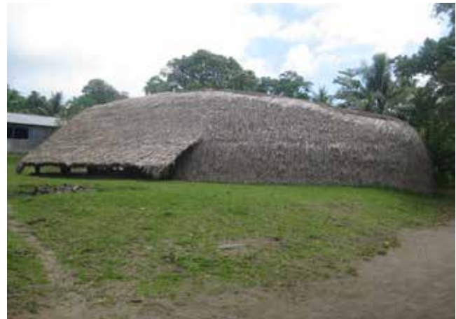
Figure 9: View of the Taloa Farea showing the recently incorporated side opening (pre- Tropical Cyclone Pam).
