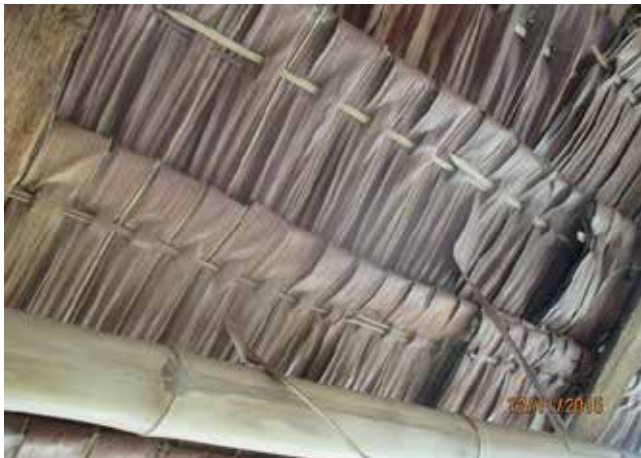
Figure 13: The natangura thatching as seen from inside (post- Tropical Cyclone Pam).
