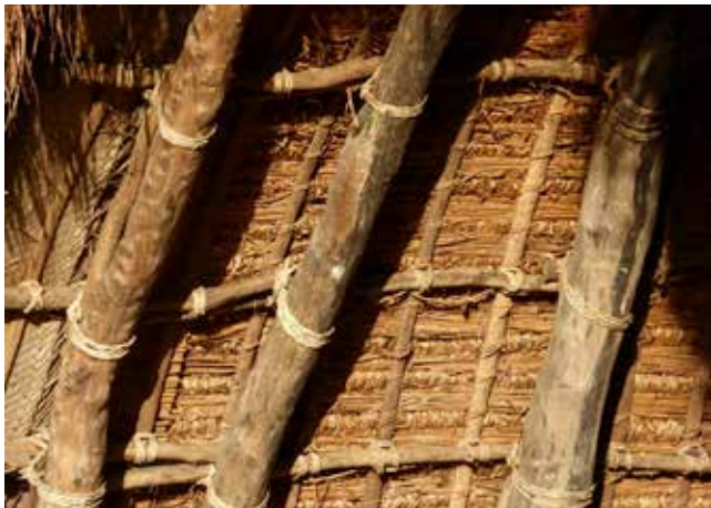
Figure 13: The interior wall texture made up of a layering of locally sourced materials (pre- Tropical Cyclone Pam).
