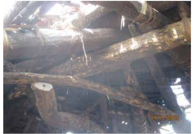
Figure 12: Sunlight streams through the holes in the natangura thatched roof post- Tropical Cyclone Pam. Without protection from the rain, the timber structural members are likely to deteriorate.
