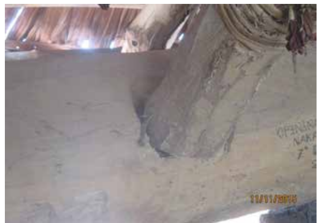
Figure 15: Rafter/beam connection detail (post- Tropical Cyclone Pam).
