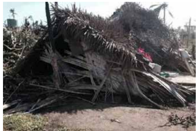
Figure 26: A house constructed from traditional materials in Tanna that was completely destroyed by Tropical Cyclone Pam.
