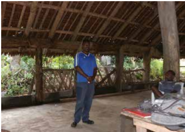
Figure 7: The interior and roof structure of the Mangarisu Nakamal (pre- Tropical Cyclone Pam).
