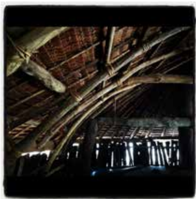
Figure 2: The interior of Nikaura Nakamal prior to Tropical Cyclone Pam.
