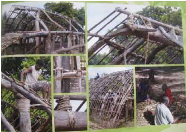
Figure 7: Photographs from 2010 showing the community rebuilding the farea.
