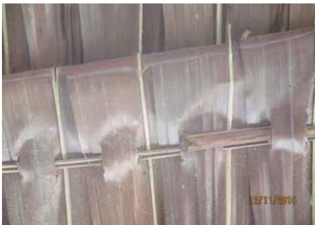
Figure 14: Natangura thatch detail (post- Tropical Cyclone Pam).
