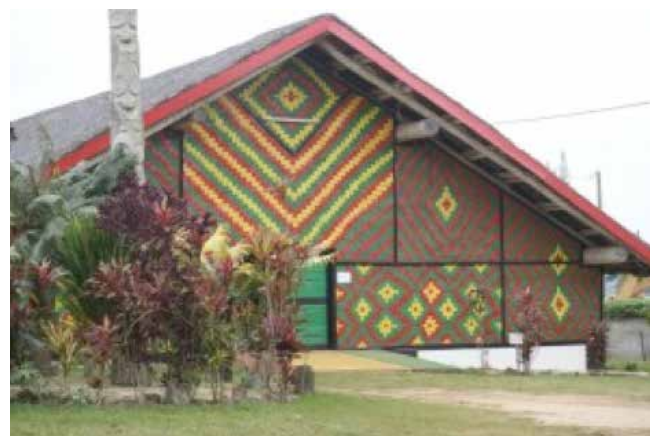
Figure 4: Exterior of the Chiefs' Nakamal prior to Tropical Cyclone Pam. Note the colourful painted split bamboo thatching to the front gable end wall.
