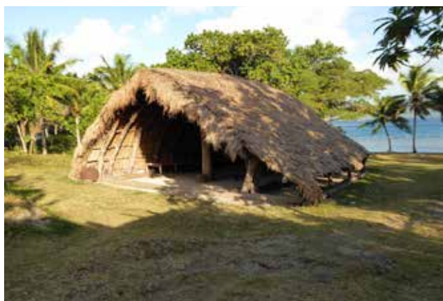
Figure 2: The form of the Taloa Farea with the main entrance facing away from the sea (pre- Tropical Cyclone Pam).
