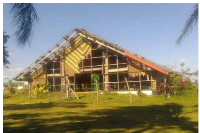
Figure 16: The front gable of the Chiefs' Nakamal was significantly damaged during Tropical Cyclone Pam.
