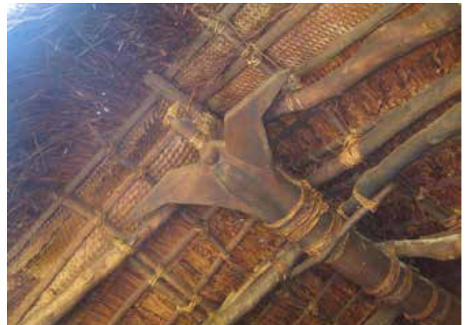
Figure 15: The carved ridge beam in the form of a pigeon at the front entry of the farea (pre- Tropical Cyclone Pam).
