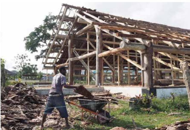
Figure 35: The primary structural members are being reused in the rebuild.
