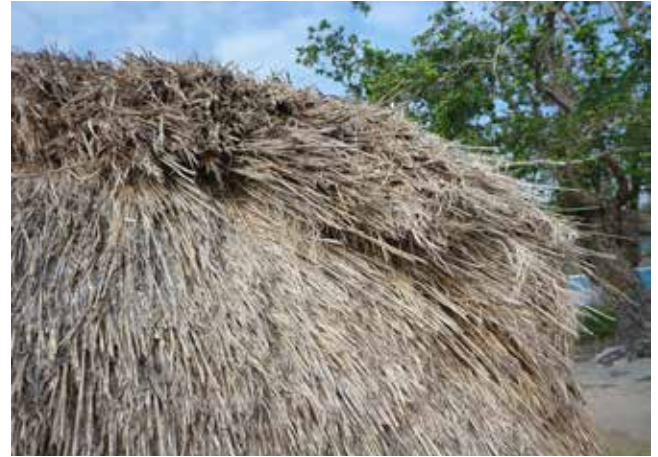
Figure 24: The wild cane fared quite well during Tropical Cyclone Pam and only appears to have been ruffled.
