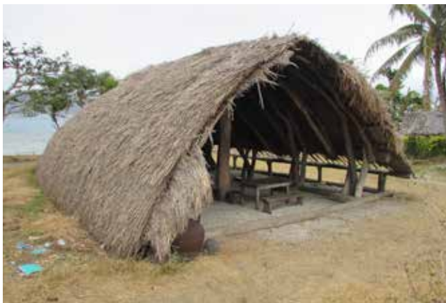
Figure 18: Front entry of the Taloa Farea on Nguna Island, post-Tropical Cyclone Pam. Despite some damage made to the natangura thatch, the farea remains in reasonable condition.
