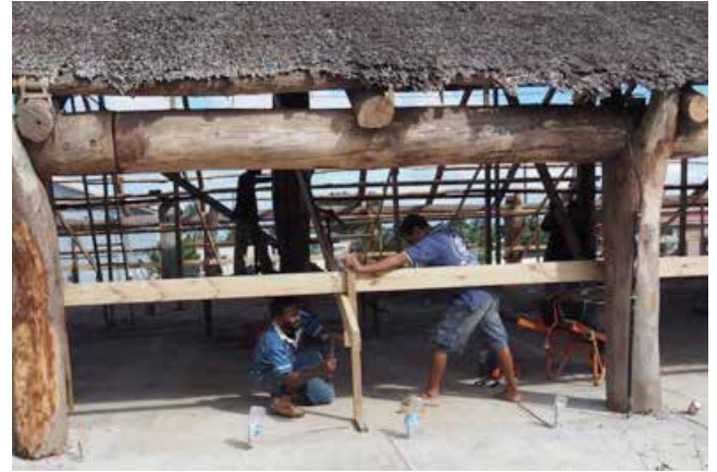
Figure 37: Note the scaffolding system being used during the reconstruction.
