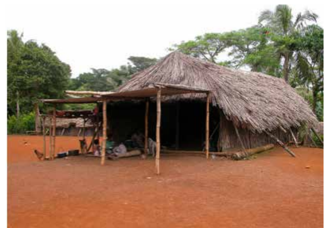
Figure 4: The exterior of the Erromango Nakamal (pre-Tropical Cyclone Pam). At this time a tin lean-to roof structure sheltered the entry to the nakamal.
