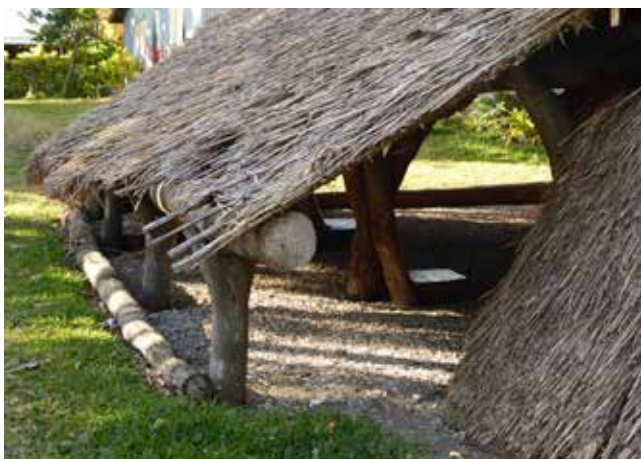
Figure 11: The low side entry to the Taloa Farea. Note that even prior to Tropical Cyclone Pam, there was already damage to the wild cane over the side eaves.
