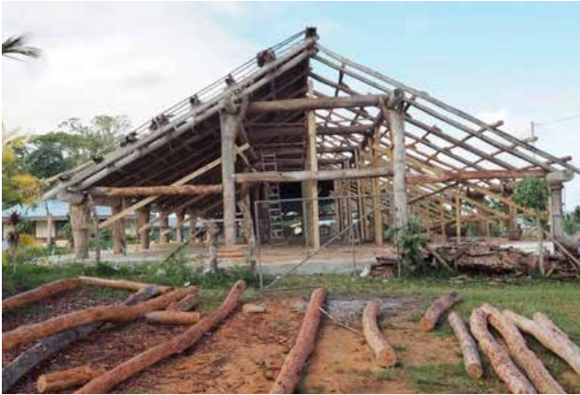
Figure 34: The Chiefs' Nakamal being reconstructed in July 2016.
