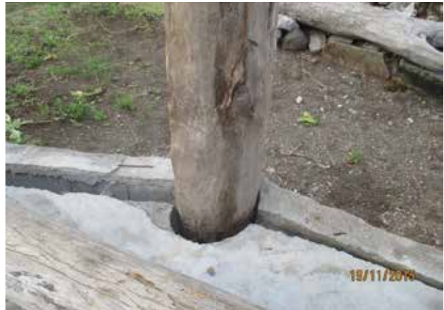
Figure 20: Post/slab edge detail (post-Tropical Cyclone Pam).
