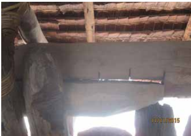
Figure 12: Beam connection detail (post- Tropical Cyclone Pam).
