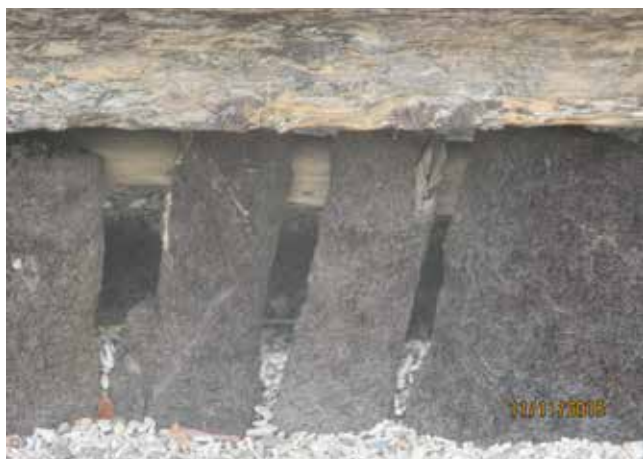
Figure 16: Detail of the black palms at the base of the walls of the Nikaura Nakamal (post- Tropical Cyclone Pam).
