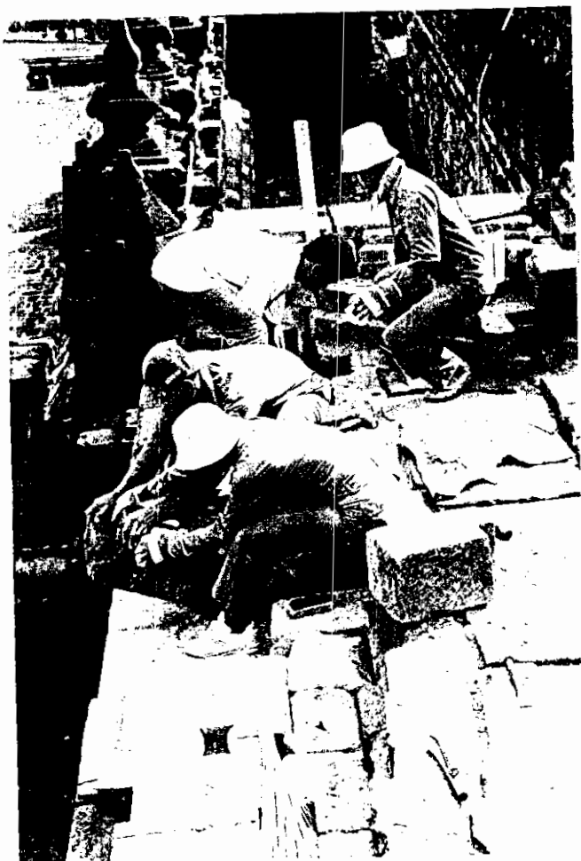
APPENDIX 15. Replacing Wall Stone of Borobudur Temple
