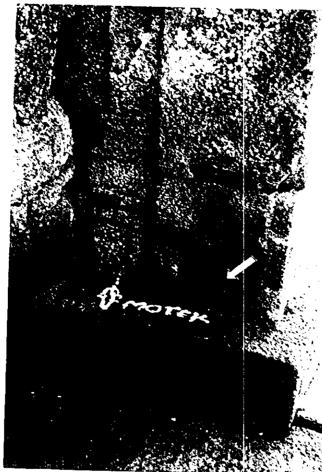
APPENDIX18. Visitors Vandalism by Graffiti on the Stone Surface
