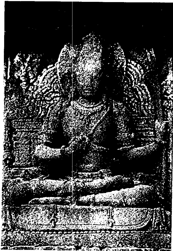
13. Detail of deterioration on the Lokapala relief at Siwa Temple on north-west side, panel XV
