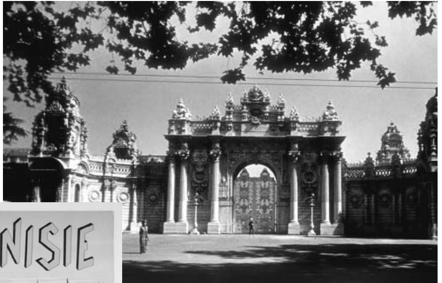
Plate 187 Main entrance gate of Istanbul's Dolmabahçe Palace, designed by Armenian architect Garabed Balyan in the 1850s. The neo-classical ensemble overlooking the Bosphorus served as the administrative centre for the Ottoman Empire from 1856 to 1923. © J.Pascal Sébaébah
