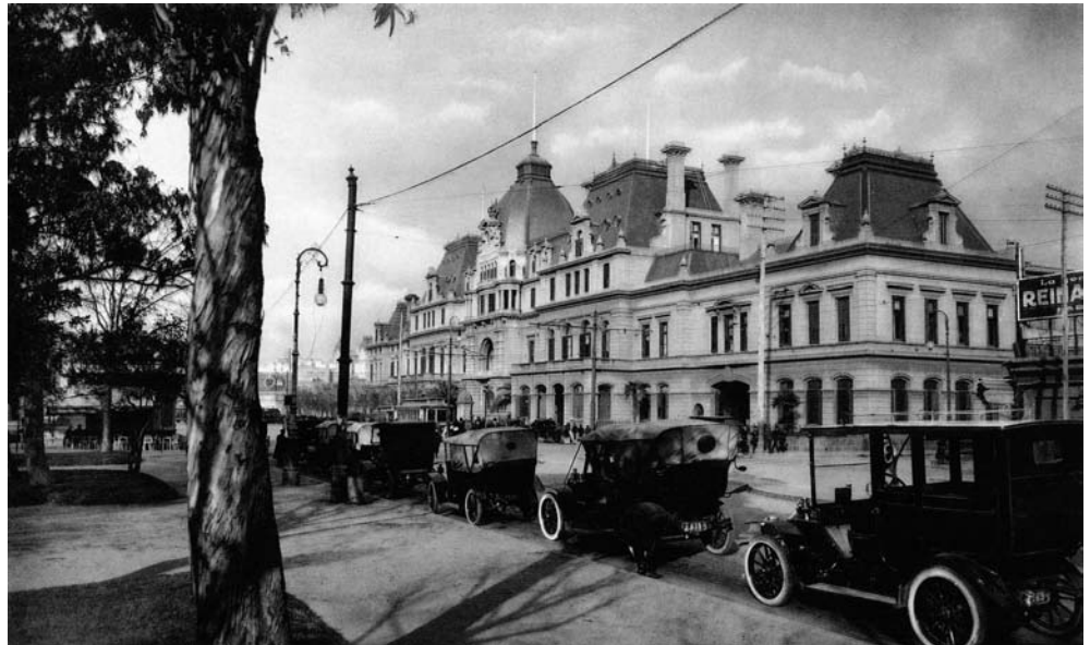
Plate 172 Estación Constitución in Buenos Aires inspired by French Second Empire architecture. © Hulton-Deutsch Collection/Corbis/Cover
