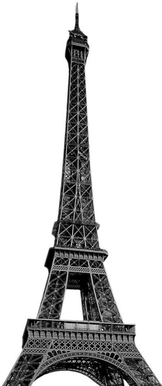
Plate 36 The Eiffel Tower (1887–89) with its innovative puddle iron framework shocked many contemporaries but eventually became Paris's pre-eminent landmark. DeA Picture Library
