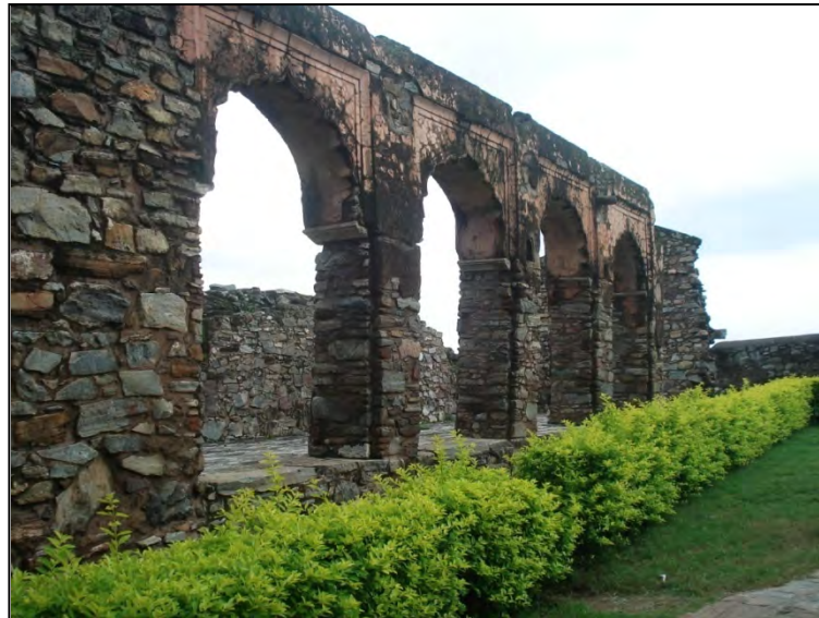
Simple arcaded structure built in Kumbha's time seems to have been renovated in 20 th century as lime stucco remains show-built in rubble stone laid in lime mortar
