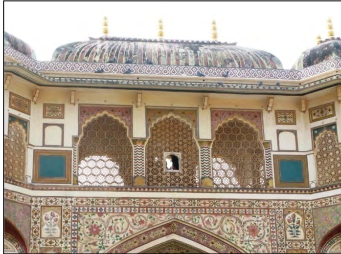
Cusped arches with intricate jalis on the upper floor of Ganesh Pol
