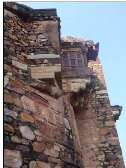
Random rubble masonry wall with jharokas
