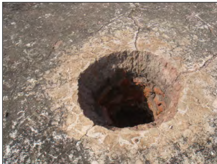
An opening to the store house to fill the grains from top
