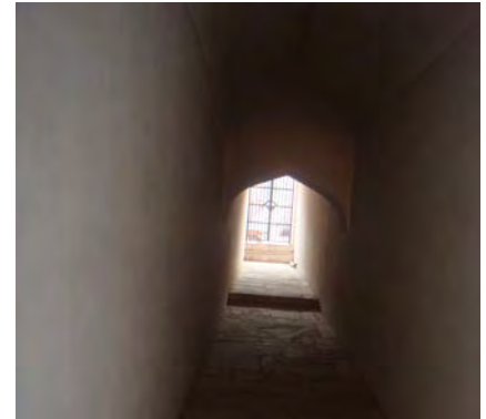
Internal View of tunnel at Amber Source: Dronah
