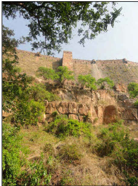
Fortification as viewed from Shiv Temple area
