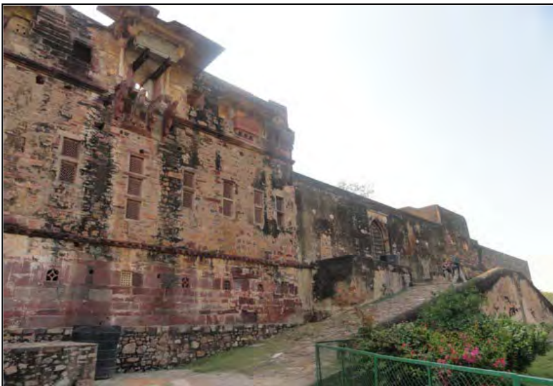
Stone brackets and jais on the façade of Hammir Mahal
