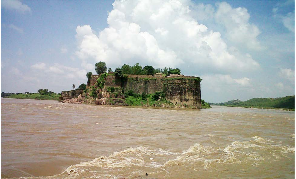
View of Gagron from the rear showing the fort structure as it stands on the solid rock with a double fortification layer seen at a higher level
