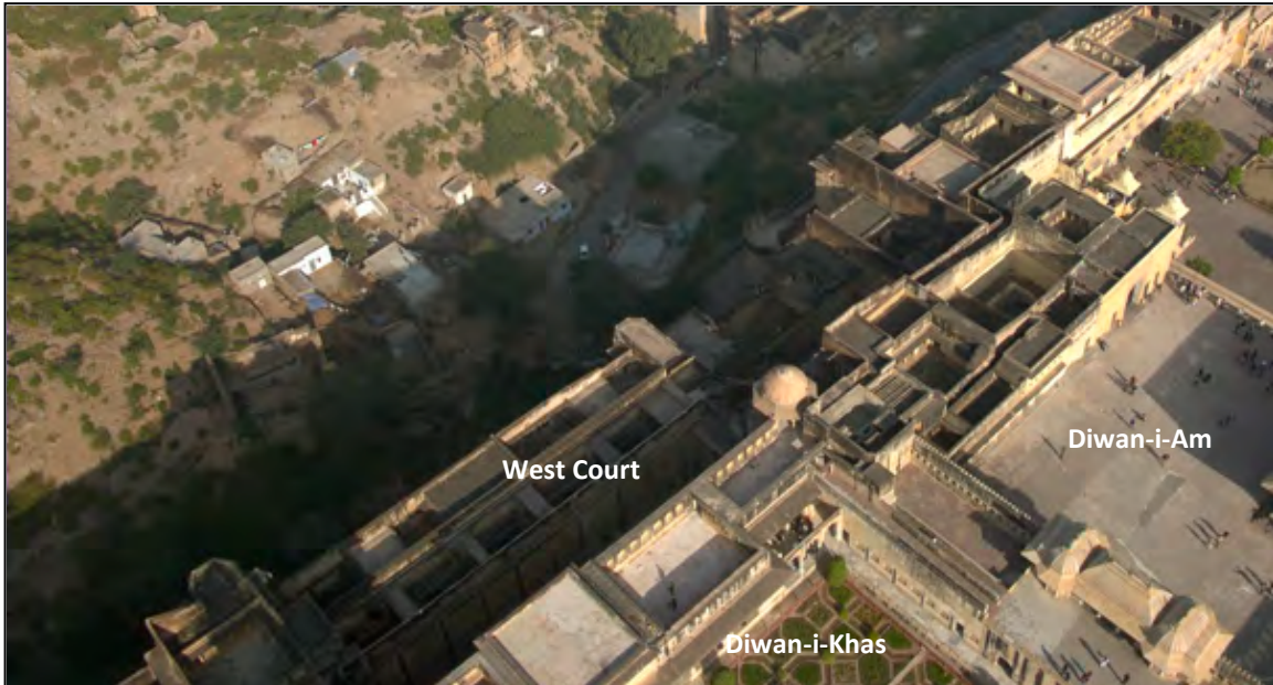
Area covered under west courts showing the character of the spaces with small courtyards, verandahs and several rooms
