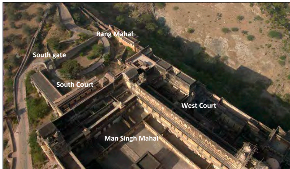
An aerial view of the courtyard at South Court with service spaces around Source: State Department of Archaeology -Rajasthan
