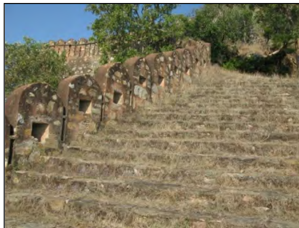
Inner view of the fort wall showing the merlons
