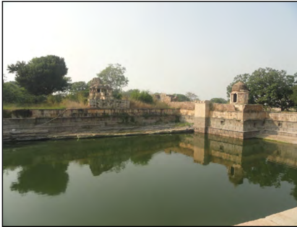
Embankments in stone with a shrine – Bhimlat tank
