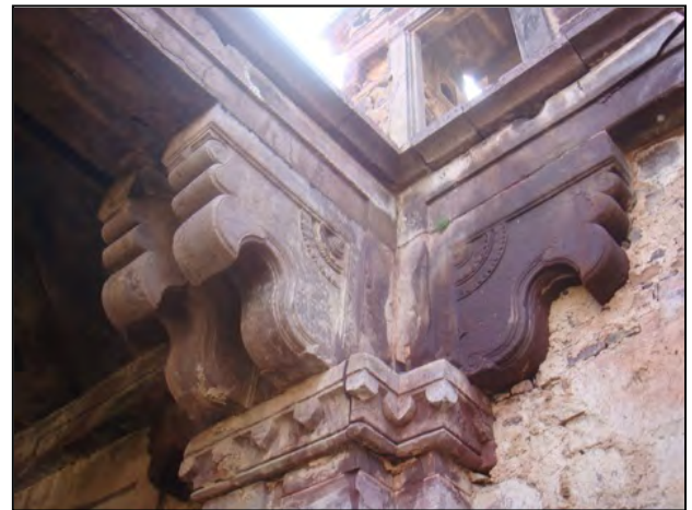
Brackets carved in sandstone supporting beams
