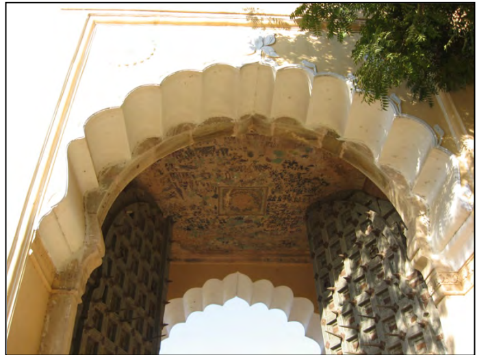
Cusped archway of Suraj Pol with metal spikes on the wooden gate
