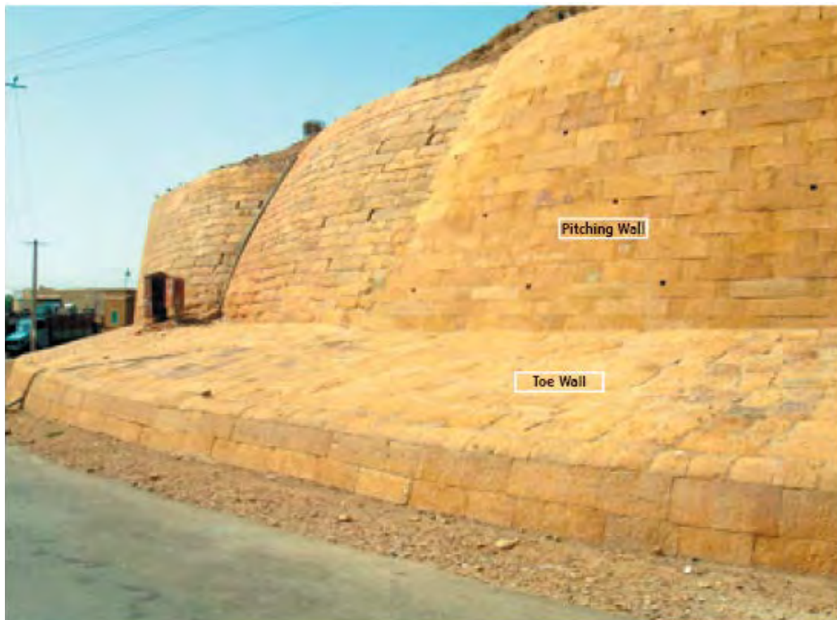
View of the pitching and Toe wall, Source: World Monuments Fund
