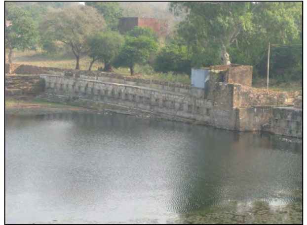
Embankment in stone along Chatrang ka Talab
