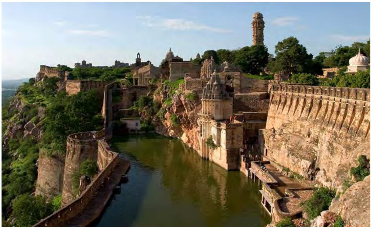
View of Chittorgarh fort. Source: DRONAH
