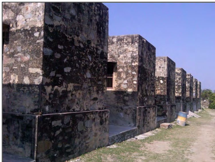
Barracks in plain stone masonry structure laid in lime mortar with no ornamentation
