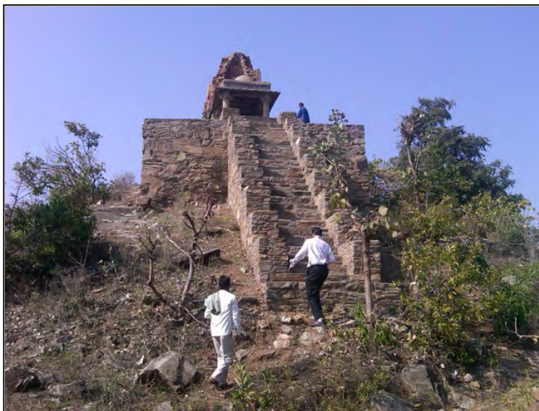
The temple raised on a high plinth
