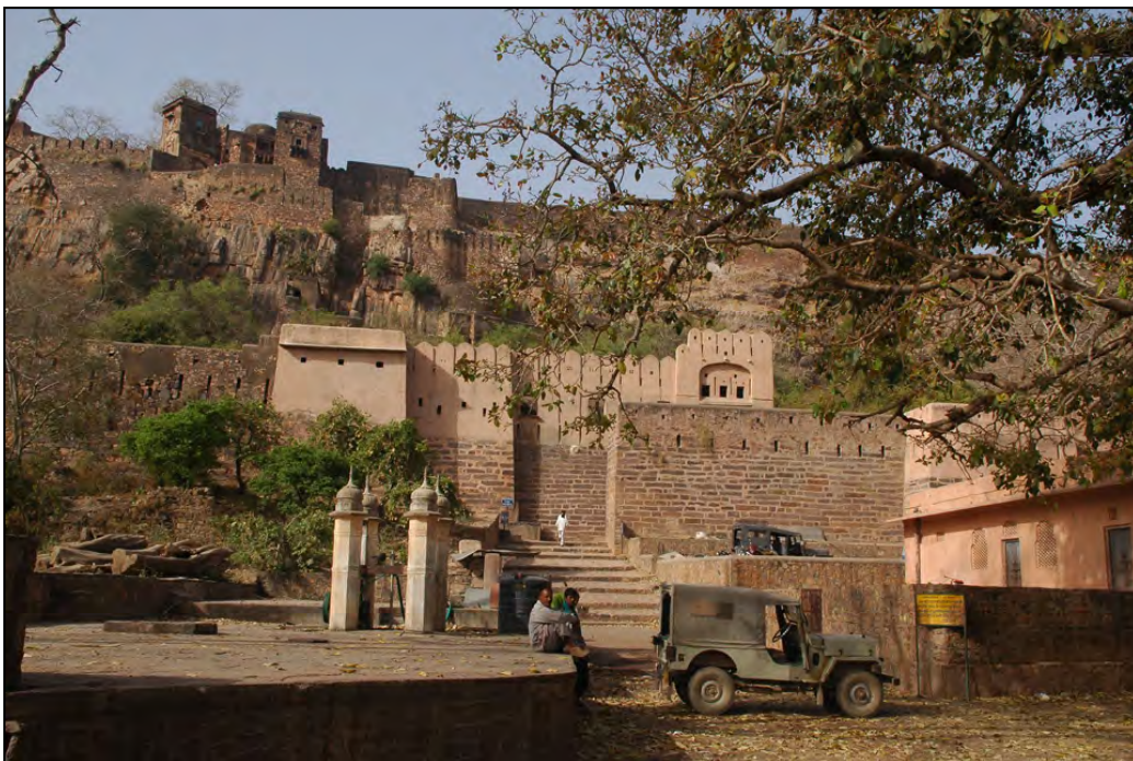
The entrance to the fort from Naulakha Pol and the fort at the higher level reached by steps and ramps following a zig zag pattern; all laid down as part of security measures in synchrony with the terrain
