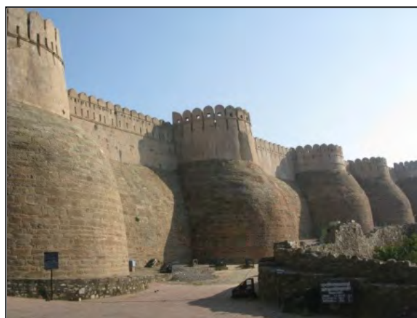
The D shaped bastions almost as high as the walls with a single storey, have a strong talus that is nearly vertical along most of its lower part and then abruptly comes to an end. This form of talus prevented the tower from being taken by escalade (Nossov, 2006, 19)
