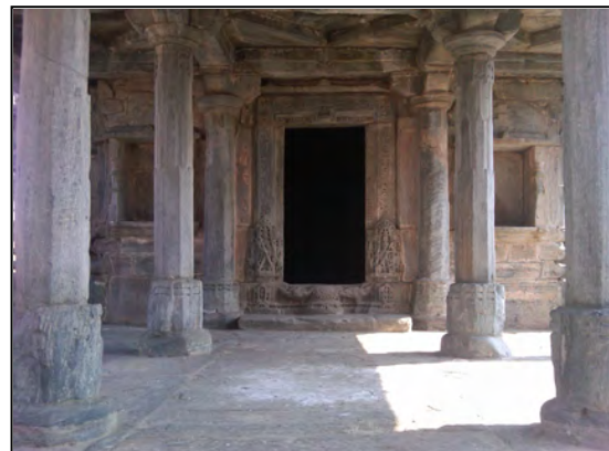
Trabeate system of spanning the temple roofs
