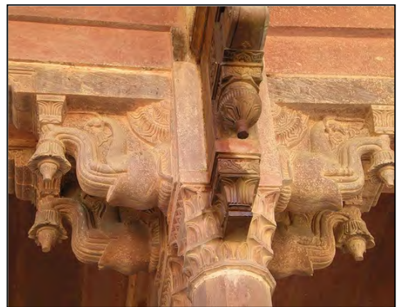
The sandstone carved brackets supporting the trabeate system of spanning spaces
