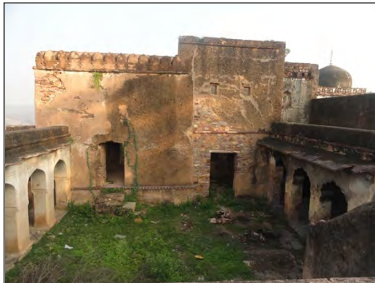
Verandah with cusped arches in stone - Badal Mahal
