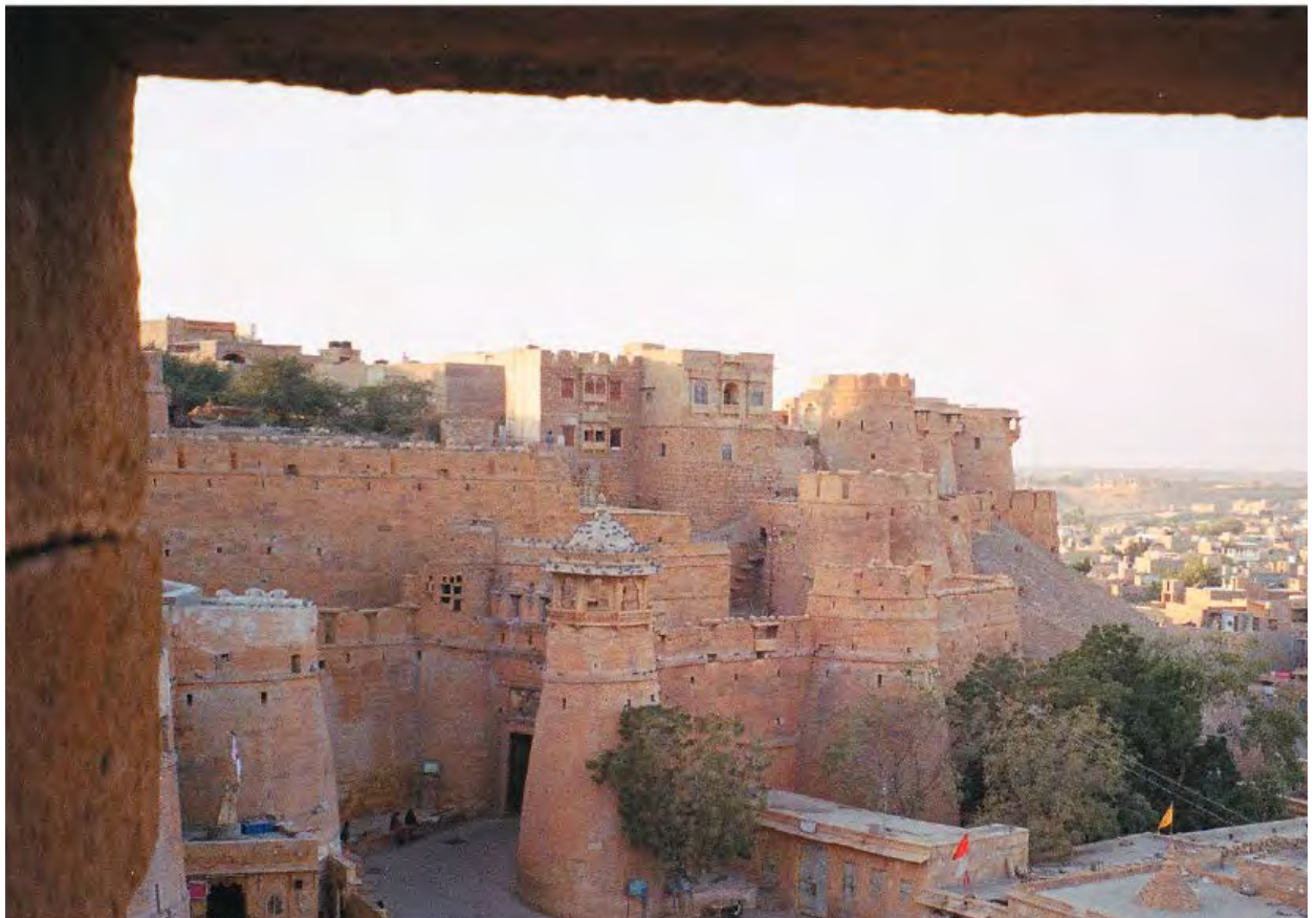
Gunports covering the main entrance gateways
