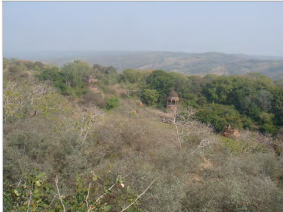
Ruined Chattris amidst dense vegetation - these are found dispersed all over the site and require detailed mapping. Smaller chhatris were usually built in memories of young Princes who died at an early stage
