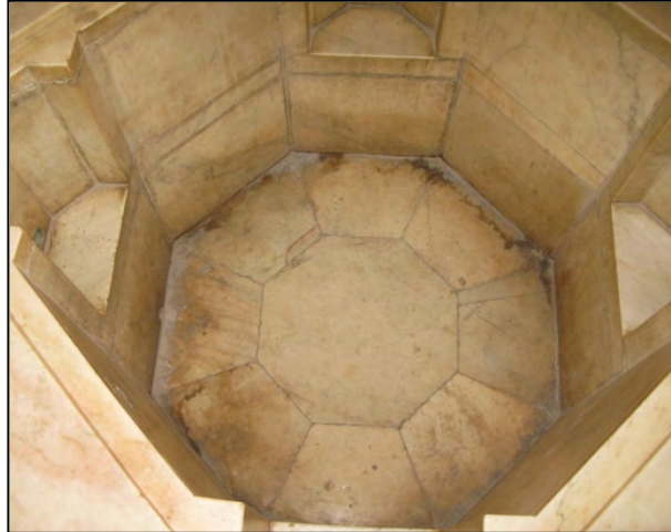
Hammam between the Diwan-i-Am and Diwan-i-Khas with water outlets at four corners
