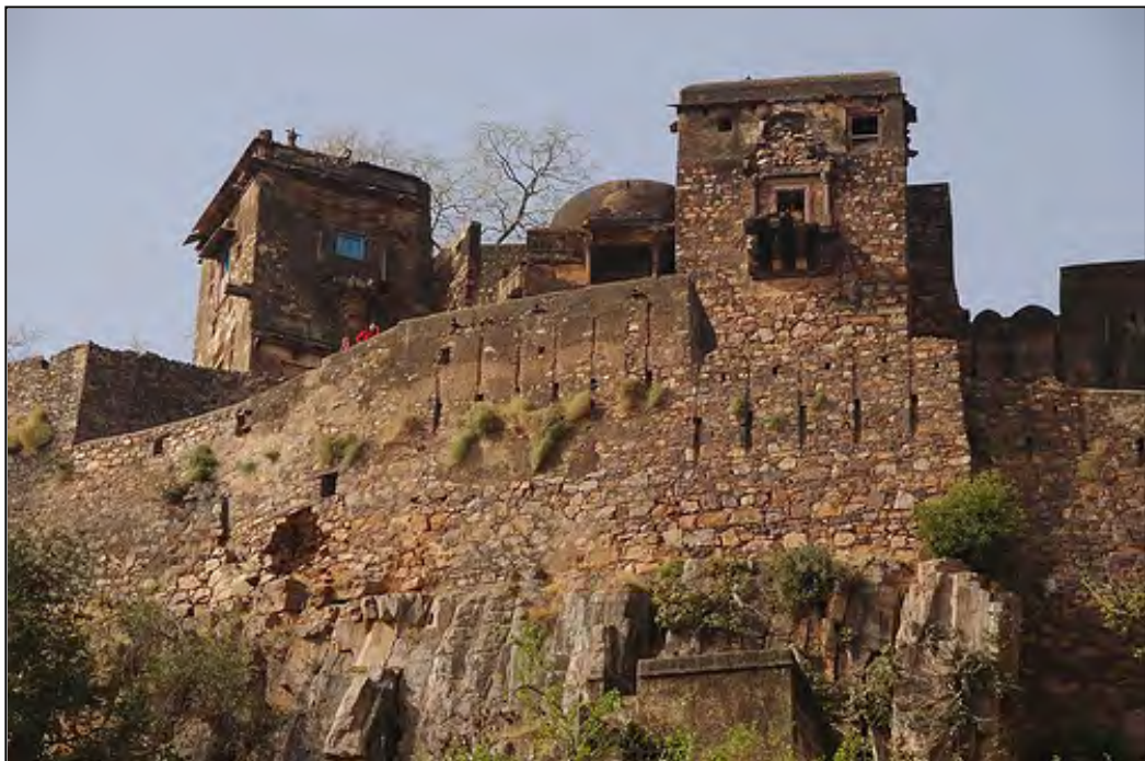
View of the fortification varying in heights with the narrow embrasures for firing
