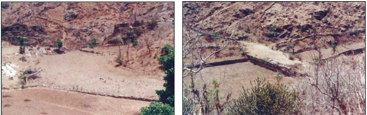
Talabs and dams near Juna Bhilwara village Source: Dorje and Dimri, 2008
