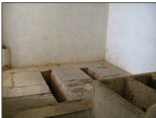
Toilets at Man Singh Mahal that open to South Court
