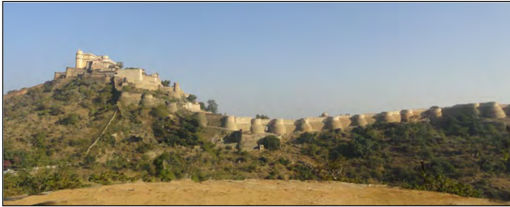
View of the fortification and bastions following the natural contours of the hill
