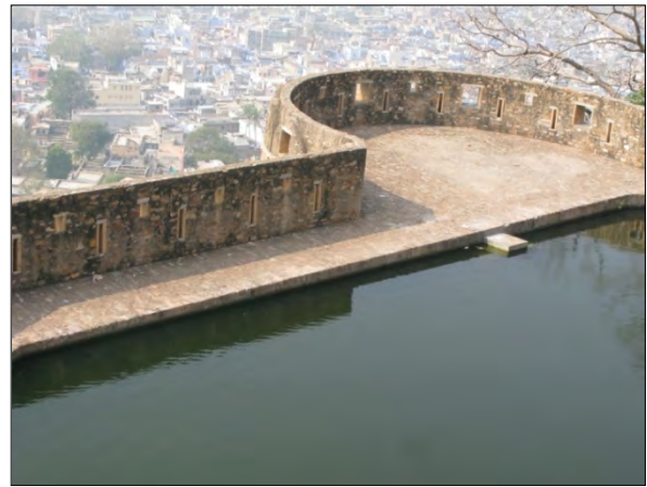
View of the Gaumukh kund along the edge of fortification wall
