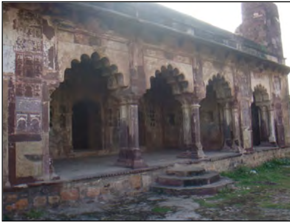
Cusped arches in sandstone – Chhoti Kachehri
