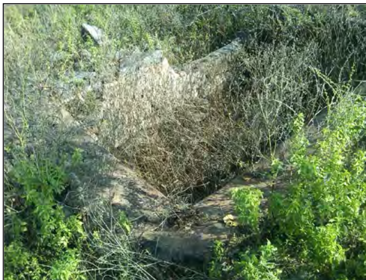
Remains of a traditional lime mortar grinding set-up: structures like these lie scattered amidst the wild vegetation of the fort and require detailed mapping
