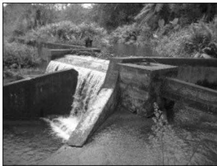
Figure 15.3 Water intake, Rio Barbas, Colombia
