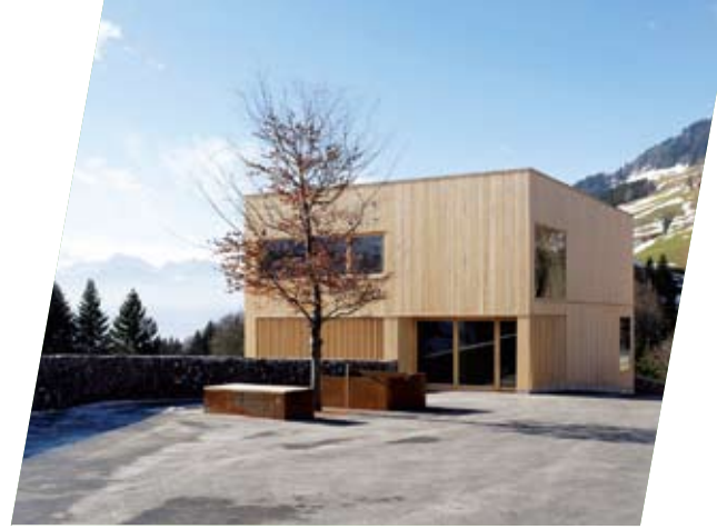
The municipal office of St. Gerold in Großes Walsertal BR was constructed as a 'passive house' (© BR Management).
