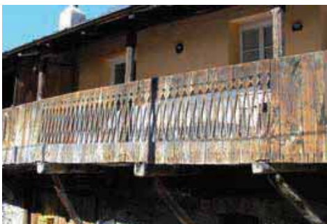
Typical balcony in the Puente neighbourhood Jorge F. Layna
