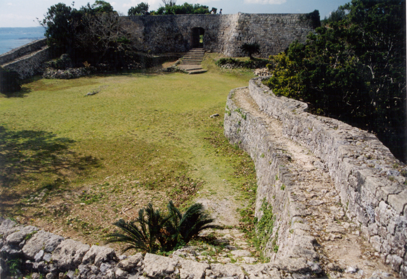
2-D-16 Nakagusuku-jô site. Arched gate and castle walls of second enclosure. S
