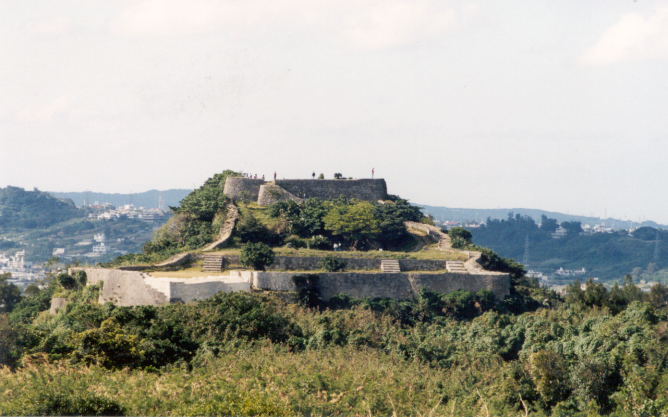
2-C-4 Katsuren-jô site. View from southeast. S
