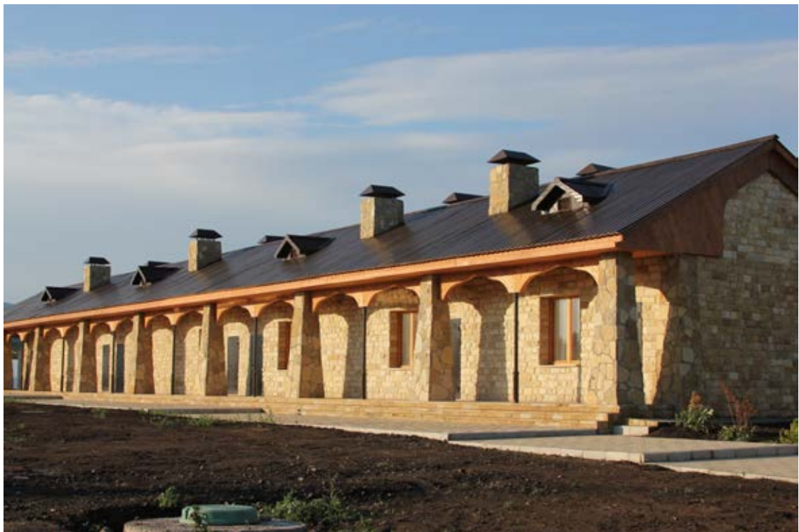
General view of Craft workshops. View from the south.
