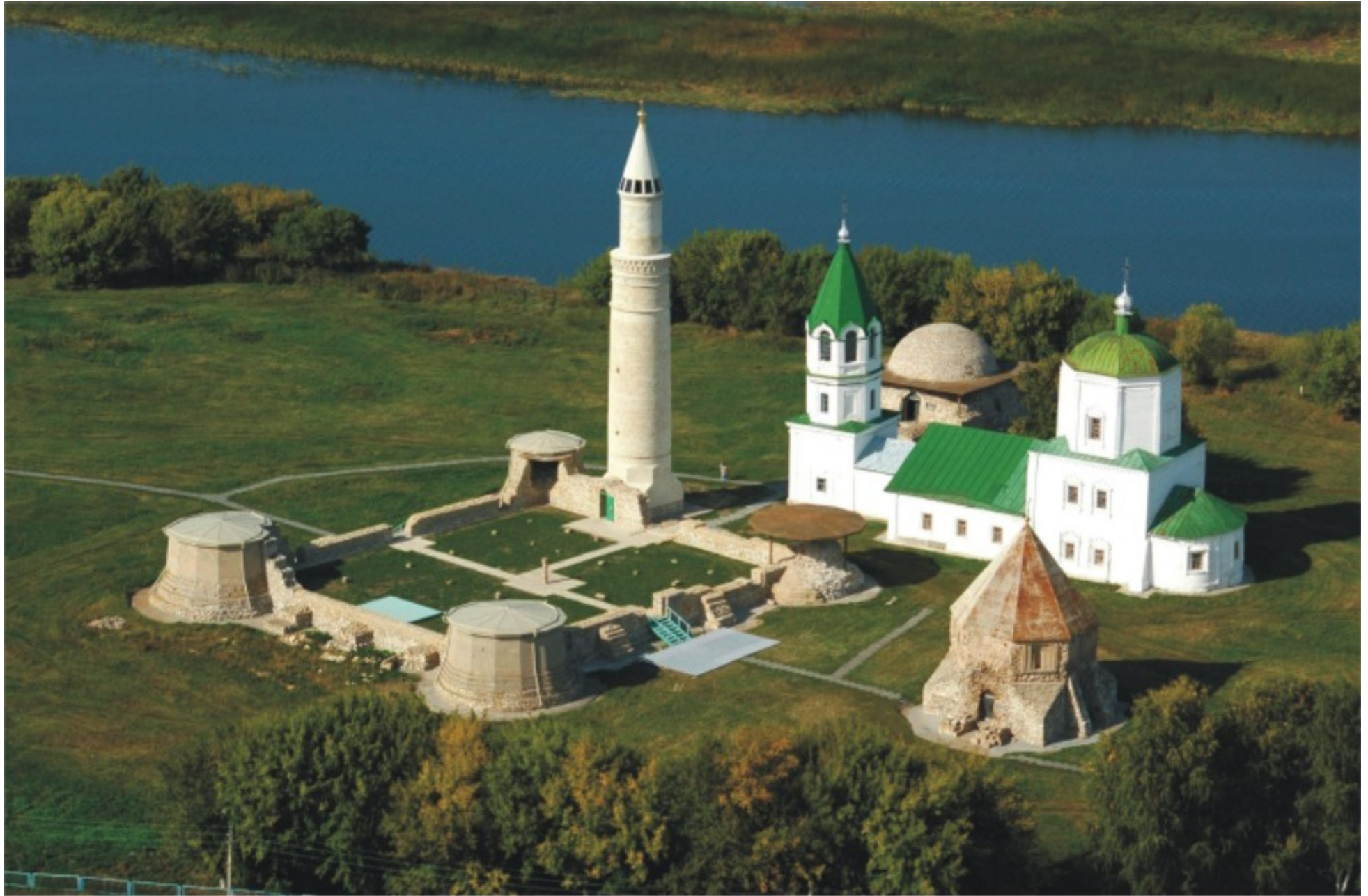
Fig.20 . View from above
