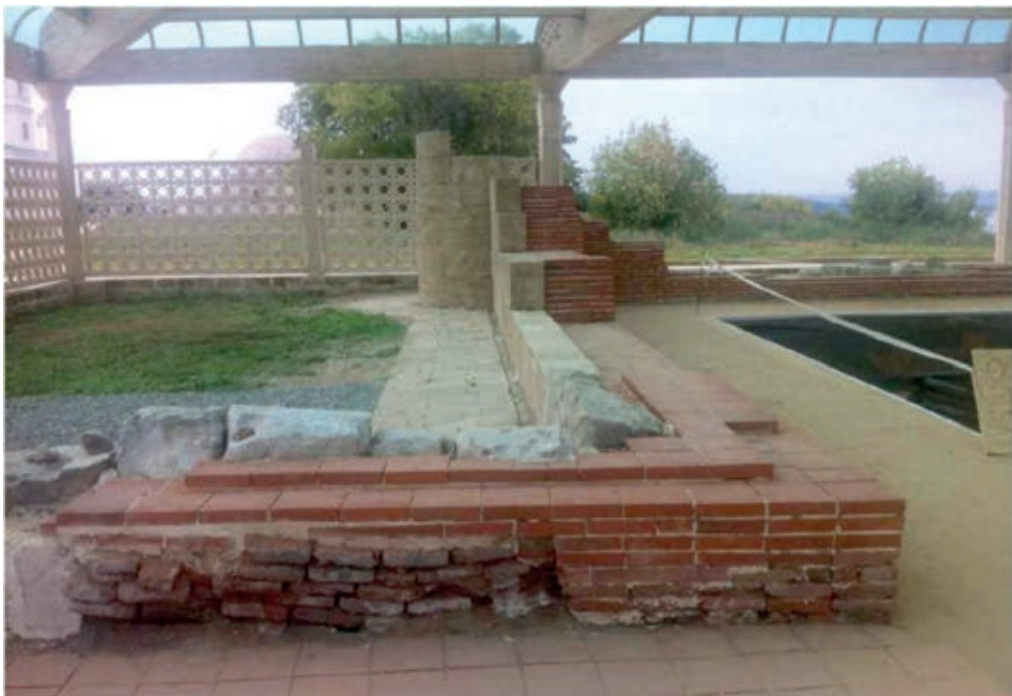
PHOTO 4: VIEW FROM INSIDE THE KHAN'S PALACE AREA. WHILE SOME ORIGINAL TILES ARE INCORPORATED, THE WALLS AND FLOORS ARE COMPLETE RECONSTRUCTIONS THAT HAVE REPLACED THE ORIGINAL CONTEXT. THIS HAS SIGNIFICANTLY REDUCED INTEGRITY AND AUTHENTICITY. THE AVERAGE VISITOR DOES, HOWEVER GAIN A GOOD UNDERSTANDING OF THE STRUCTURES THAT WERE ONCE PRESENT. HENCE, THE COVERED AREA CAN BE CONSIDERED A SITE MUSEUM.
