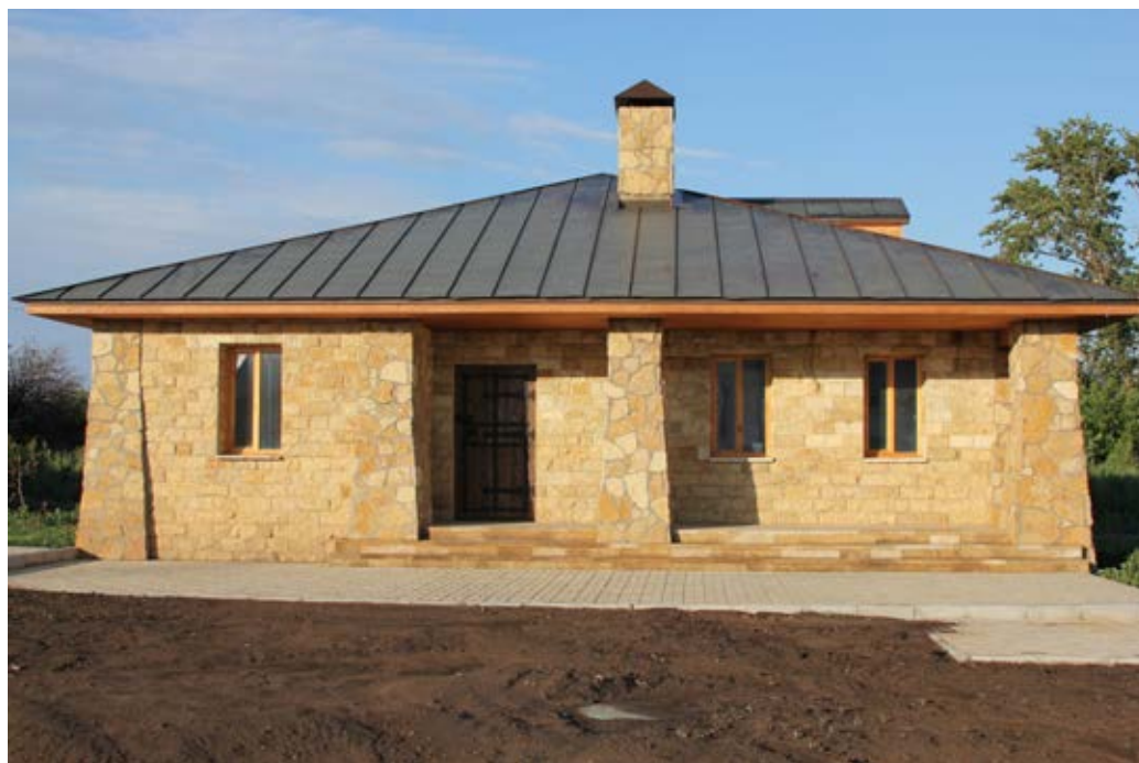
General view of “The House of a doctor”. View from the west.
