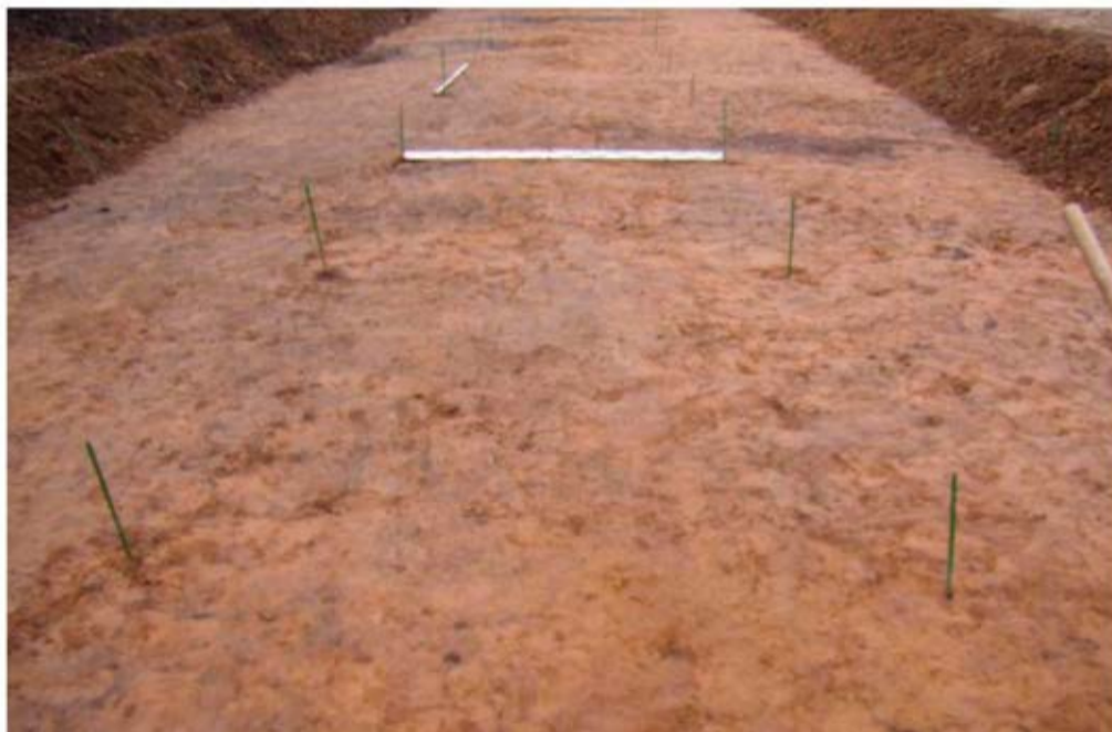
Observations during asphalt road construction on the site of historic roads
