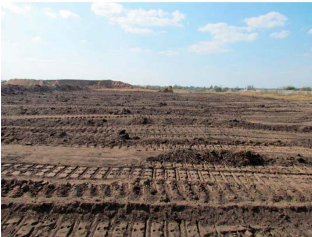
Soil cutting on the place of the oncoming car parking construction
