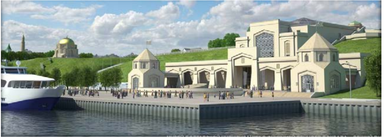
The project of the river station and the Museum of Bolgar civilization.
