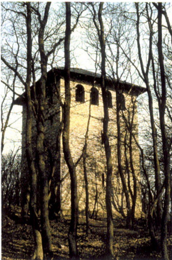
006 - Ober-Mörlen, Wetteraukreis. The reconstructed watchtower WP 4/16 on top of the Gaulskopf was built 1912 according to plans of Ernst Fabricius, secretary of the Reichs-Limeskommission. (Landesamt f. Denkmalpflege Hessen).
