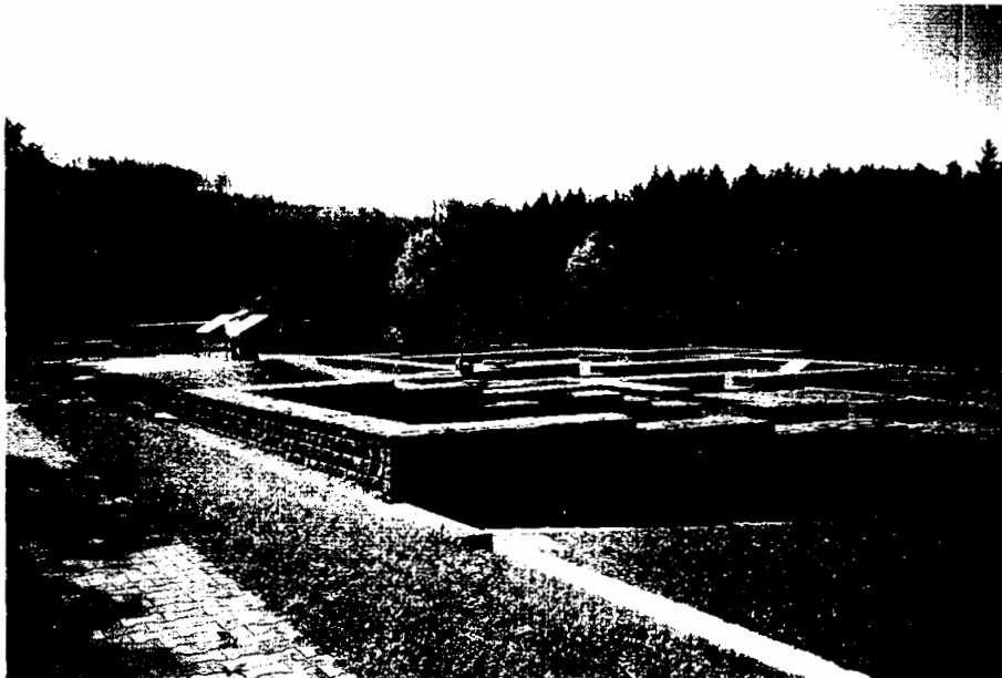
008 - Schwäbisch Gmünd, Ostalbkreis. Baths of the fort at the Schirenhof. The visible walls are modern constructions separated by layers of gravel from the ancient structures in the soil. (Landesdenkmalamt Baden-Württemberg).
