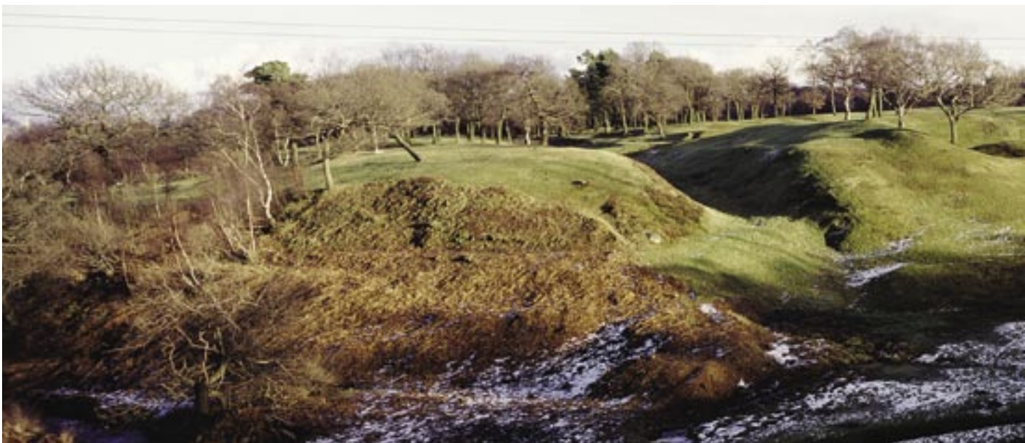
The western defences of the fort at Rough Castle seen from across the Rowan Tree Burn.
