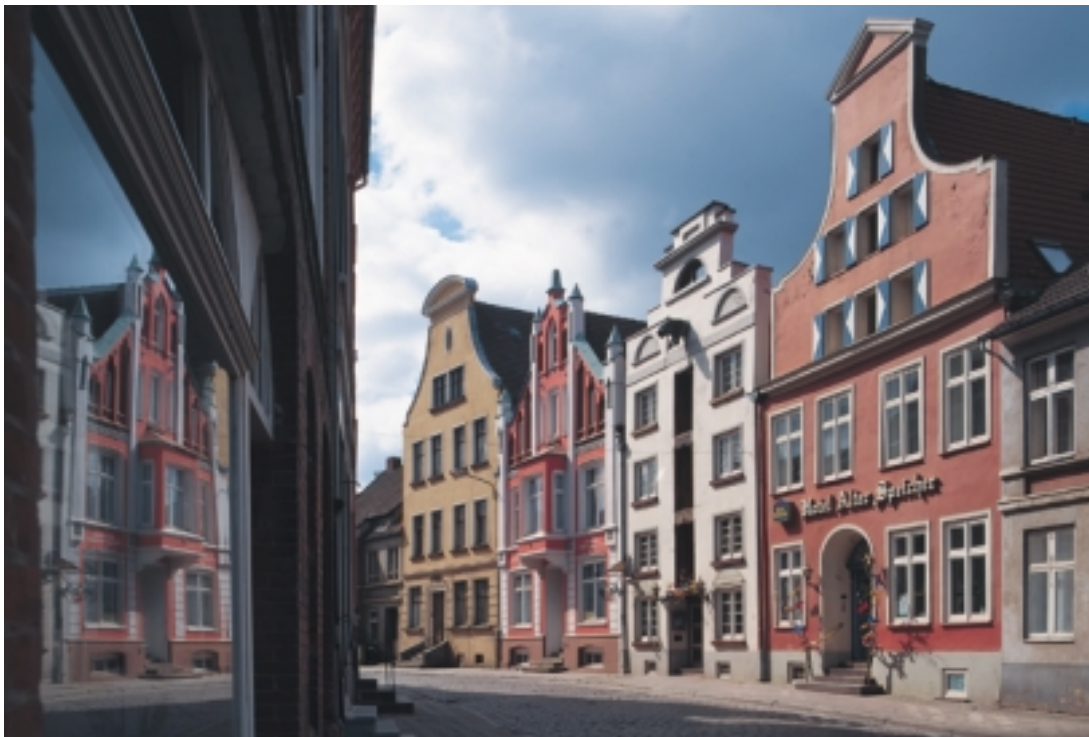
Fig. 98: Gabled house facades from different epochs in Bohrstraße in Wismar
