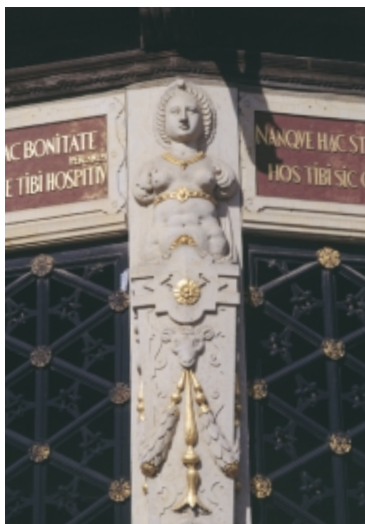
Fig. 107: Decorative herma pilaster, a detail of the Wasserkunst in Wismar
