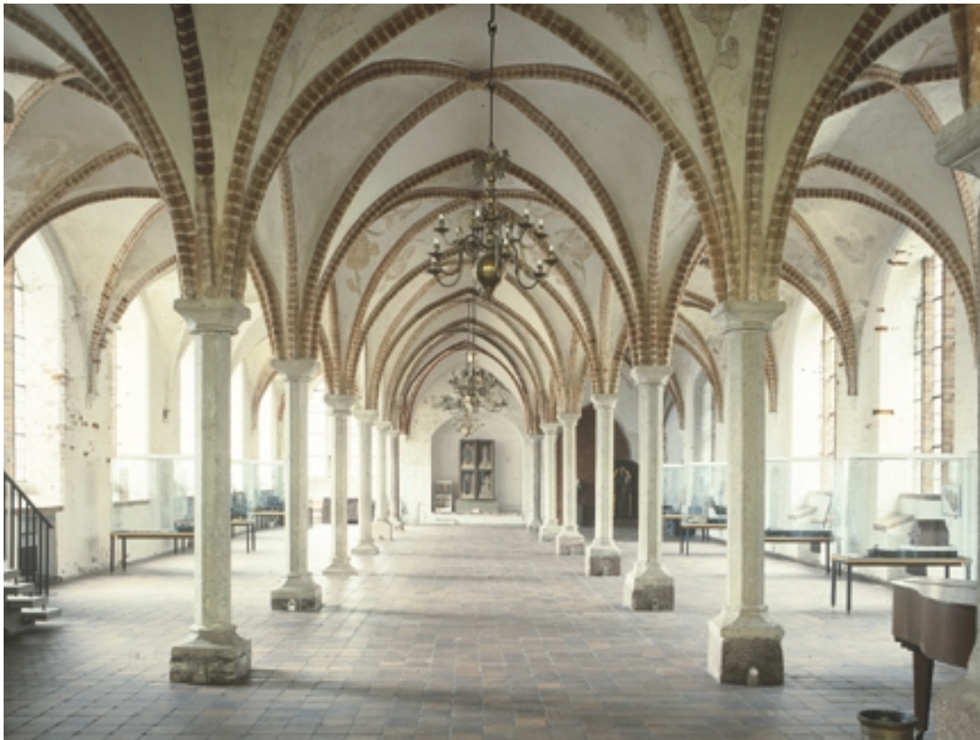
Fig. 45: The Remter or summer refectory of St. Catherine's monastery in Stralsund
