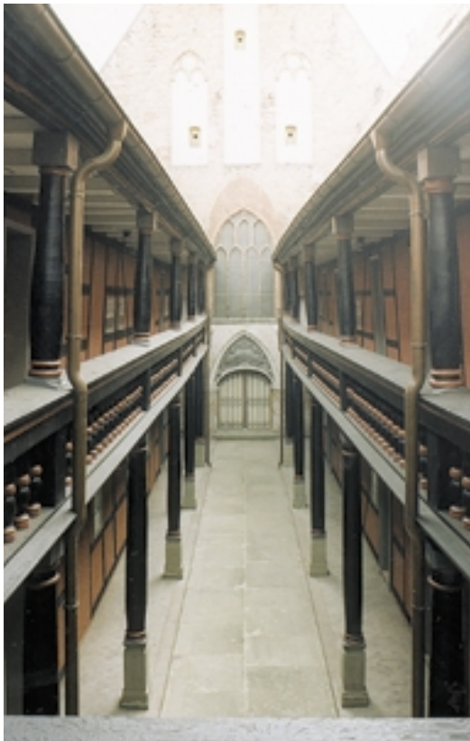
Fig. 47: The Kirchgang built onto the east wall of the Heilgeist-Kirche in Stralsund with inserted wooden gallery
