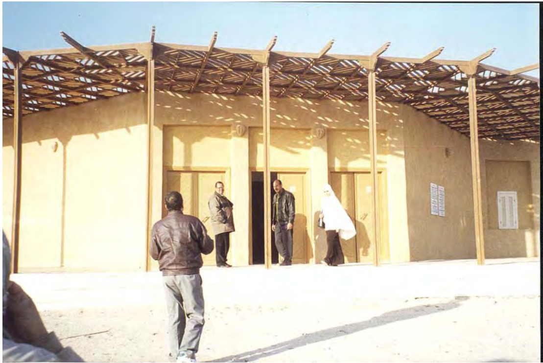
Fig. 26 – Visitor Center at WRPA, on the western shore of the Lake.
