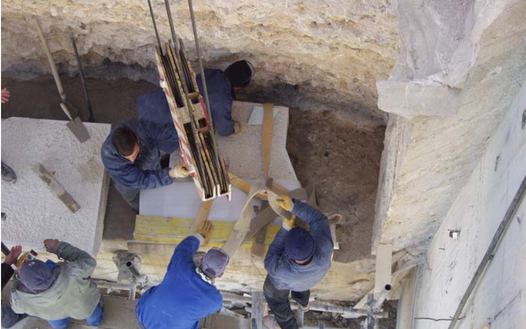
Photo 42: Masonry works (PCU Collection, 2003)
