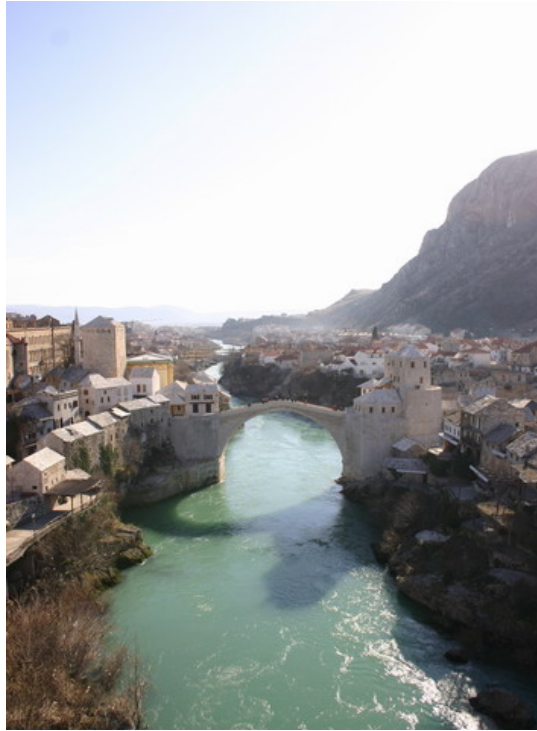
Photo 59: Old Bridge (AKTC/WMF Collection, 2004)
