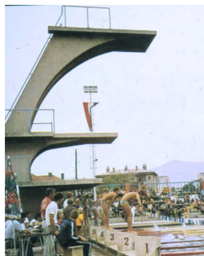
Swimming pool, constructed in 1958
