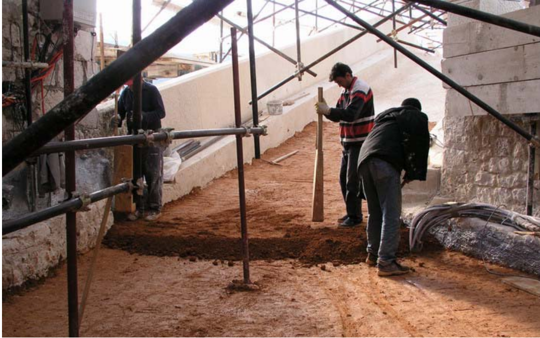
Photo 46: Terra rossa hydro - isolation (PCU Collection, 2004)
