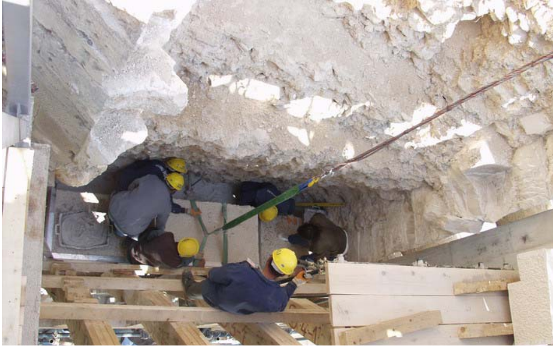
Photo 44: Masonry works (PCU Collection, 2003)
