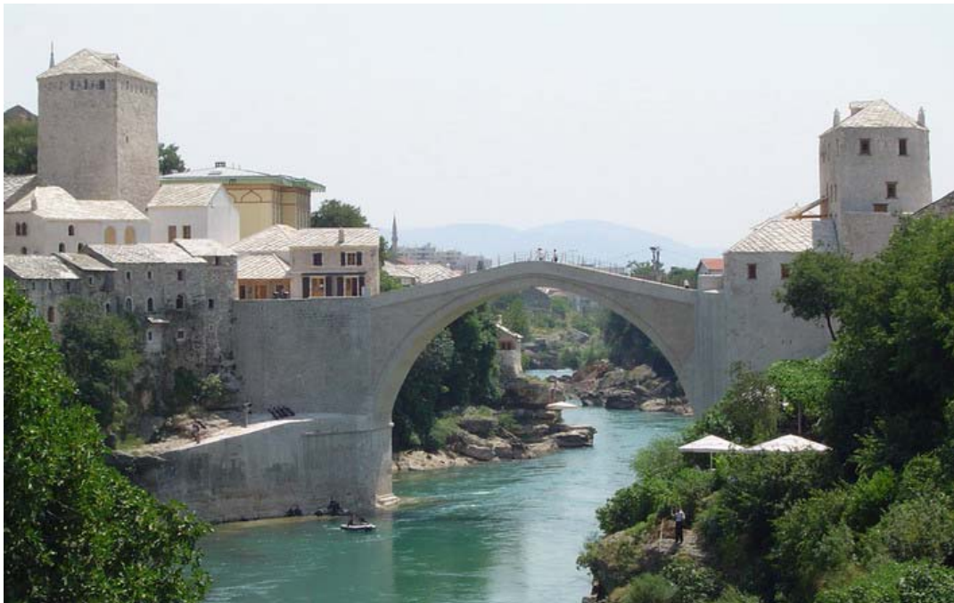
Photo 58: Old Bridge (AKTC/WMF Collection, 2004)
