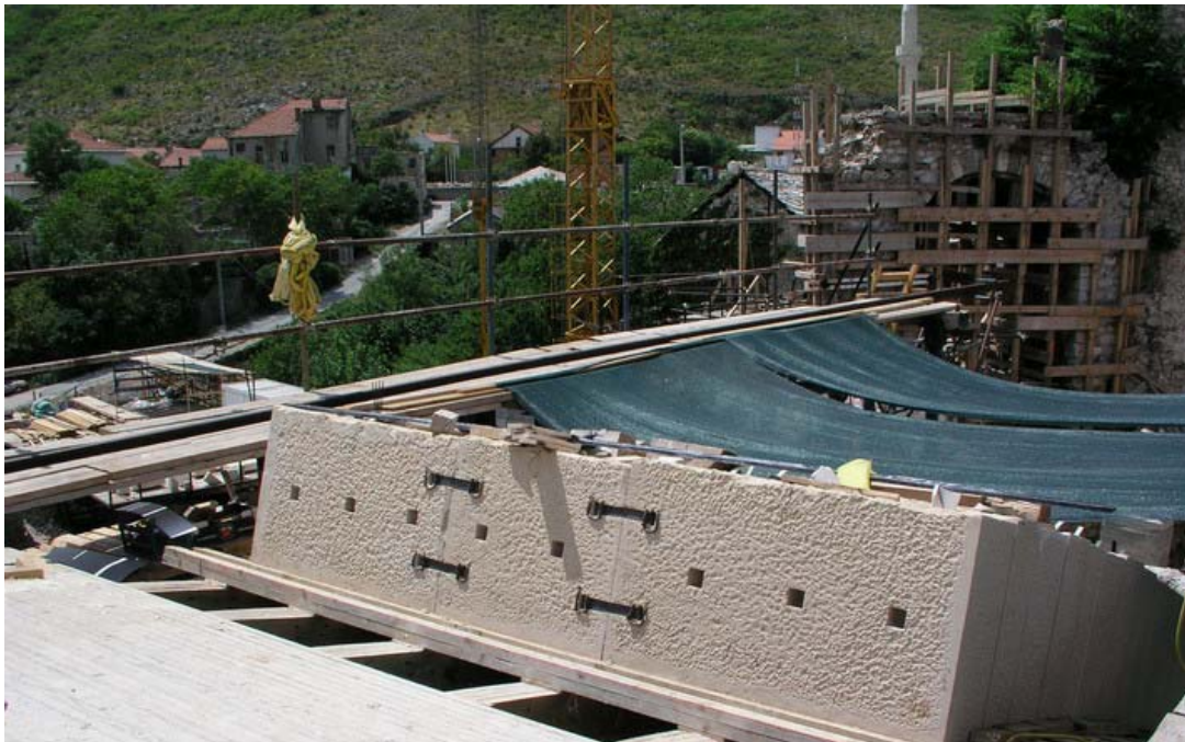
Photo 45: Masonry works - vault (PCU Collection, 2003)
