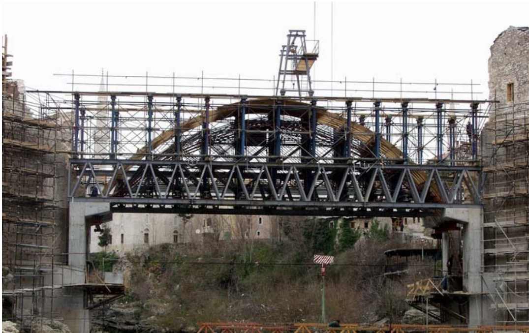
Photo 37: Scaffolding (AKTC/WMF Collection, 2002)
