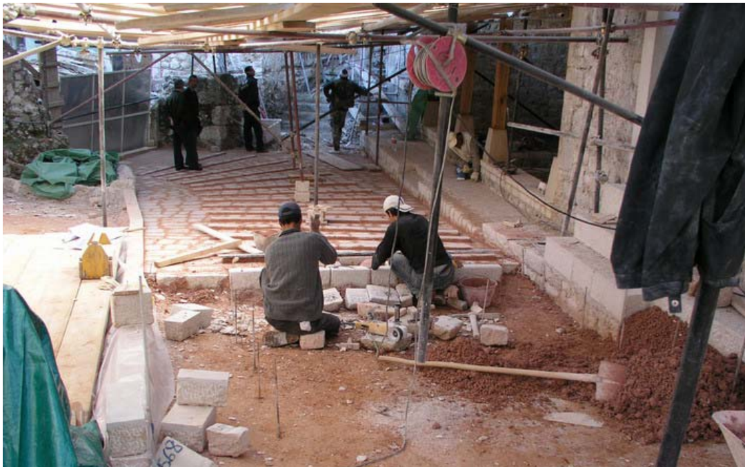
Photo 47: Bridge pavement (PCU Collection, 2004)
