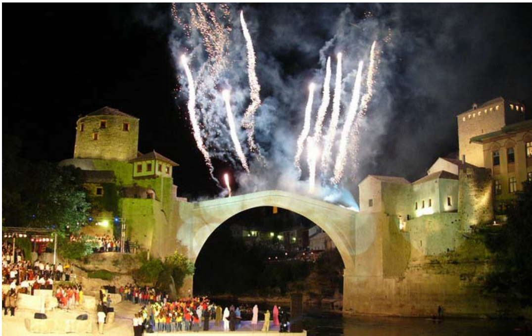
Photo 61: Mostar Old Bridge (AKTC/WMF Collection, July 23, 2004)
