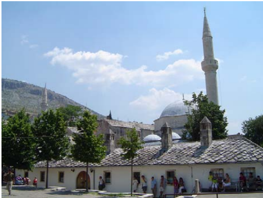
Photo 14: Koski Mehmed Paša Mosque (AKTC/WMF Collection, 2004)
