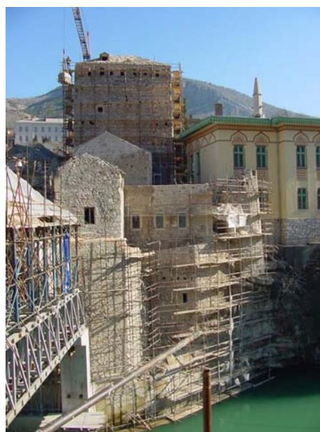
Old Bridge Complex – during restoration
