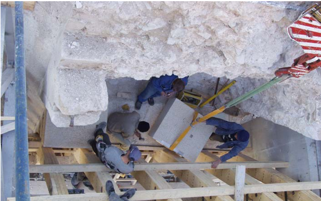
Photo 43: Masonry works (PCU Collection, 2003)
