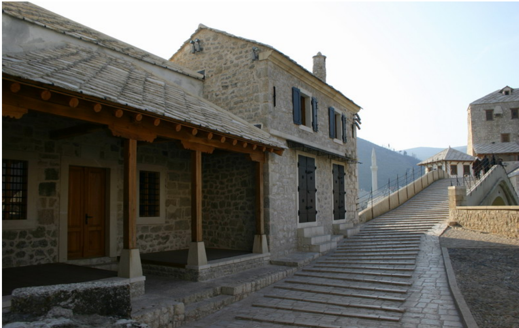
Photo 57: Old Bridge (AKTC/WMF Collection, 2004)
