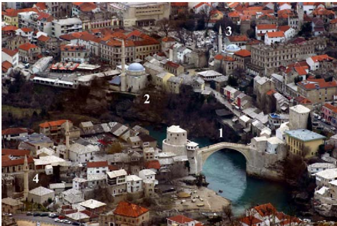
Old City of Mostar (Nominated Area): 1. Old Bridge Complex, 2. Koski Mehmed Paša Mosque, 3. Nesuh-age Vučijeković Mosque, 4. Nezir-aga Mosque
