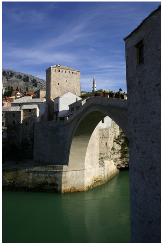
Photo 60: Old Bridge (AKTC/WMF Collection, 2004)
