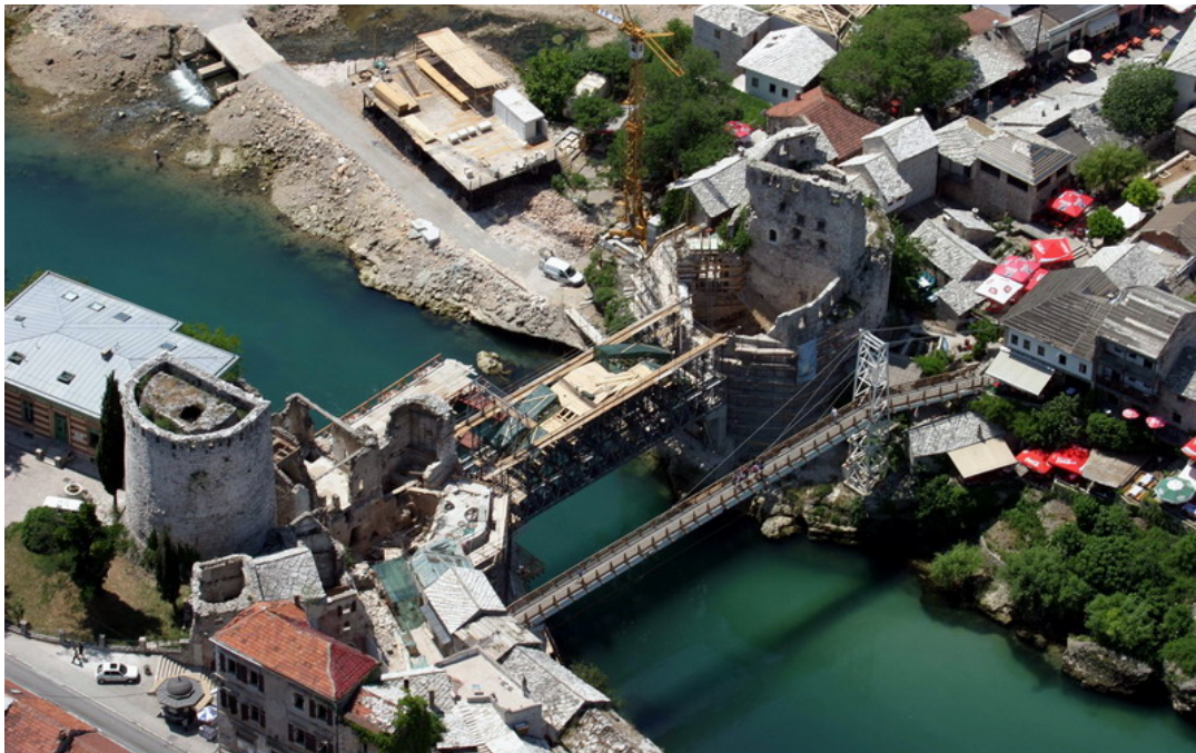
Photo 38: Scaffolding (AKTC/WMF Collection, 2002)
