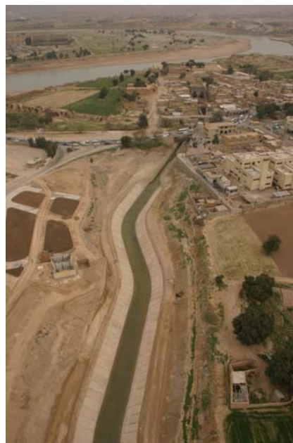
Fig. 119. The Dâriun Canal going through town
