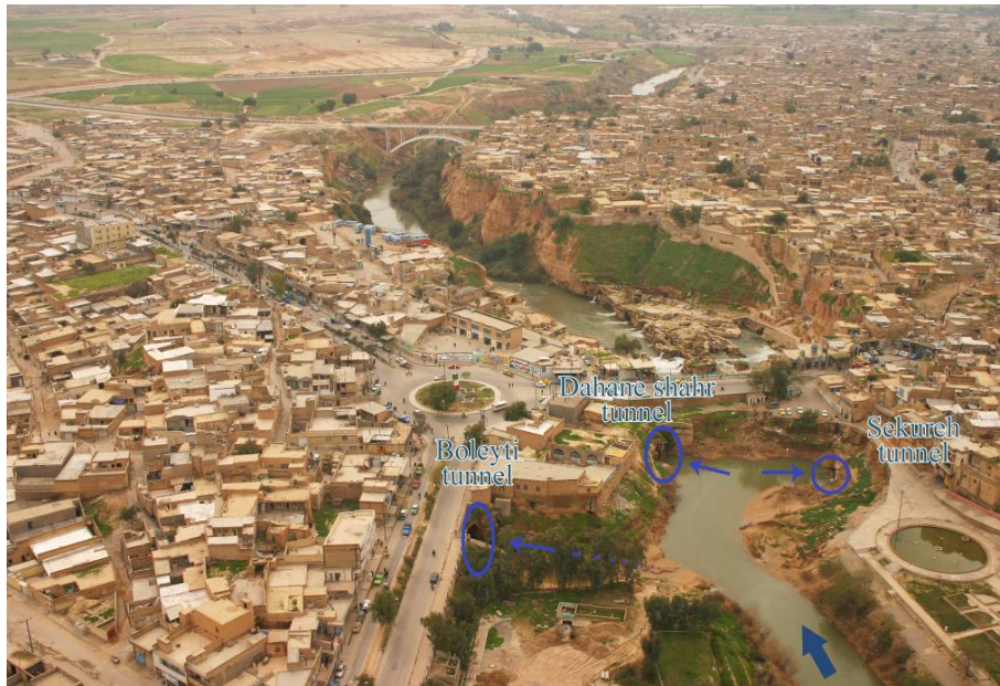
Fig24 :Aerial photo of the tunnels built inside Polband-e Gargar Bridge-dam
