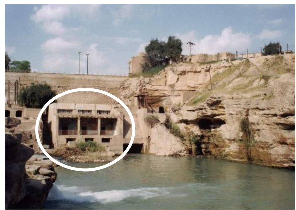
Fig. 26. Hydro power station
