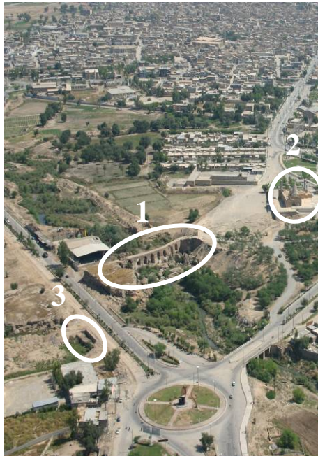
Fig. 103. Air view of 1-Lashkar bridge-Dam 2-Emamzadeh Abdollah 3- Shâhali bridge
