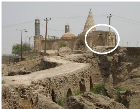
Fig. 109. View from entrance room of Lashkar bridge-Dam
