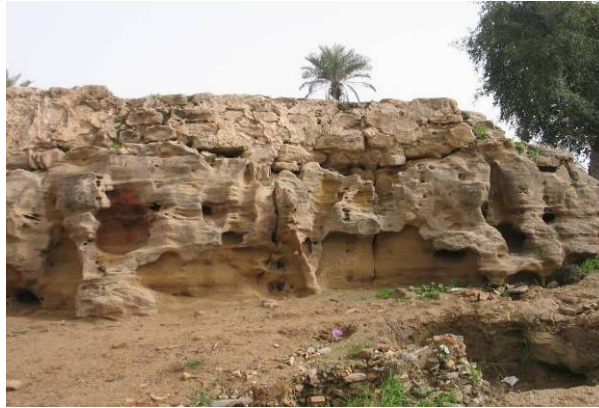
Fig. 53. A section of the Borj-e Ayâr Dam
