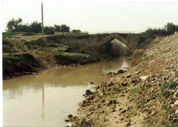
Fig. 83. the Haj-Khodai'i Bridge
