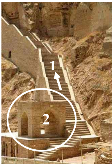
Fig. 31. 1-View of the western ramp of area 2- view of the châhâr-tâqi
