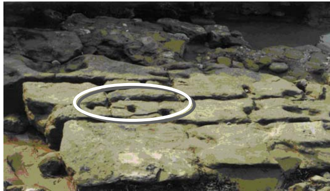
Fig. 90. Location metallic clamps in the pavement of the river bed at Polband-e Shâdorvân
