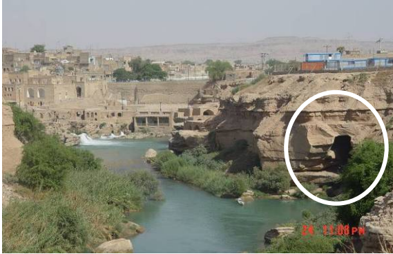
Fig. 34. One of the openings of the Boleyti tunnel
