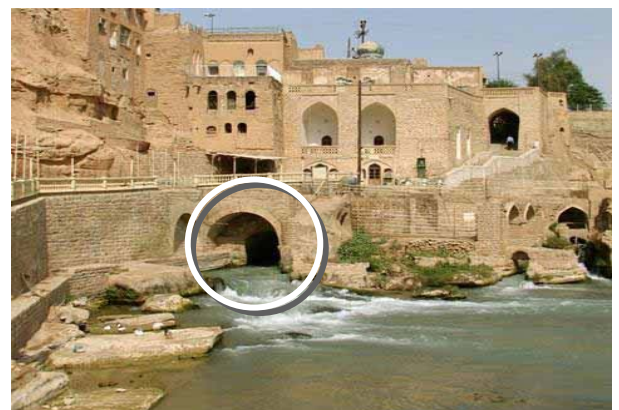
Fig. 40. Opening of the Se-Kureh tunnel in the Waterfalls area
