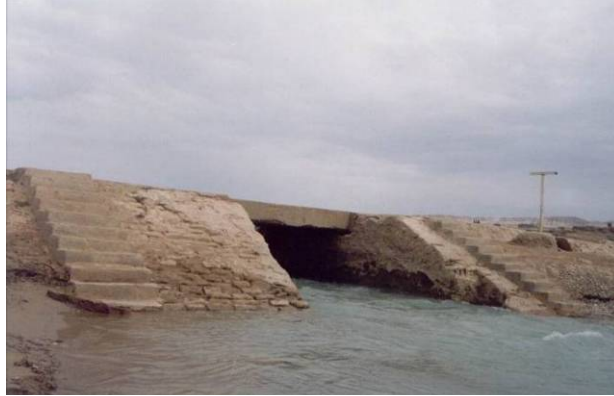
Fig. 11. View of the western outlets
