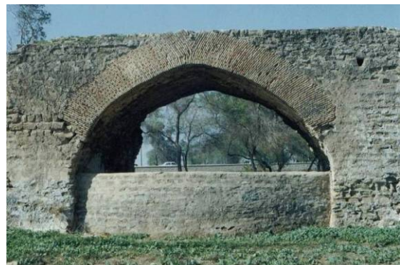
Figs. 94-95. Types of arches in the Shâdorvân bridge-Dam
