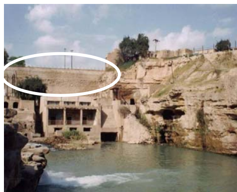
Fig. 19. Ground view of the Dam on the Gargar
