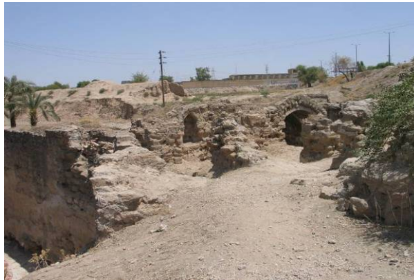
Fig. 108. View from the adjacent water watermills of Lashkar bridge-Dam
