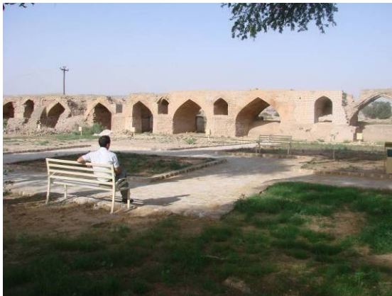
Fig. 96. A View of Shâdorvân bridge-Dam
