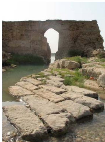
Fig. 126. Part of the riverbed stone pavement at Polband-e Shâdorvân
