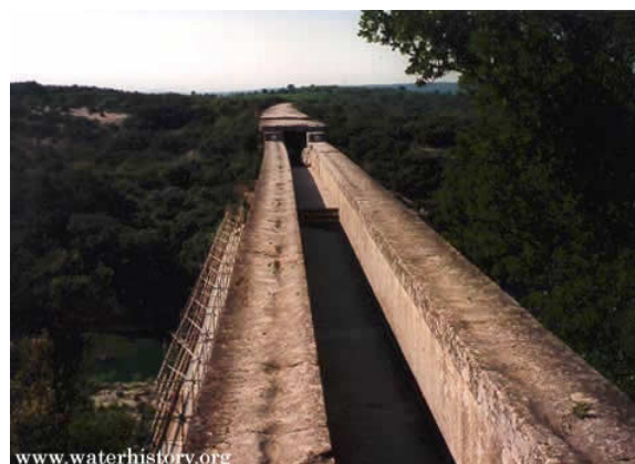
Fig. 151. Water channels of the Pont du Gard
