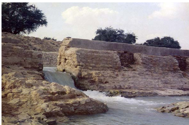
Fig. 99. the Khâk Dam in 1978
