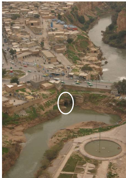
Fig. 127. View of the Shushtar tunnel built inside the Gargar Bridge-dam
