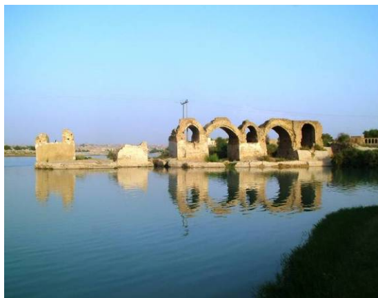
Fig. 93. View of the main and ancillary orifices in the Shâdorvân bridge
