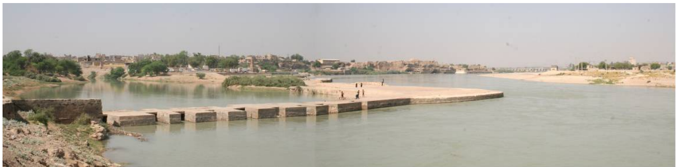
Fig. 9. View of the northern section of Band-e Mizân
