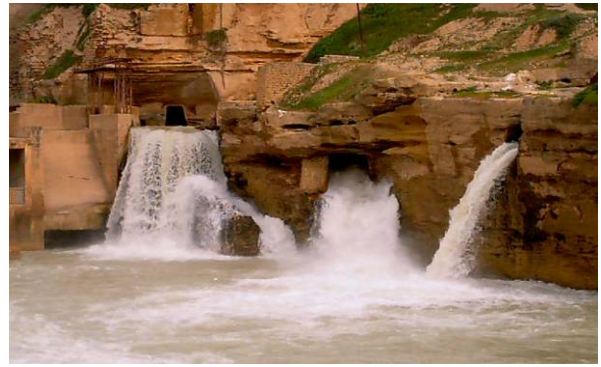
Fig. 38. Openings of Dahân-e-Shahr tunnel in the waterfalls area
