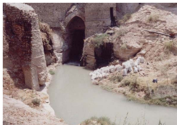
Fig. 154. View of Boleiti tunnel in Shushtar Gargar bridge-dam.
