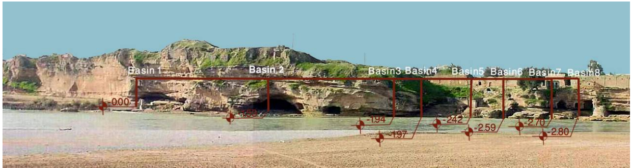
Fig. 78. The eight intakes under Salâsel castle
