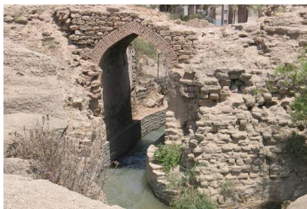
Fig. 107. View from the Lashkar bridge-Dam
