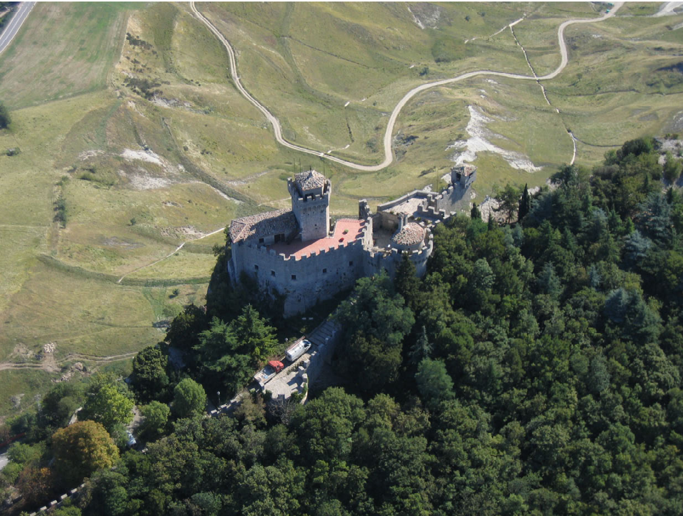
2.9. Aerial view of the Second Tower "Cesta or Fratta"
