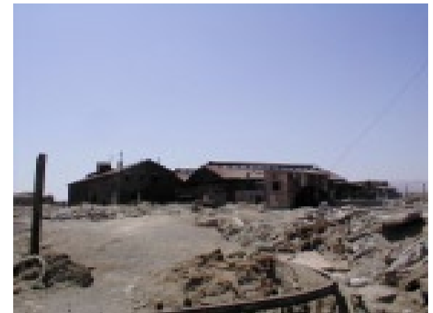
Vista general de los sectores demolidos. A la derecha la maestranza General view of the sheds. To the right is the Foundry Sergio Rowe, 1999
