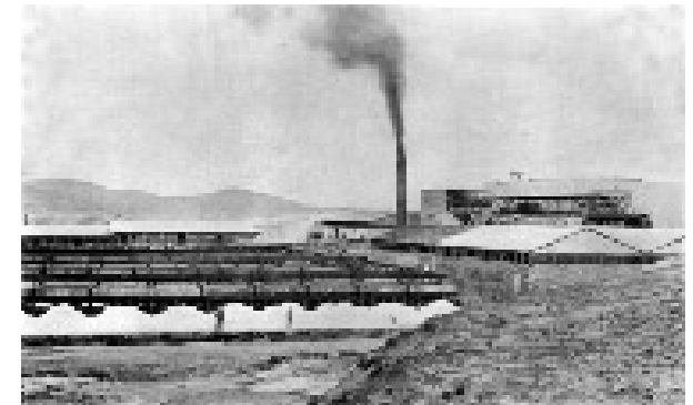
Oficina con sistema Shanks | Works featuring the Shanks system Gentileza de | By kind permission of Juan Vásquez Trigo
