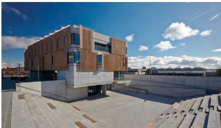
The new building for Veröld – International Centre for Multilingualism and Intercultural Understanding opened in April 2017 © The Vigdís International Centre for Multilingualism and Intercultural Understanding
