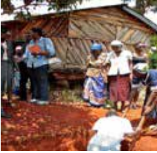
Figure 2.12: Underground tanks: Showing how they dug for constructing the tank.
