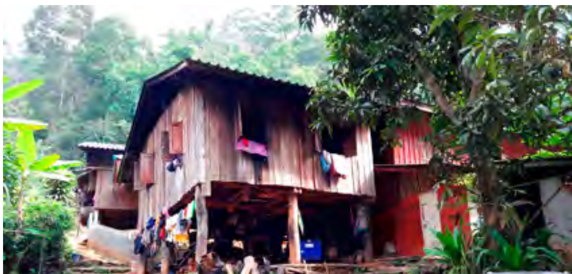
Photo 2.4 This house was rebuilt on the original settlement site of the village founder, Mr. Suka (three families are living together in the house now).
