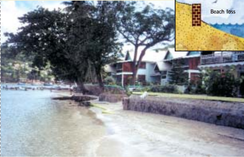
Retaining wall at Port Elizabeth, Bequia, 2000
