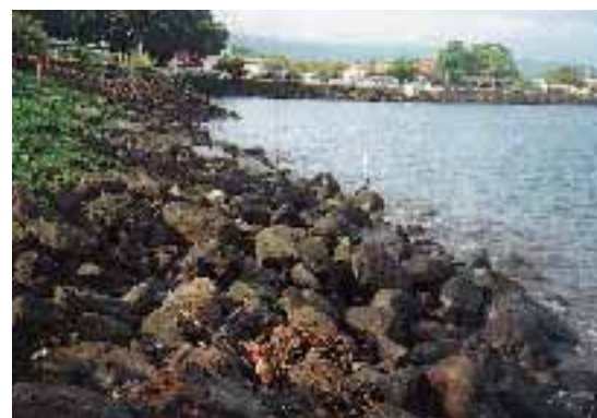
After two major cyclones in 1990 and 1991, Samoa's capital, Apia was protected with massive sea defences, December 2000.
