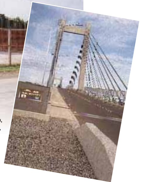
Batching plant for Palau's Compact Road, Babeldaob, and Friendship Bridge linking Koror to Babeldaob, Palau, February 2002.
