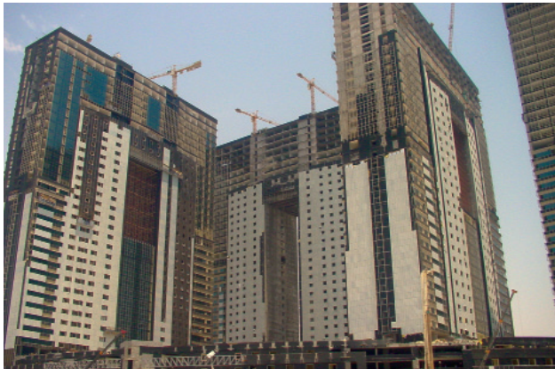
Picture: Construction site in Doha, Qatar (by H. Schwarze)
