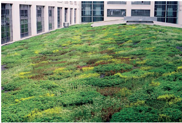
Picture: Green roof technology (by K. Barth-Scholz)
